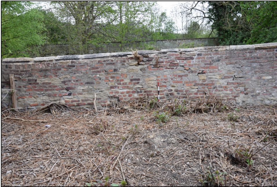
Photograph 95: Wall E, west face. This area of irregular masonry is close to the site of a small building shown in the 1816 OS map
