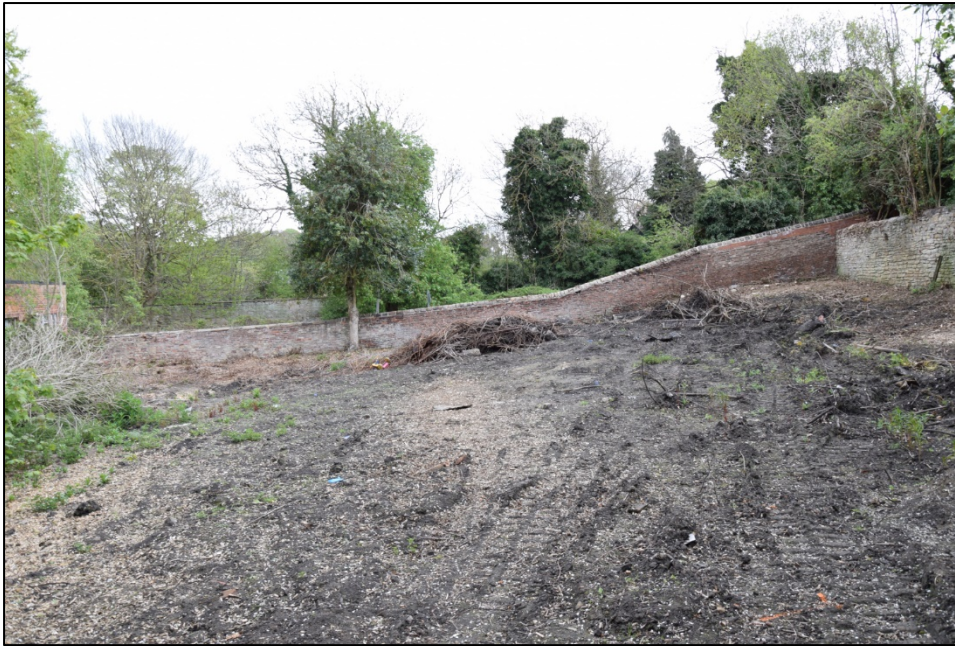
Photograph 93: Wall E, west face. This is largely brick but there are areas of rough stone in the lower section
