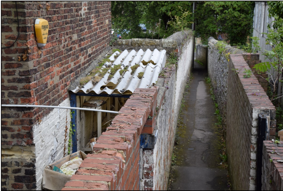
Photograph 7 (above): A view looking north along the vennel. The east end of the Cottage is about a metre west of the path. Note the distortion of the stone wall on the right side of the vennel, beyond the brick wall
