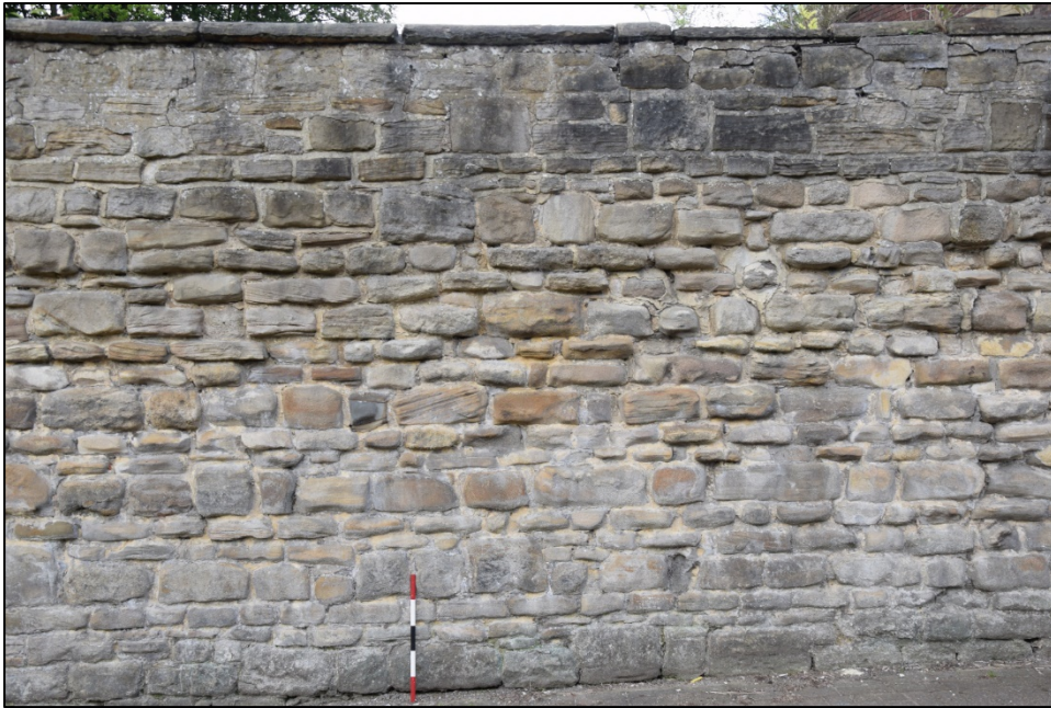
Photograph 119: Wall J, north face. Detail of the stonework
