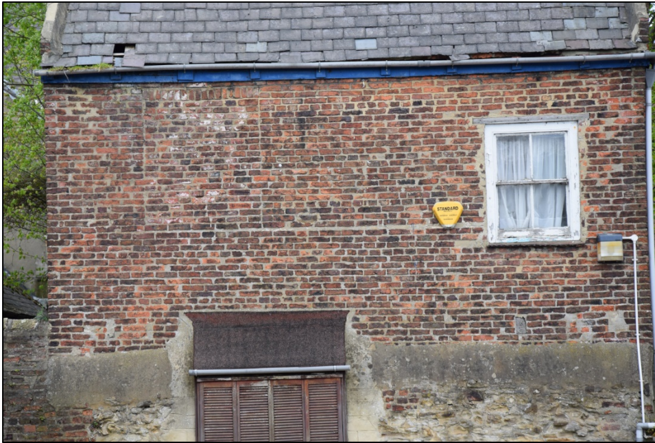
Photograph 11 (above): The first floor wall on the north side of the cottage. The blocked opening at the left does not match the existing window. Note the row of joist holes for a vanished floor just above the mortar at the bottom of the brickwork
