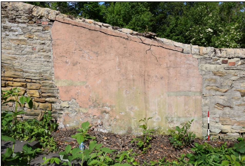
Photograph 104: Wall E, east face. The plaster marks the site of a shed shown on the 1896 OS map
