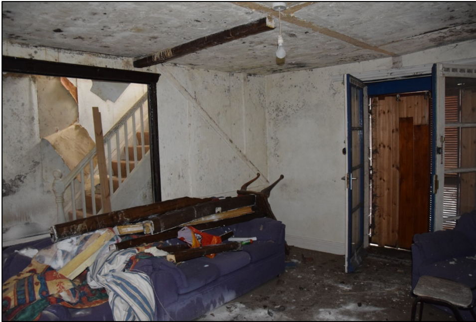
Photograph 21: The partition has a large window and 'half-timbered' features
