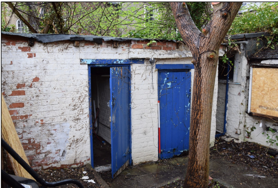
Photograph 16: A view looking south-west across the yard
