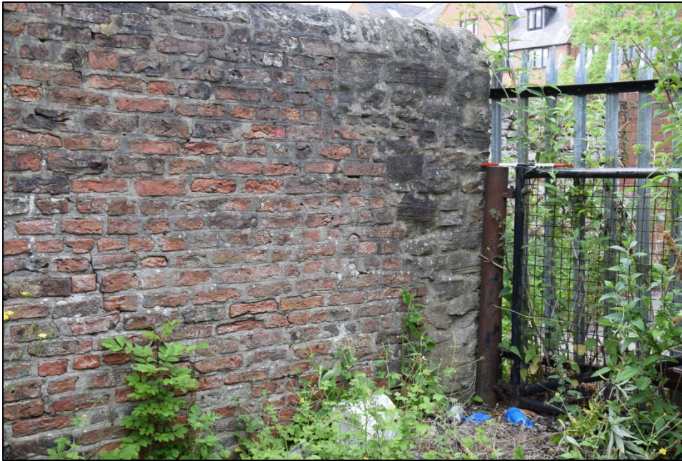
Photograph 81: Wall C, east face. This wall, like others, has brick throughout its inner face. This is the north end, rebuilt after a small building south-west of the baths was demolished
