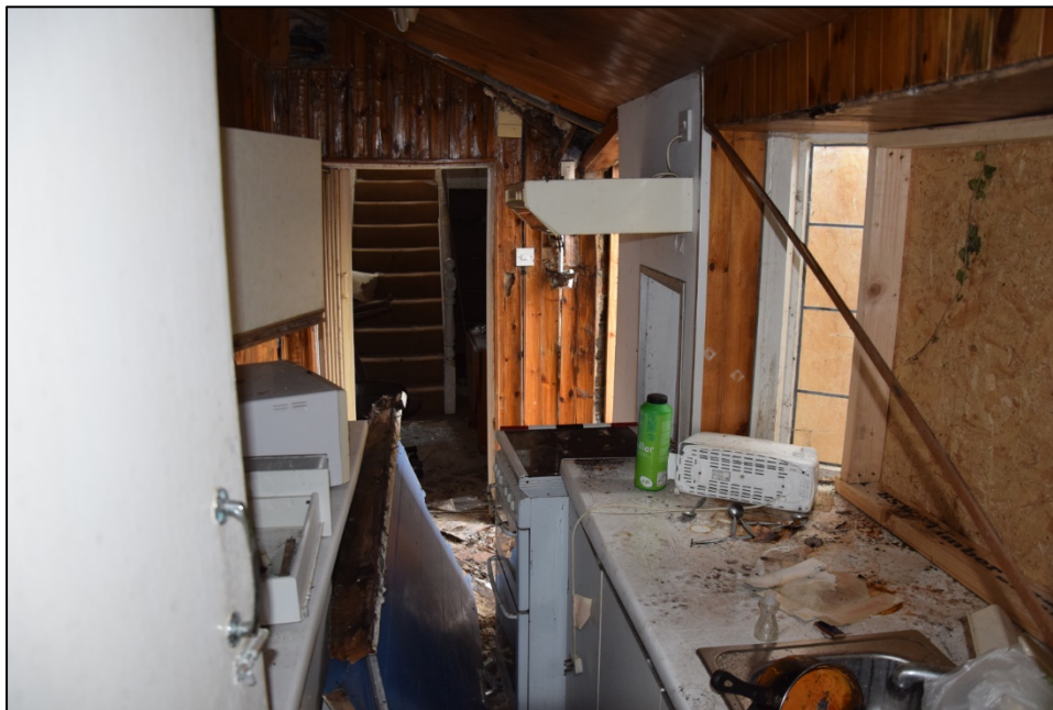
Photograph 26: The kitchen [3] and staircase [2], seen from the south
