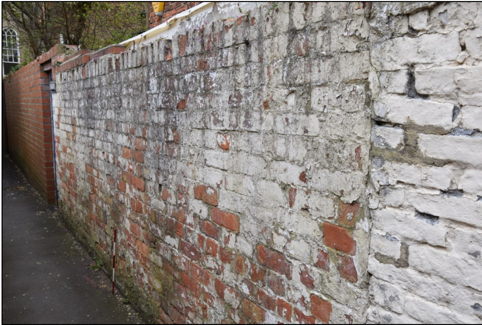
Photograph 71: Wall B, east face. The painted brick wall beside Vennel Cottage
