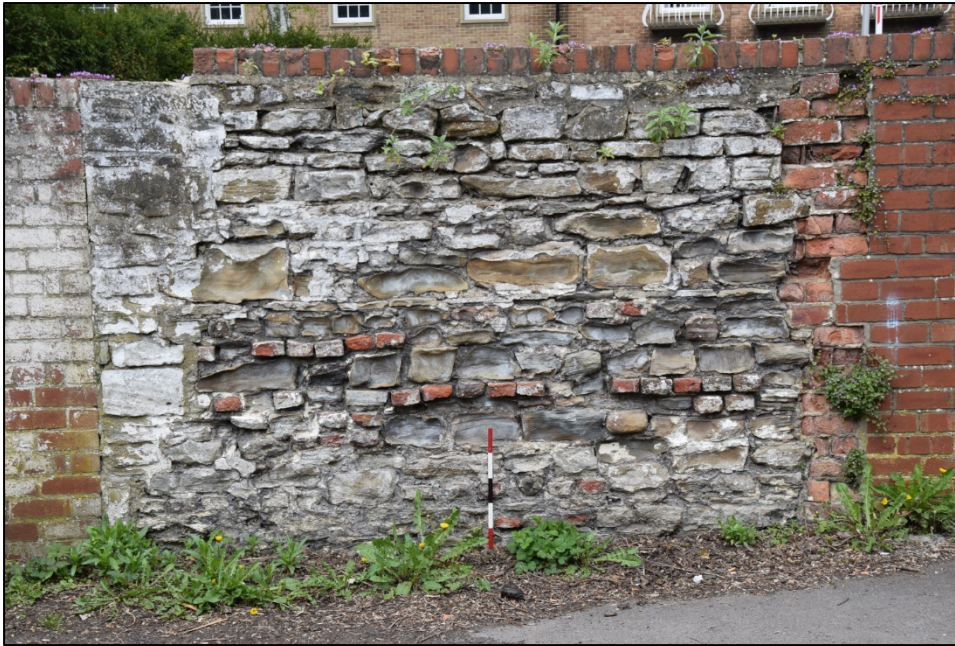
Photograph 63: Wall B, east face. Detail of the rubble masonry, with brick courses and coping and a later gate
