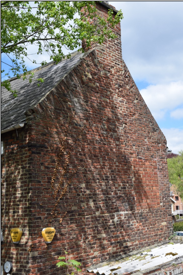
Photograph 11 (above): The first floor wall on the north side of the cottage. The blocked opening at the left does not match the existing window. Note the row of joist holes for a vanished floor just above the mortar at the bottom of the brickwork
