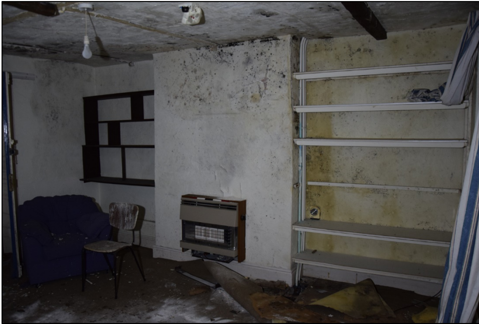
Photograph 19: The chimney breast in the east wall of the ground-floor room
