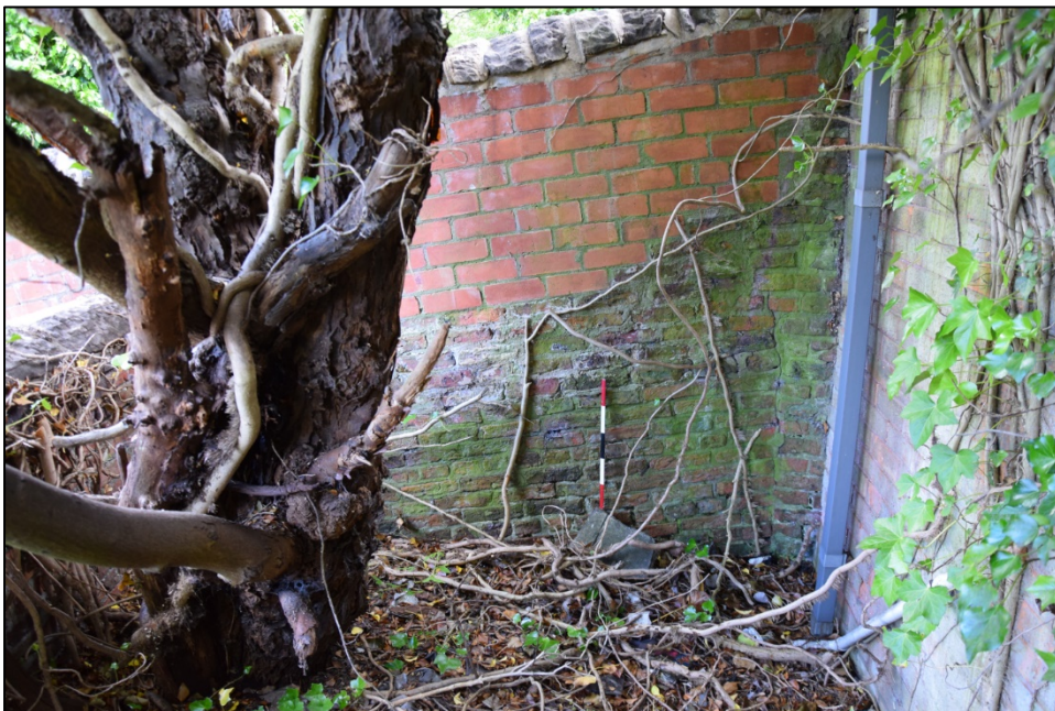
Photograph 98: Wall E, west face. The same pattern of old and modern brick between wall D and the north side of the courtyard building
