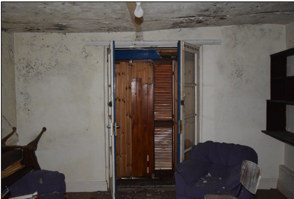
Photograph 20: Modern glazed doors in the north wall of the ground-floor room. Note the slope in the right-hand half of the ceiling here
