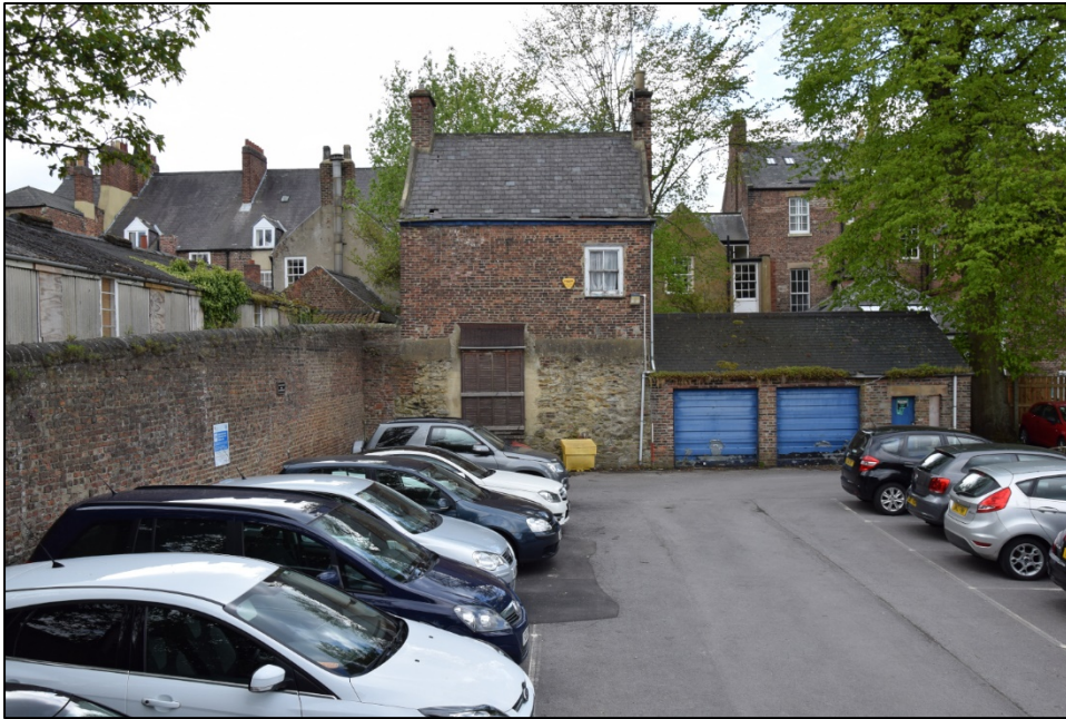
Photograph 1: Vennel Cottage and the garage block, seen from the Territorial Lane car park. The vennel runs at a higher level behind the brick wall at the left
