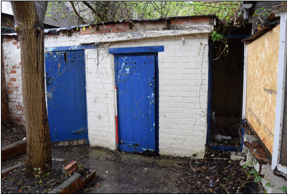
Photograph 15: The south side of the yard at Vennel Cottage. The central section was formerly a free-standing shed with a concrete slab roof. The gap at the right provides light to the bathroom window
