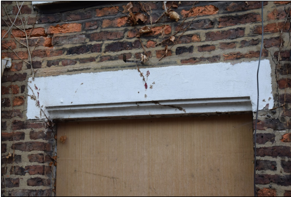
Photograph 9: Detail of one of the moulded window lintels
