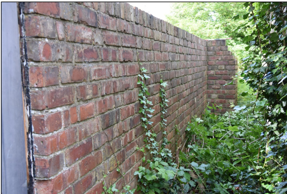
Photograph 86: Wall C, east face. Brickwork immediately north of the south gate
