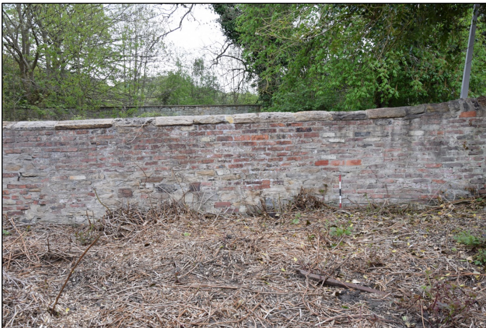
Photograph 96: Wall E, west face. Mixed sandstone and brick near the foot of the slope
