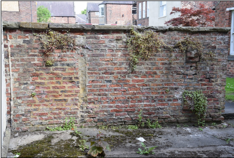
Photograph 109: Wall G, west face. Note the projecting brickwork near the south (left-hand) end
