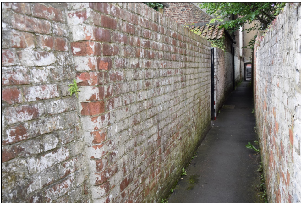
Photograph 80: Wall C, west face. The vertical brickwork is part of a small building shown on the 1919 map; the opening is the south gate
