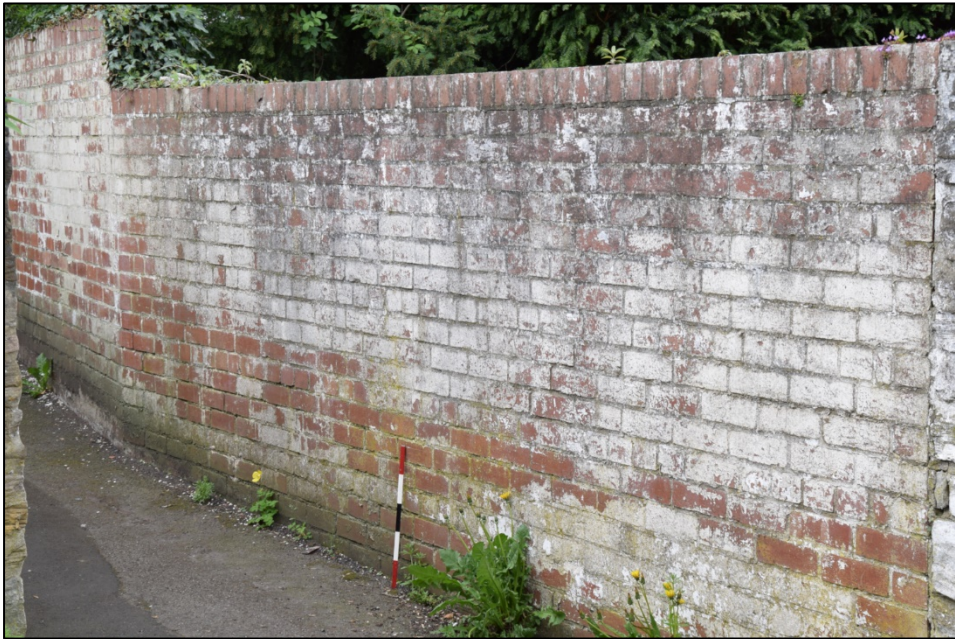
Photograph 64: Wall B, east face. Modern brickwork below and on the slope
