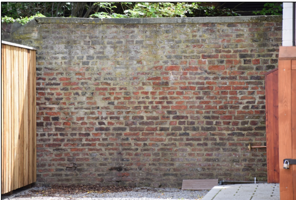
Photograph 108: Wall F, west face. Detail of the brickwork
