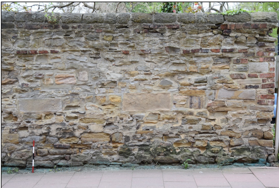
Photograph 52: Detail of the masonry in the north face of wall A; note the anomalous large dressed blocks
