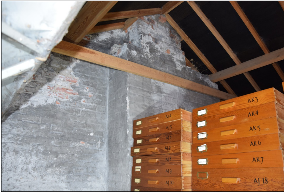
Photograph 35: The chimney on the west wall of the cottage, seen inside the east garage. The brickwork is wider low in this face, but is hidden by drawers of geological specimens
