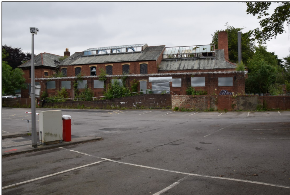
Photograph 42: The north end of the vannel, between the Territorial Lane car park and the abandoned baths building
