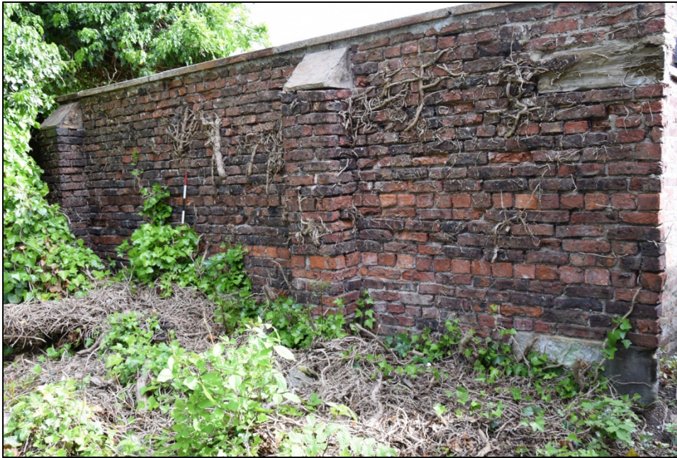
Photograph 111: Wall H, north face. These buttresses are shown on the 1816 map
