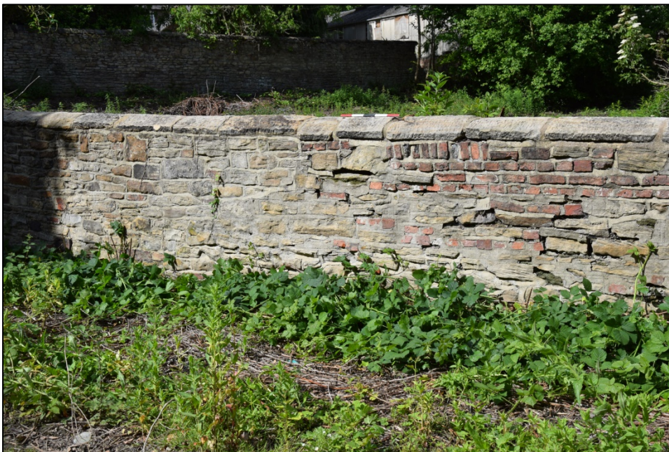
Photograph 102: Wall E, east face. This irregular masonry matches that on the west face; compare with Photo 95, above
