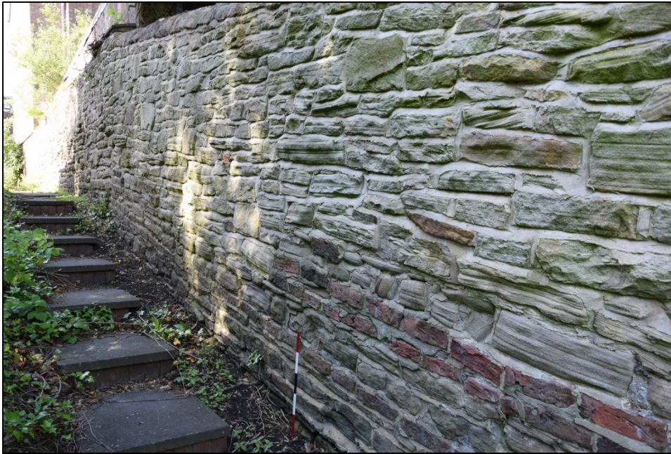
Photograph 105: Wall E, east face. The upper section of the wall has been repointed in recent years
