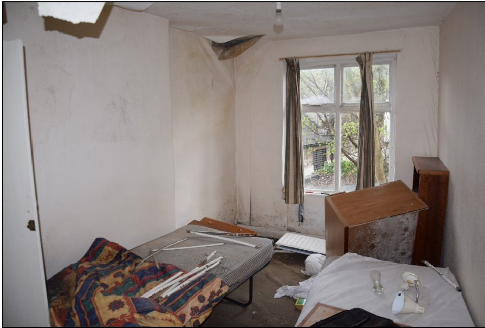
Photograph 31: The east bedroom [7], with its chimney breast. A view looking south-east
