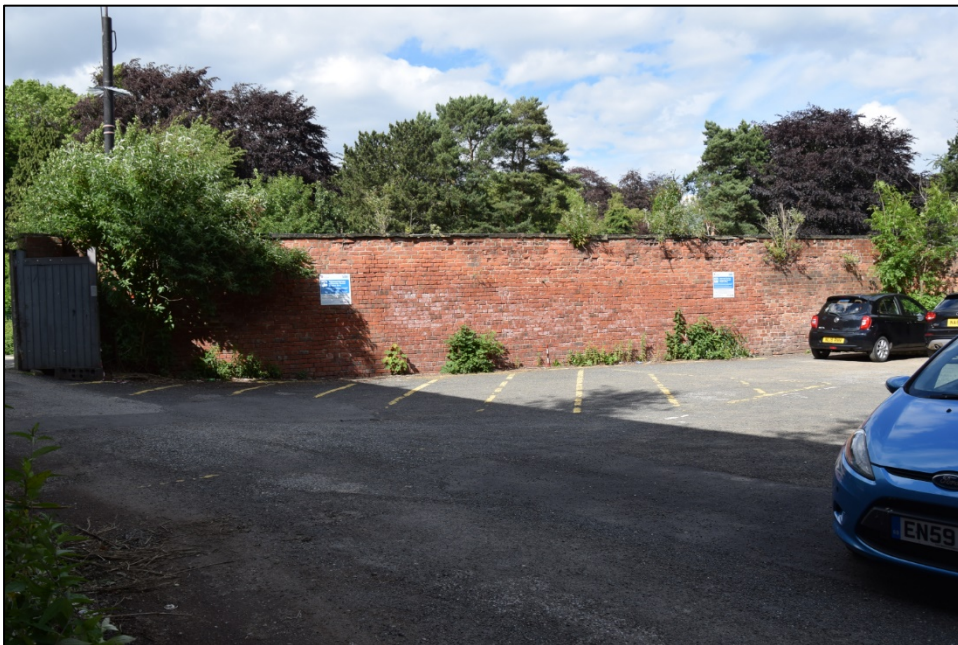
Photograph 120: Wall J, south face
