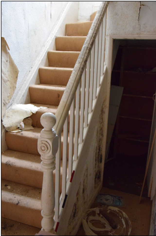
Photograph 23 (left): The staircase and the under-stair cupboard
