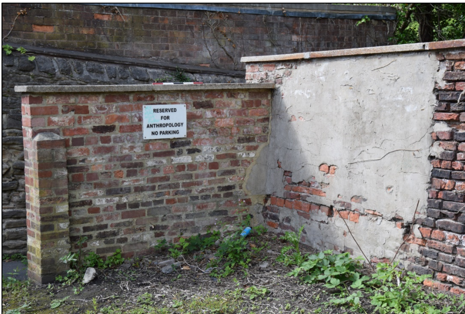
Photograph 114: Wall H, south face. A modern wall runs south beside an area of render. There was a summer house in this corner in 1816
