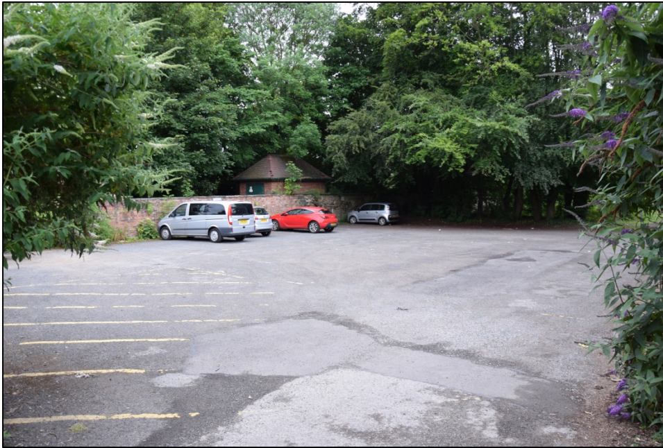
Photograph 49: Wall K, on the east side of the car park, extends beyond the substation building into the wooded area to the south
