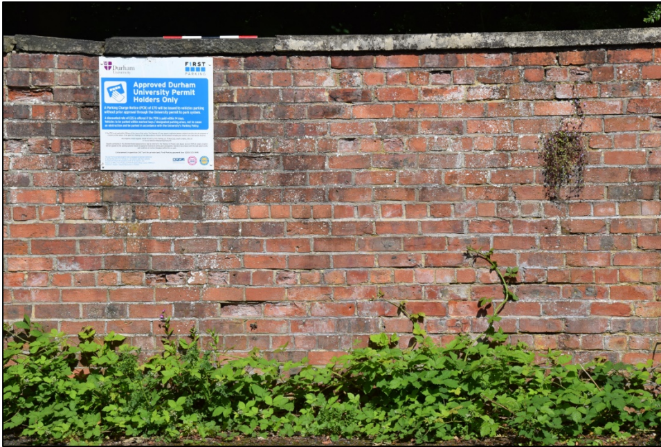
Photograph 123: Wall K, west face. Detail of the masonry
