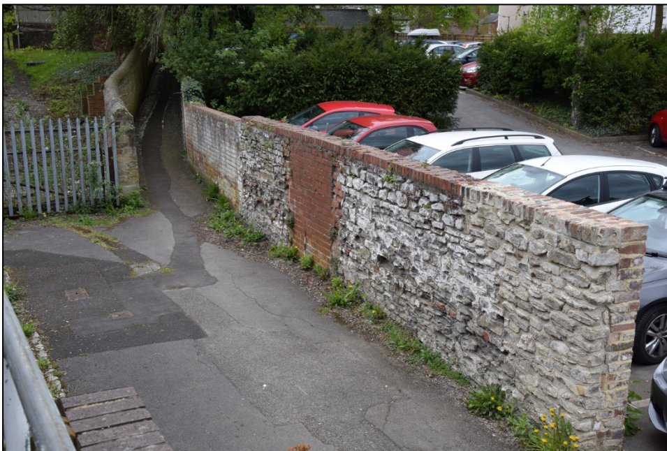
Photograph 62: Wall B, east face. This short section of the old garden wall has an outer face of roughly-coursed stone
