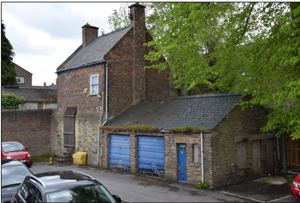
Photograph 2: Vennel Cottage seen from the north-west. Note the thick stone of the lower wall of the house
