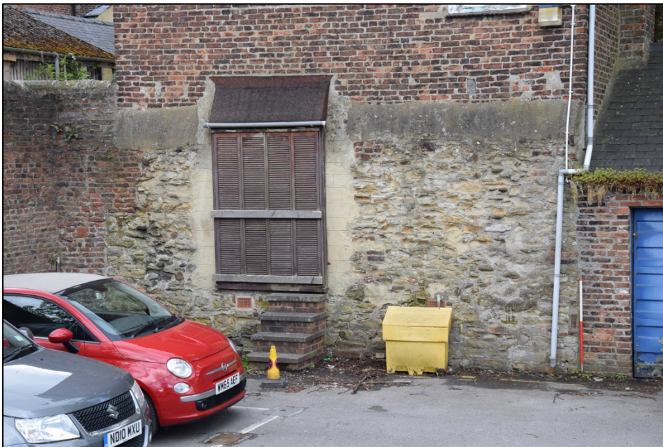
Photograph 10: The thick stone wall in the north face of Vennel Cottage does not extend as far as the wall of the vennel itself, and it does not run into the adjoining garage building at the right. A slope of cement mortar provides a crude cover for the join between the thick stone wall and the thinner brickwork above
