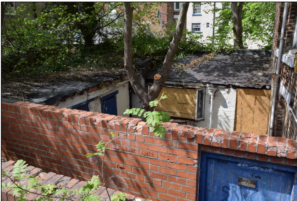
Photograph 6: The yard south of Vennel Cottage
