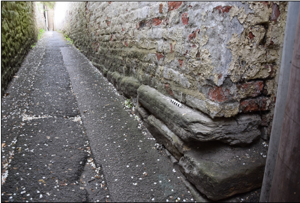
Photograph 67: Wall B, east face. This stone foundation is visible for about 13m from the north-east corner of the old building
