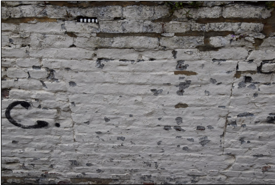
Photograph 69: Wall B, east face. Detail of the blocked opening shown above
