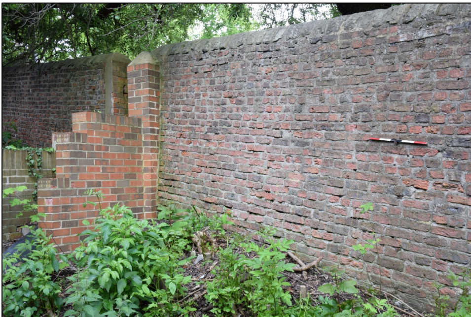
Photograph 82: Wall C, east face. The modern nursery gate and steps
