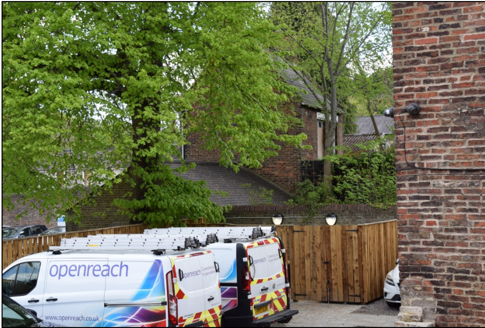
Photograph 37: A view of Vennel Cottage and the garages from the south end of Territorial Lane. The garden inside the boundary wall is about 1.4m above the ground level seen here
