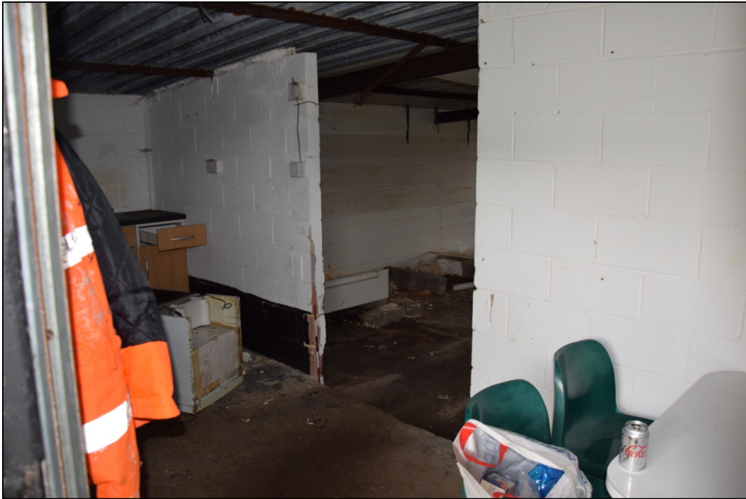
Photograph 15: Mess room at the south end of the detached kennel
