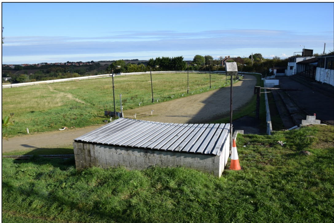
Photograph 4: The track seen from the south, with the open shed in the foreground
