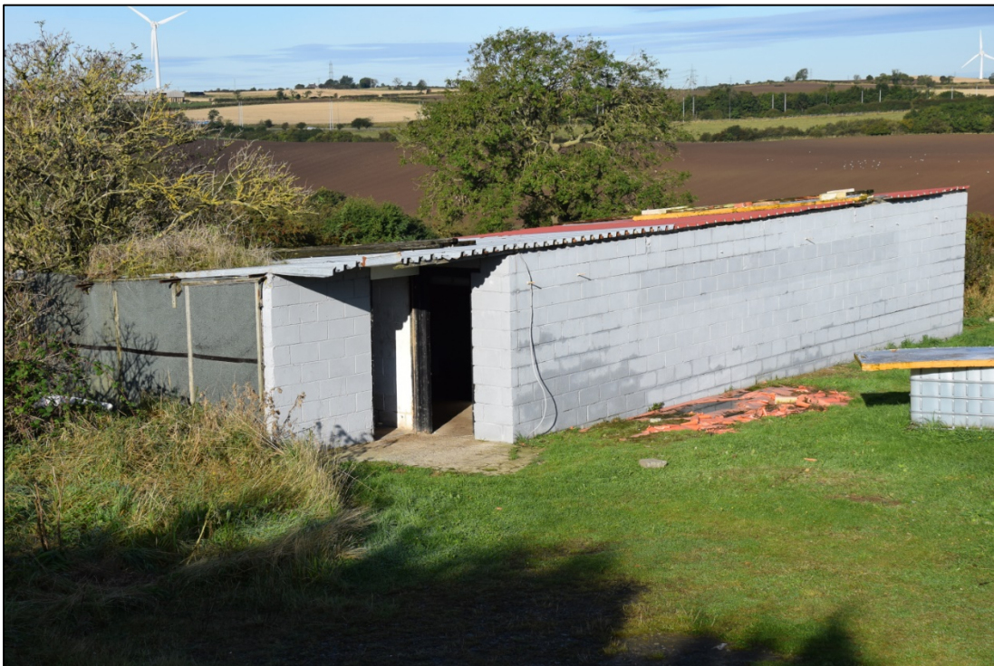
Photograph 14: The detached kennel building at the south-west side of the site
