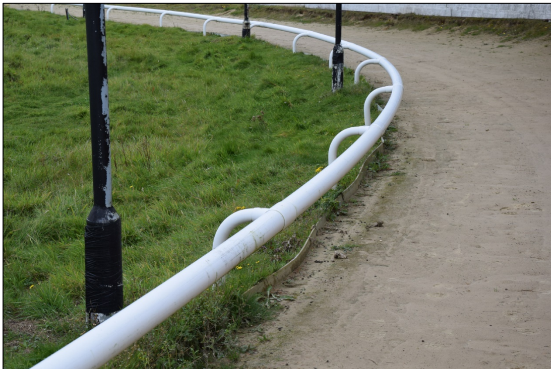
Photograph 6: Plastic tube fencing on the inside of the north-east bend
