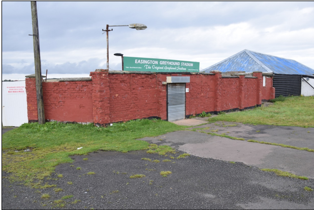
Photograph 61: The original pedestrian entrance
