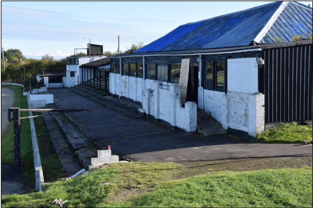
Photograph 19: The buildings and the open and covered terraces, seen from the south
