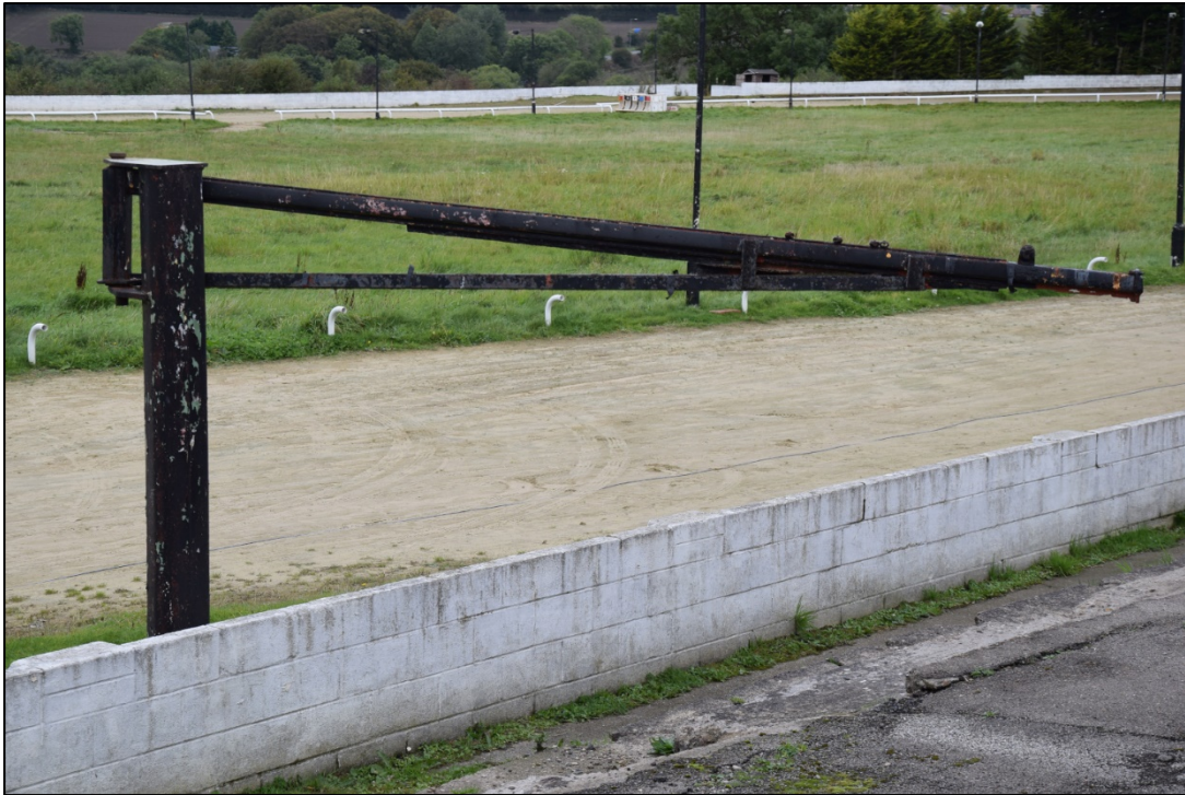
Photograph 17: The hinged gantry for indicator lights, near the starting traps
