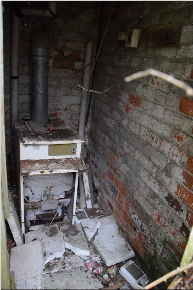
Photograph 59 (left): Boiler house [29]
