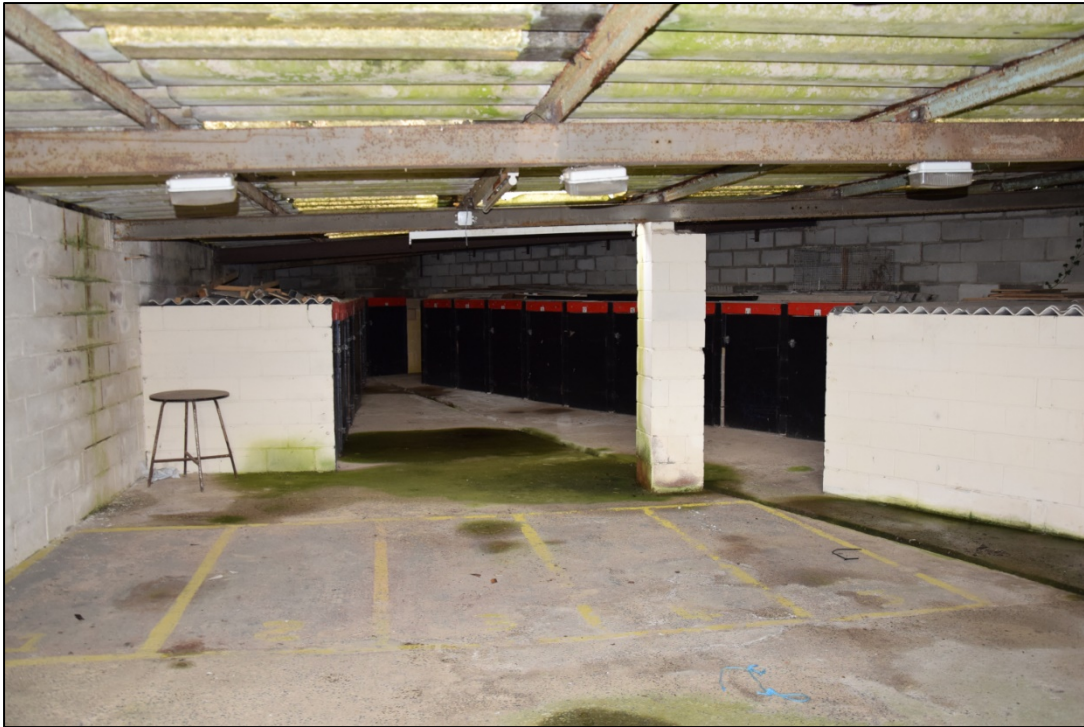
Photograph 51: A view looking north into the kennel block [23]
