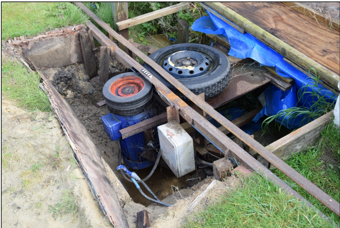
Photograph 12: The electric motor, drive wheels and the blue cable
