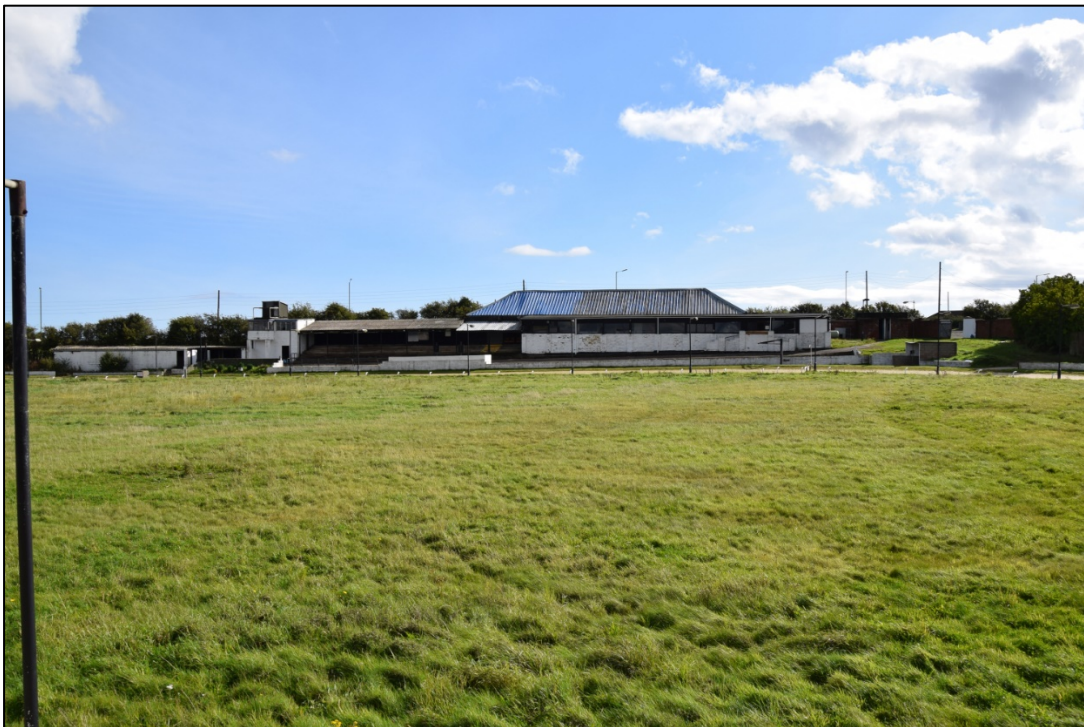
Photograph 18: A view of the stadium buildings from the west side of the track. The hipped blue roof at the centre covers the oldest part of the structure
