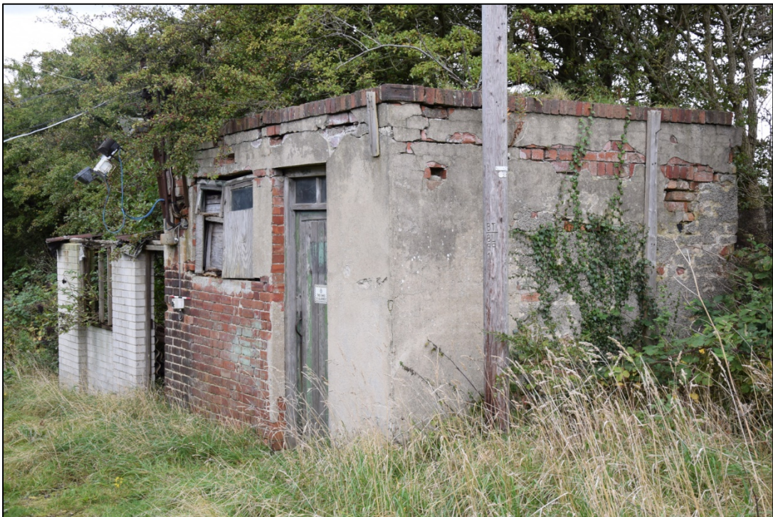
Photograph 58: The old sub-station and its later shed, seen from the south
