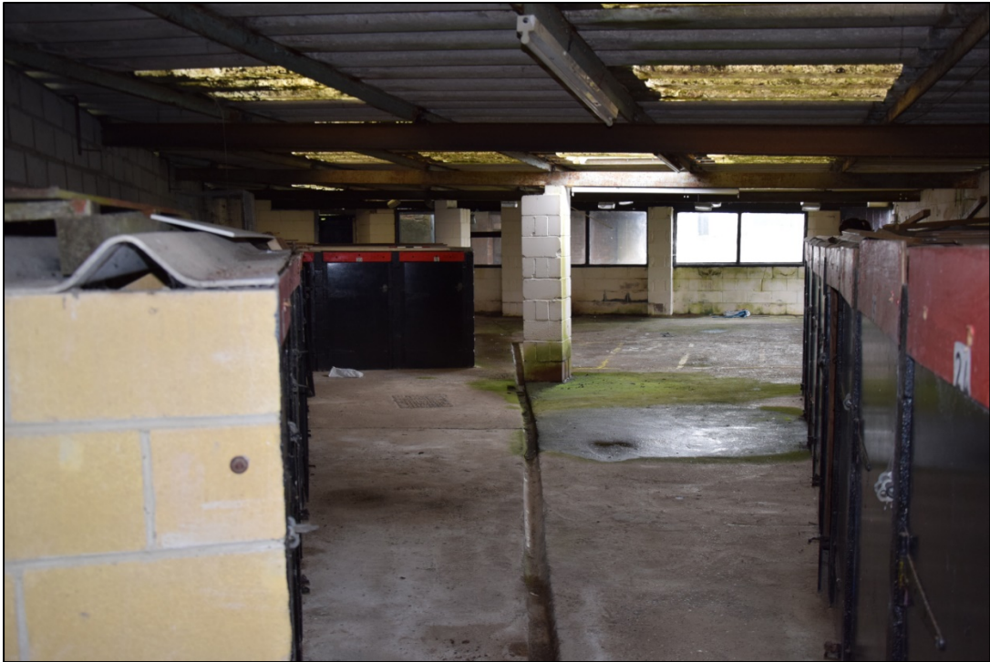
Photograph 53: The view from the north end of the kennel block [23]
