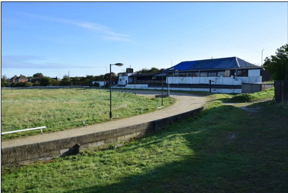
Photograph 2: The stadium buildings and the east side of the track, showing the slope
