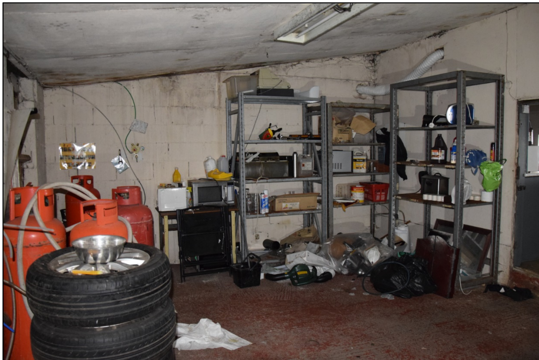
Photograph 34: Interior of the bar cellar [9]
