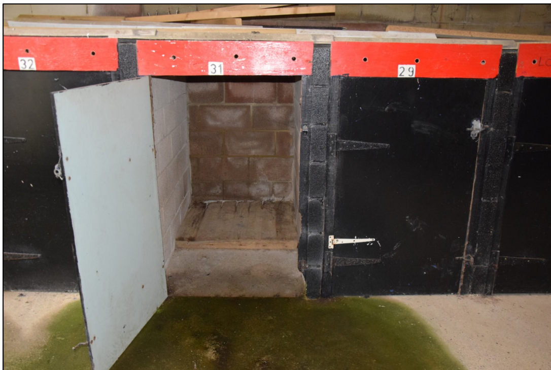
Photograph 52: A typical kennel of bare concrete and timber. It is covered with corrugated sheets
