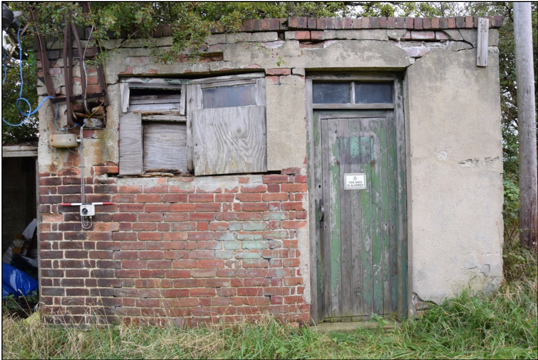
Photograph 57: The front of the old electrical sub-station behind the stadium buildings
