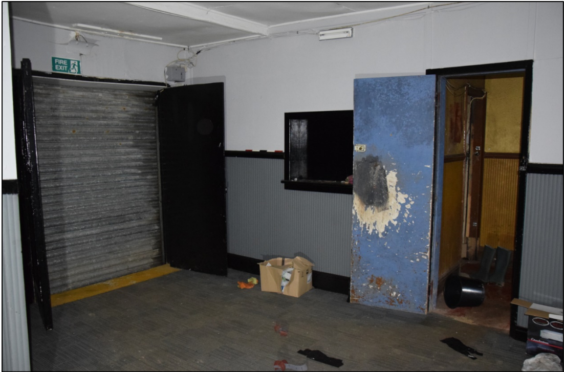
Photograph 37: Lobby 12, showing the shuttered terrace entrance and the door to the small lobby [13]
