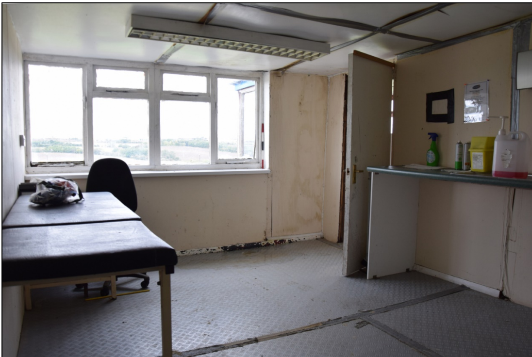
Photograph 42: The vet's room [19] at first-floor level
