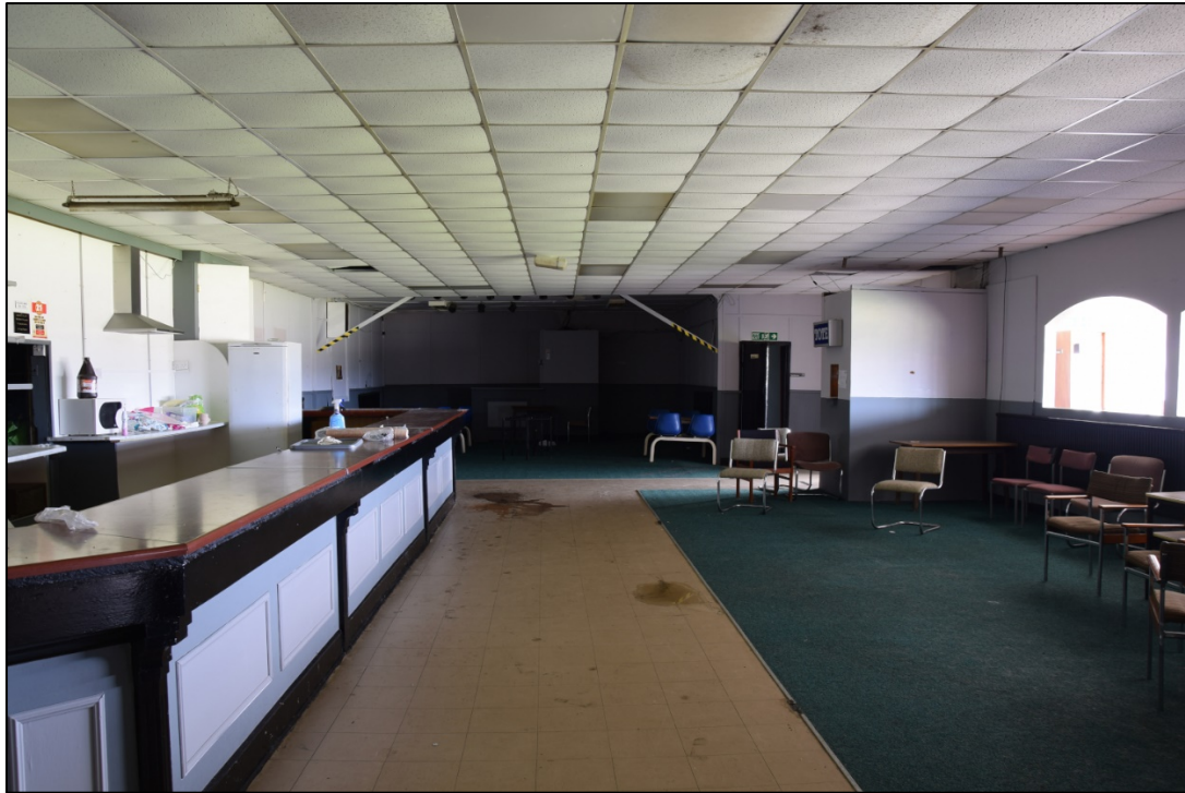
Photograph 31: A view looking south in the bar, with doors to the toilets [6, 7] at the far end
