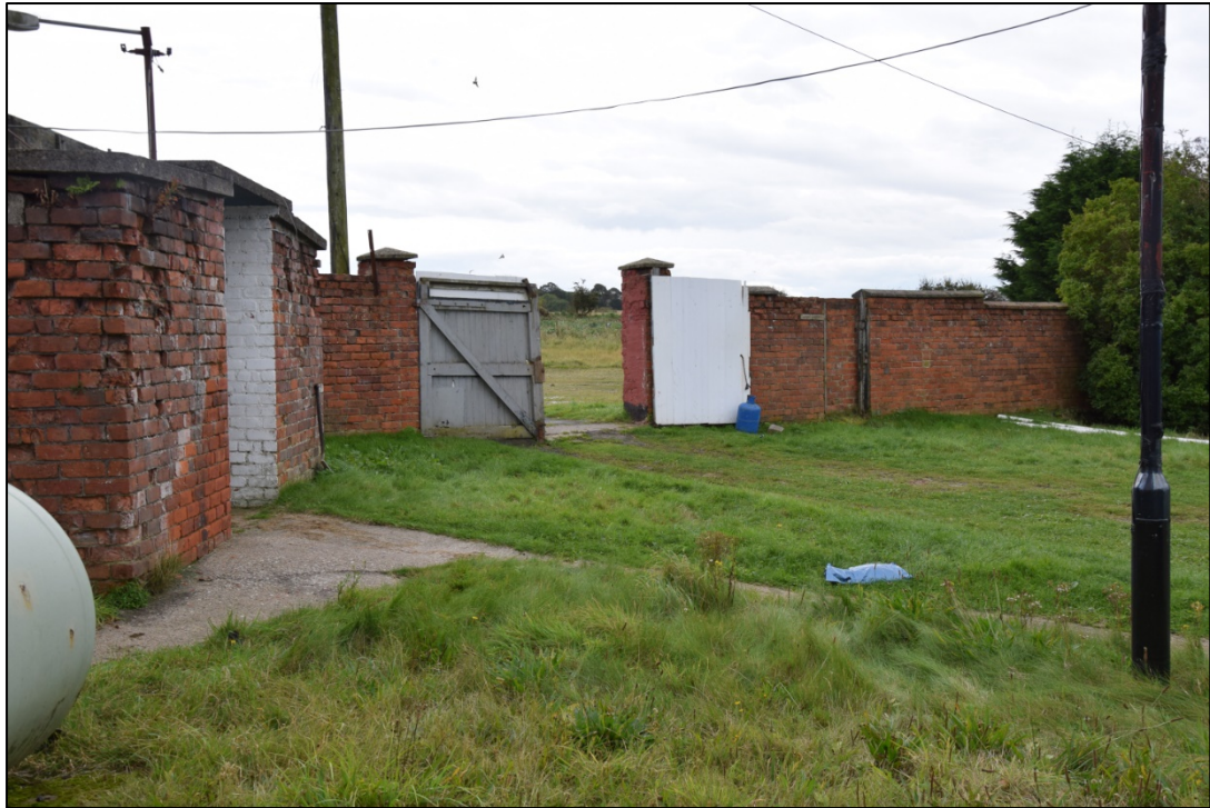
Photograph 65: The turnstile blocks [31, 32] and the main vehicle entrance [33], seen from the north
