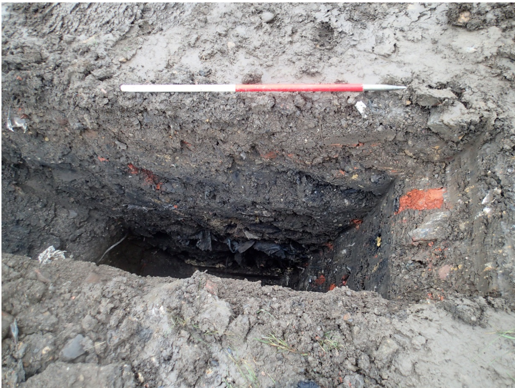
Photograph 8: Test pit 22, looking north. Note plastic at depth in made ground
