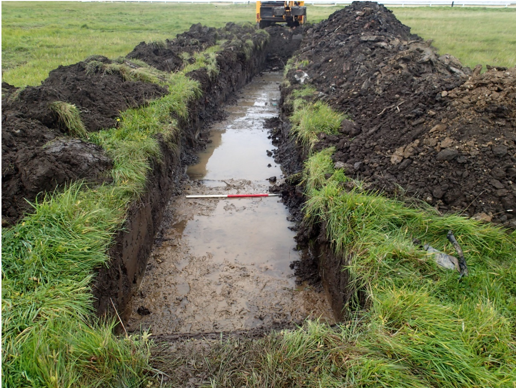
Photograph 7: Trench 20, looking west and showing increasing depth of made ground
