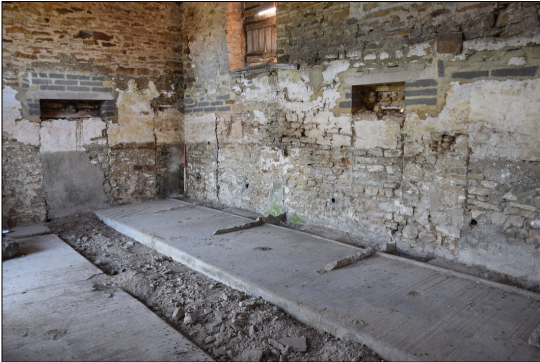
Photograph 15: Inside building 1 are the remains of 20th-century cow stalls and a large floor drain. Recent repairs to the door and window lintels can be seen. A view looking south-east
