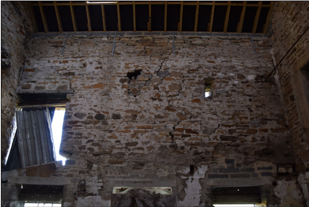
Photograph 25 (above): Settlement cracks can be seen in the north wall of the hay loft at the west end of building 1
