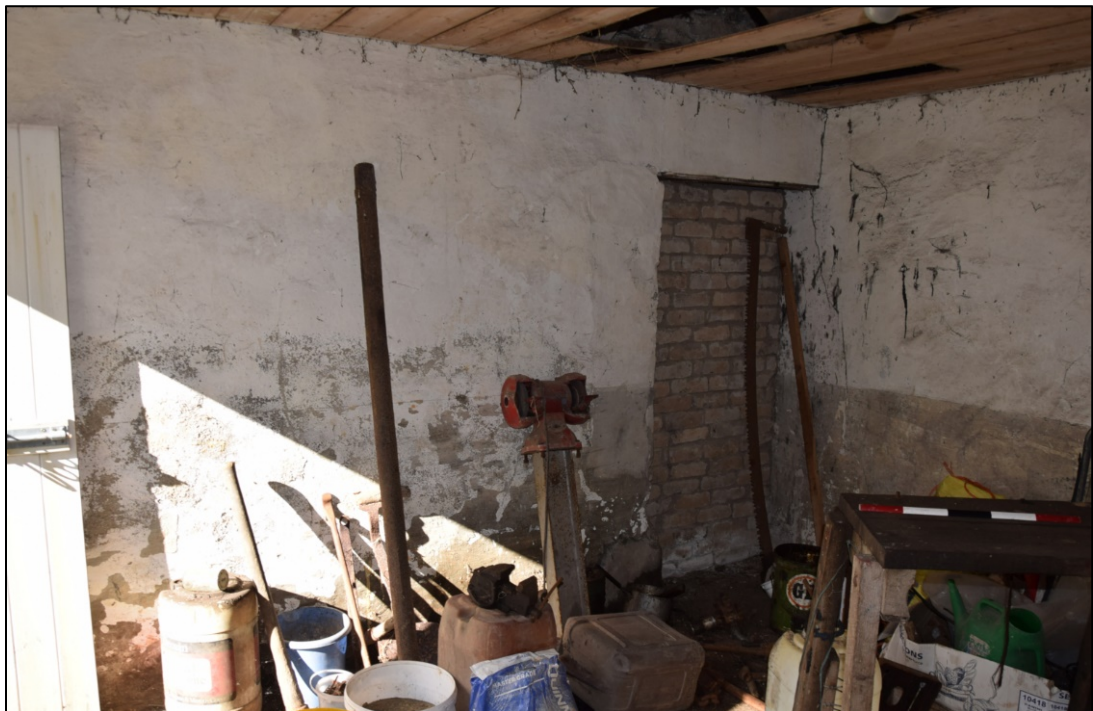
Photograph 68: A view looking north-west in the east room, with the blocked internal door
