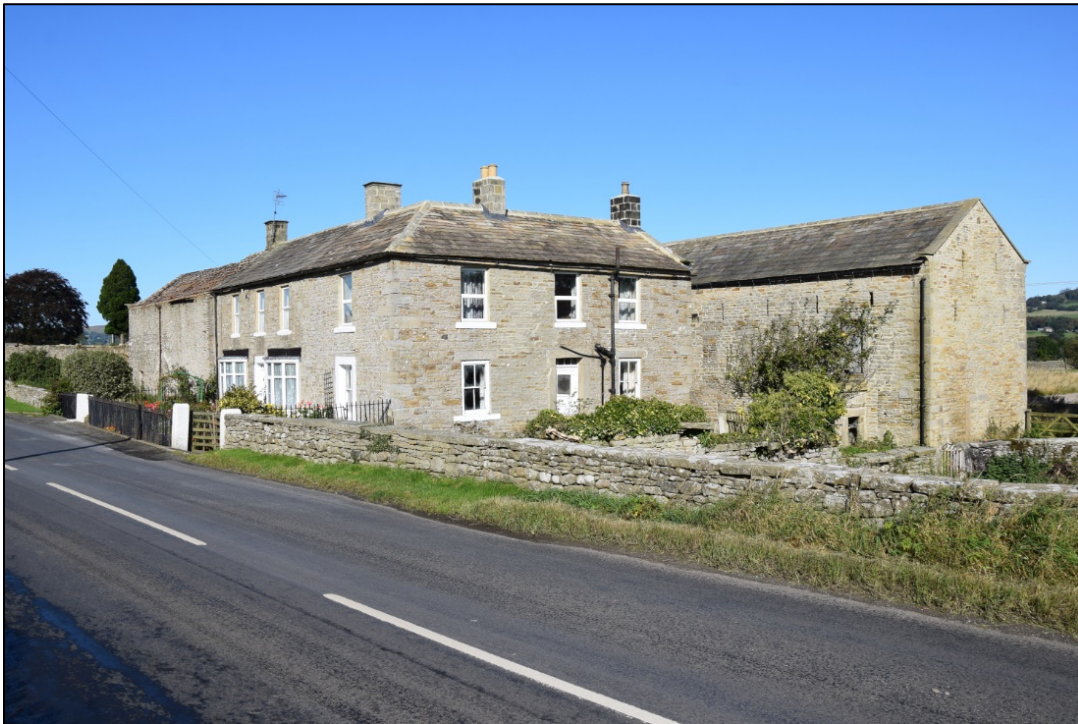
Photograph 2: The L-shaped houses at the east side of the site. Building 1 is at the right and building 2 continues the range at the left
