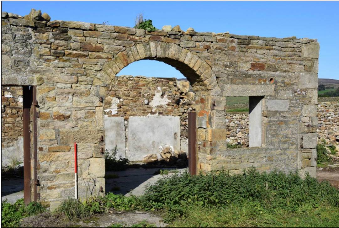
Photograph 49: The arched opening, superficially similar to a hemmel door, is a later addition to the building
