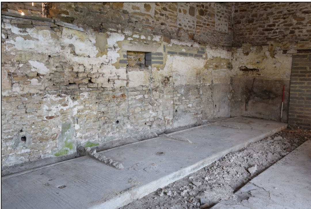
Photograph 16: A view looking south-west in the old part of the building. Older masonry fills the first-floor windows, above the recent repairs
