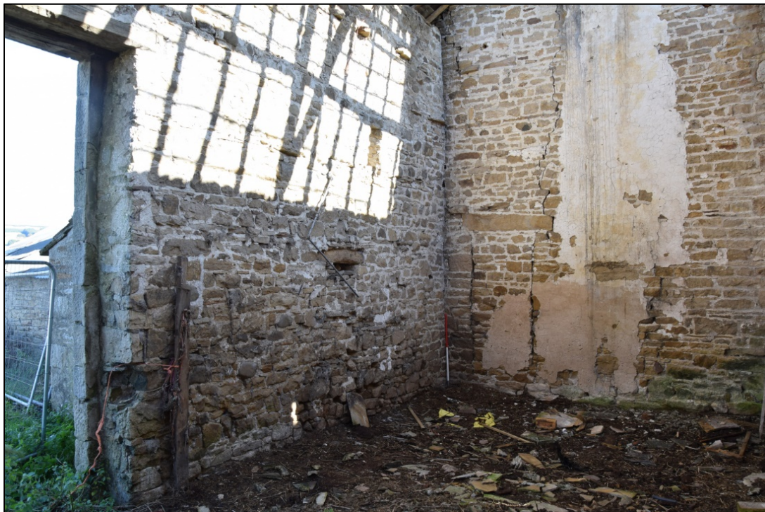
Photograph 44 (below): The east end of the north wall, with a small blocked window that is now covered by a lean- to shed outside
