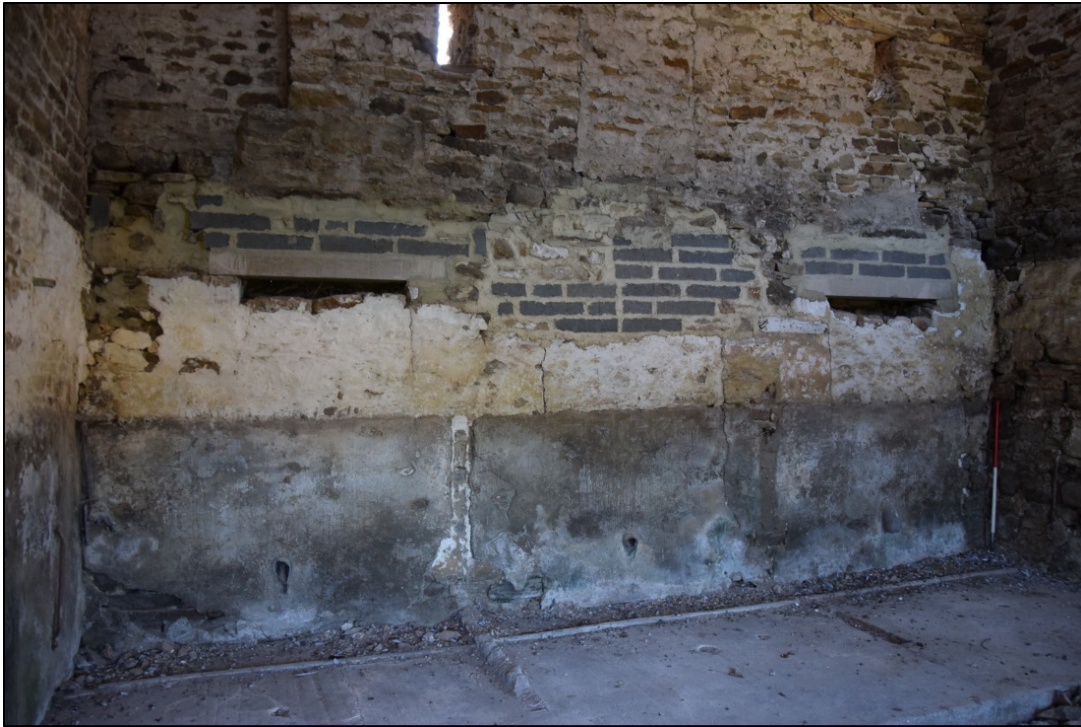
Photograph 21: The south wall of the byre in the west extension. The arrangement of stalls, the wall finishes and the recent repairs are the same as those seen elsewhere in building 1
