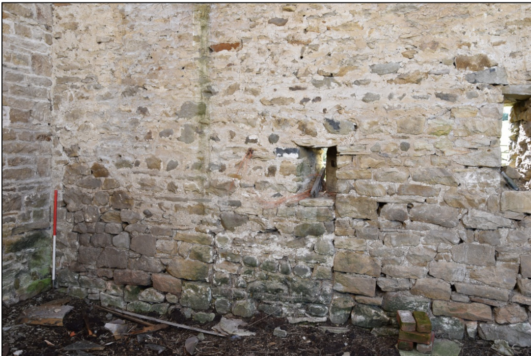
Photograph 42: The truncated blocked door at the south-east corner. The jamb can be seen in the low breather slit. Older masonry survives low down, beside the scale
