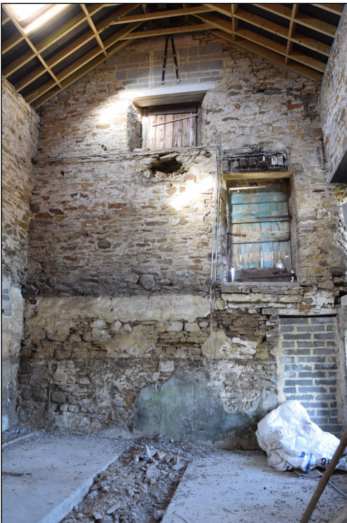
Photograph 25 (above): Settlement cracks can be seen in the north wall of the hay loft at the west end of building 1
