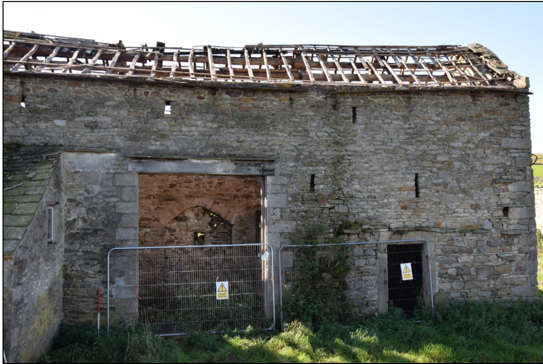
Photograph 29 (above): Detail of the north wall showing the change in the quoins at the right
