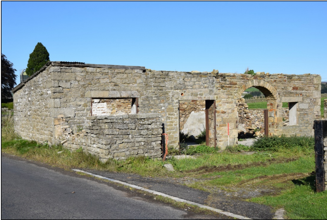
Photograph 47: Building 4 seen from the south-east
