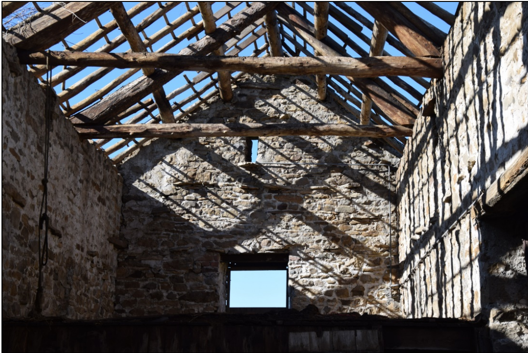
Photograph 37: The hay loft at the west end. There are more through stones here than on the outside faces of the walls. Note the crude roundwood timber of the replacement roof
