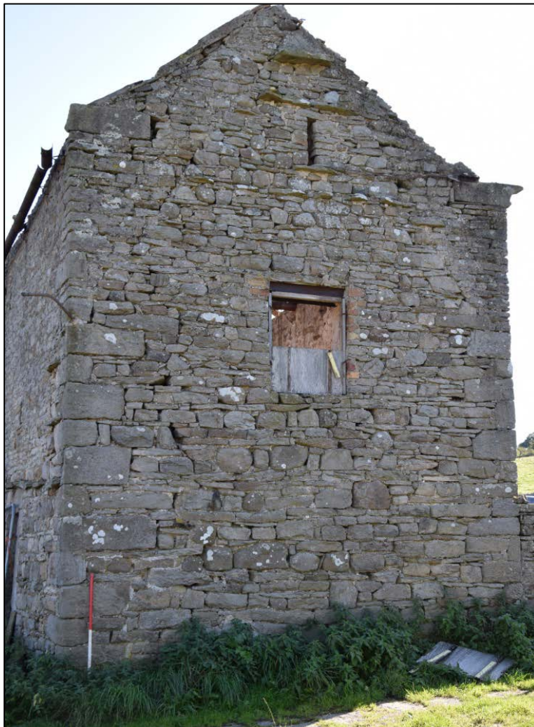
Photograph 29 (above): Detail of the north wall showing the change in the quoins at the right
