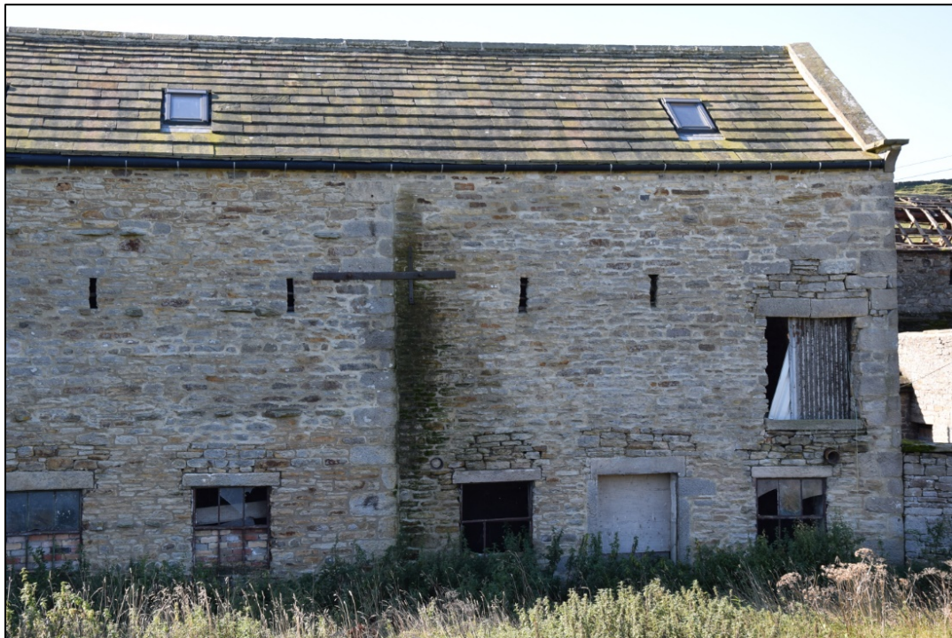
Photograph 12: The north face of the extension, with the reinforcing iron band across the junction
