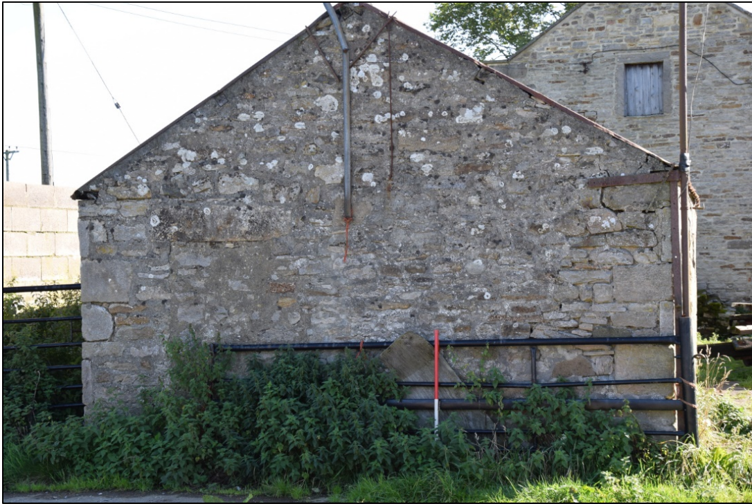
Photograph 65: The west end of the shed. A blocked door is faintly visible near the right-hand end
