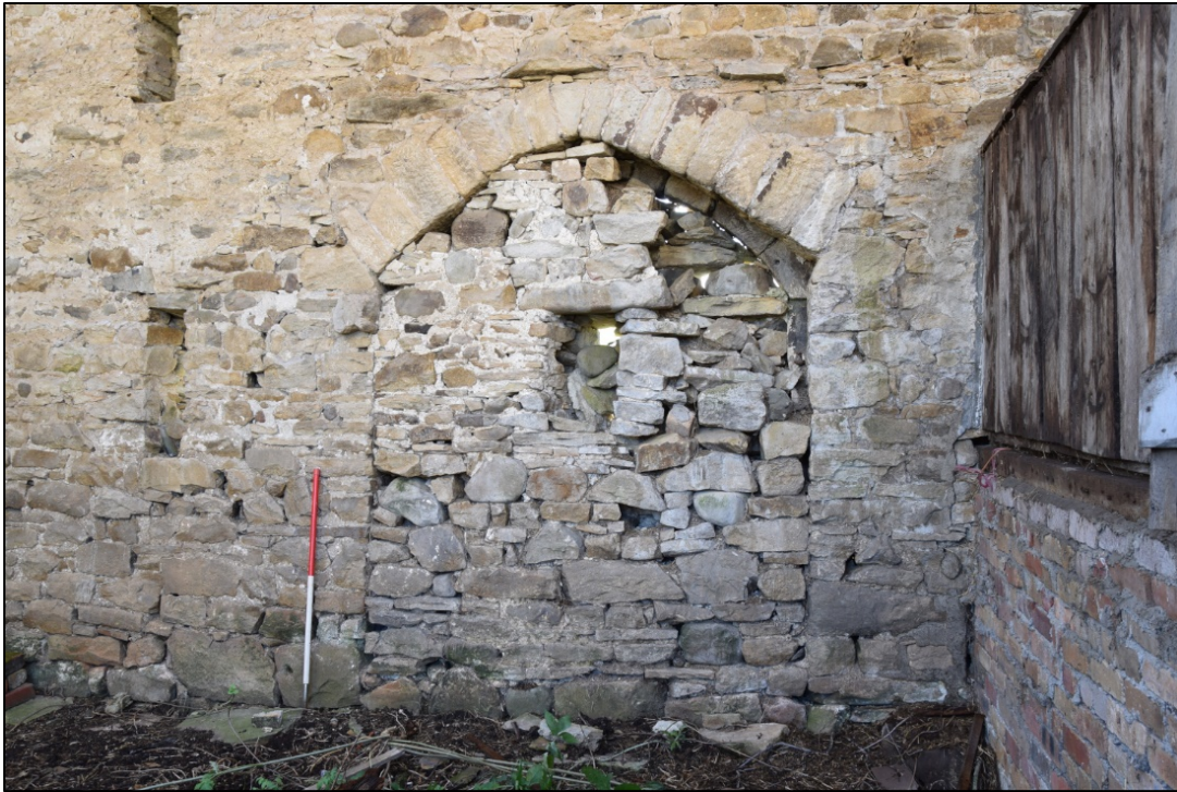
Photograph 41: Detail of the central door, showing the rebate and hinge pin
