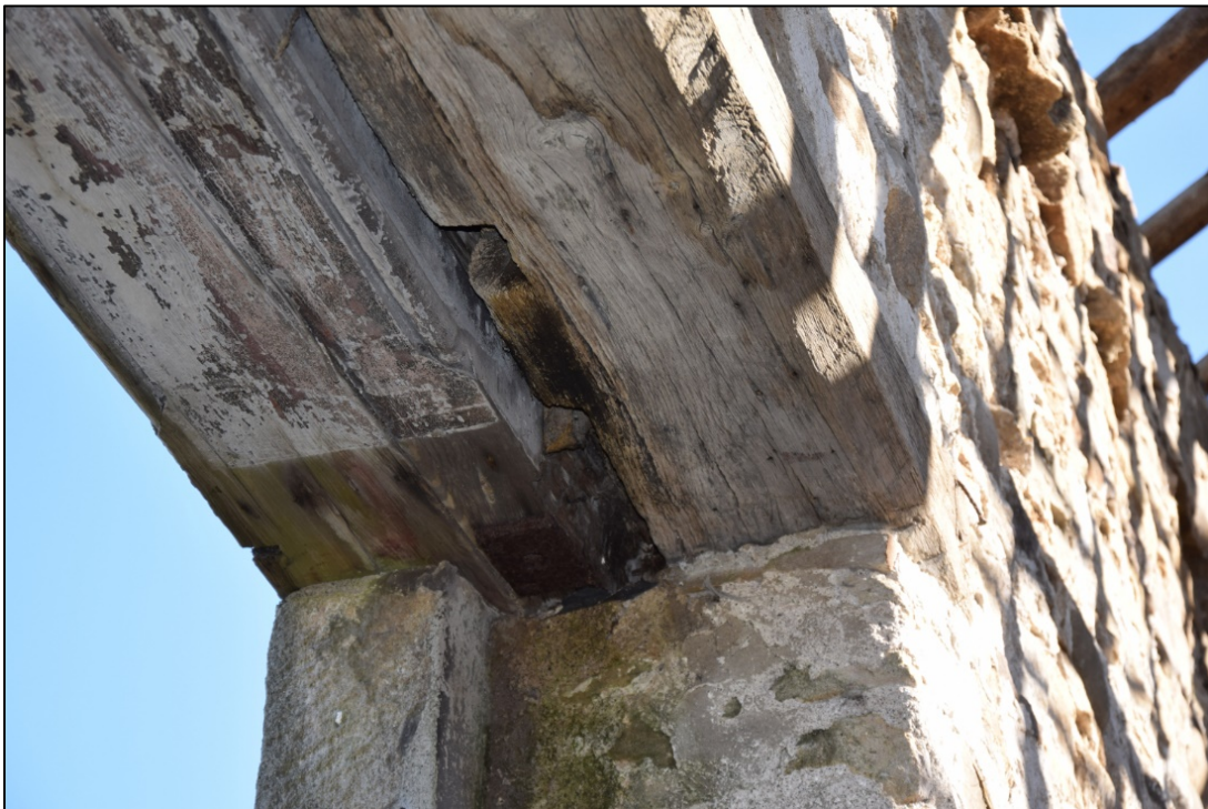
Photograph 46: Re-used timber in the lintel of the 20th-century door on the north side of building 2
