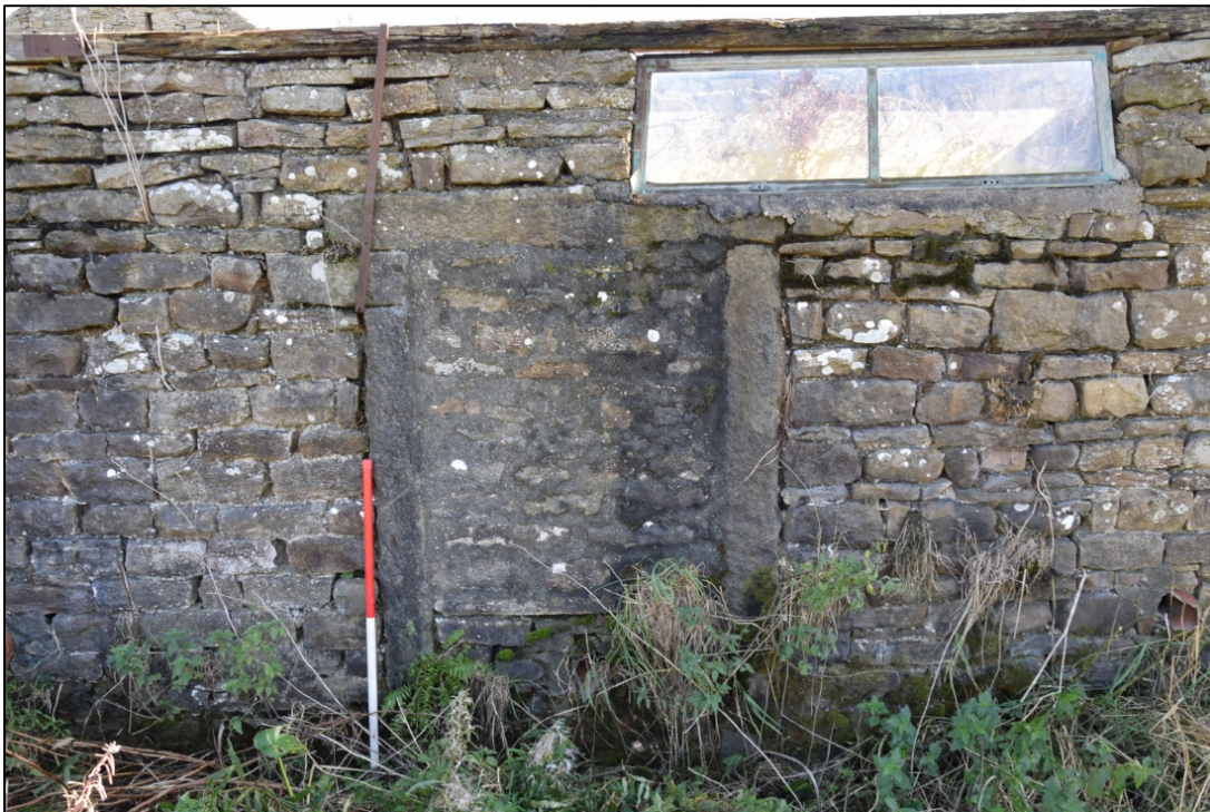
Photograph 52: Detail of the blocked door, later reduced to a window, in the west face of building 4
