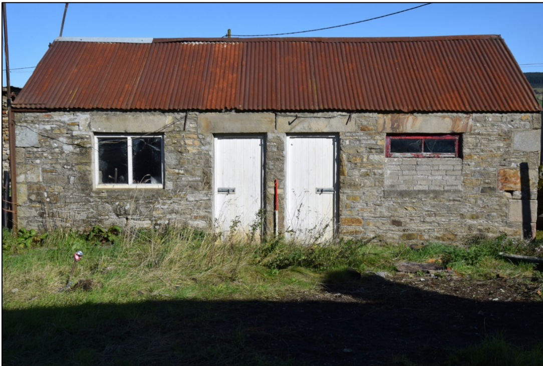
Photograph 64: The south face of building 5
