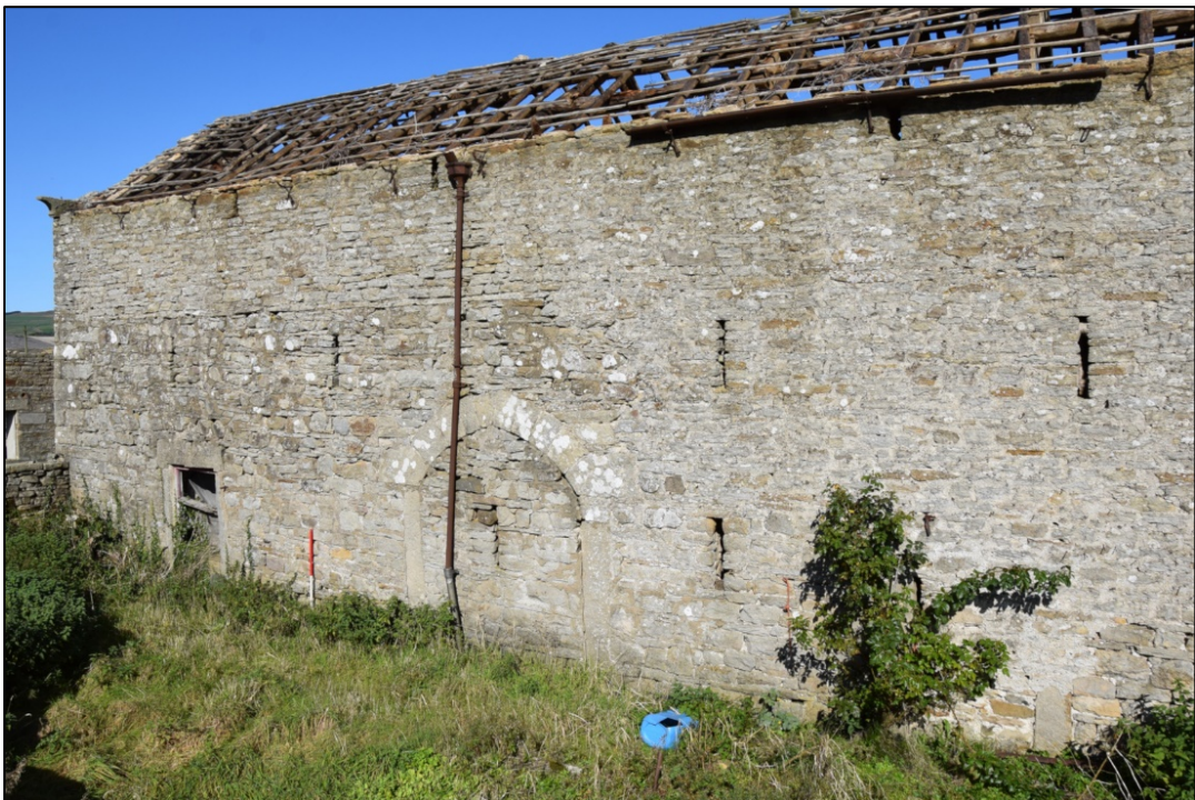
Photograph 32: The small door at the far end was matched by another at the east; the lower jambs can be seen below the shrub at the right
