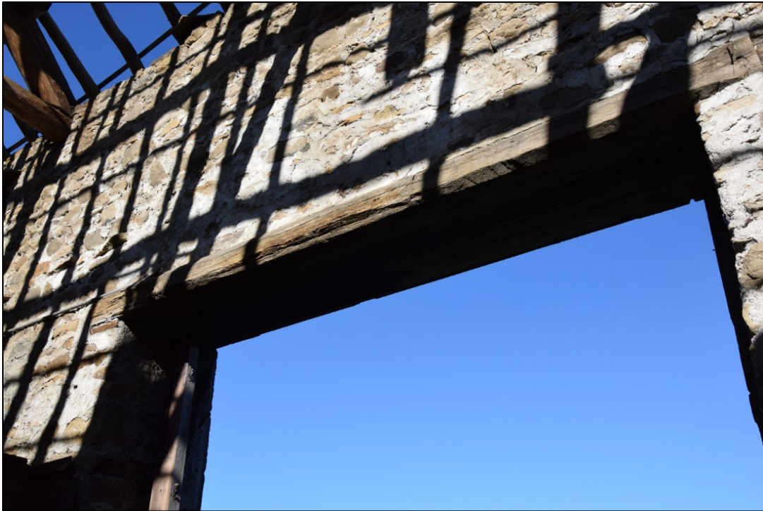
Photograph 45: The centre of the north wall and the later door
