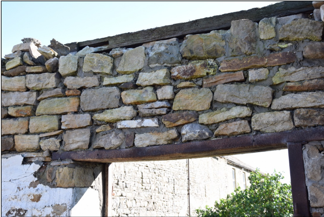
Photograph 59: Detail of steelwork and reset masonry above the south door
