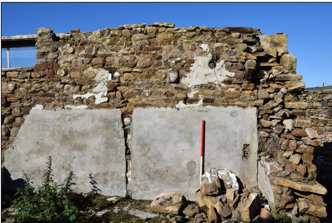
Photograph 56: The stubs of two joists can be seen above the cement render at the north-west corner of building 4
