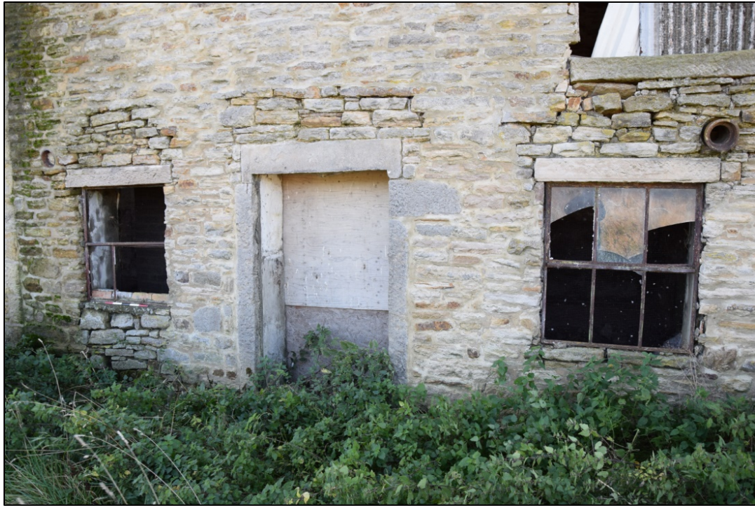
Photograph 13: The door and windows in the extension match those in the older block. The pipe is a ventilator for the cow byre
