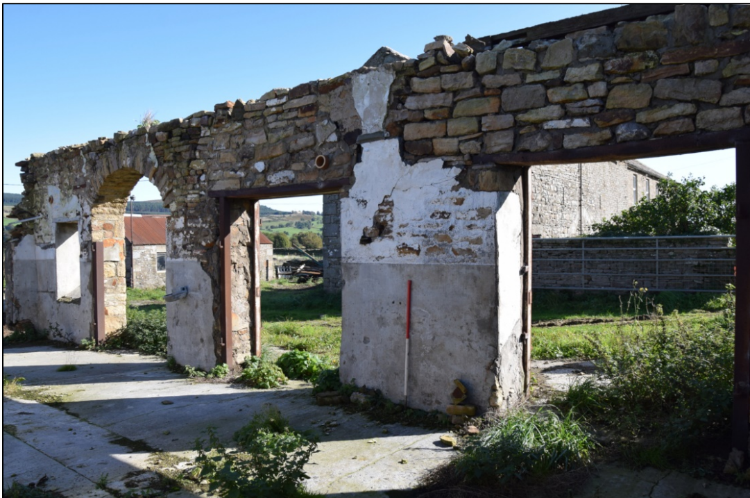
Photograph 58: Much of the upper part of the east wall has been rebuilt in recent times
