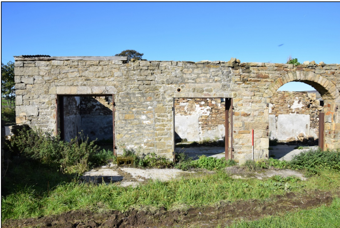
Photograph 48: Steel frames support the doors at the south end of the building's east face
