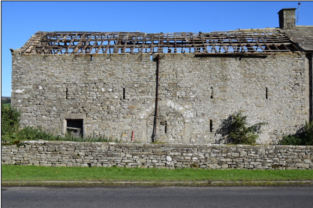
Photograph 31: The south face of building 2. The change in fabric can be seen as a neat horizontal line above the left-hand pair of breather slits
