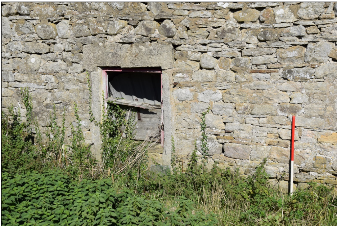
Photograph 34: The west door is partly blocked to form a window for the byre
