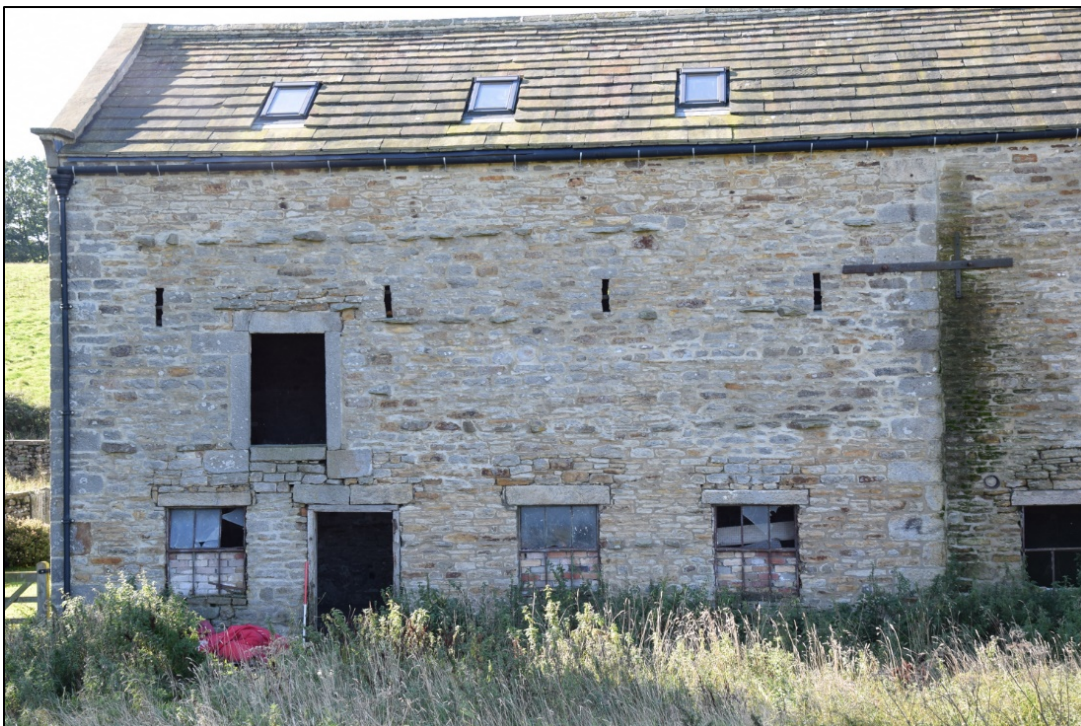
Photograph 10: The north face of the older part of the building
