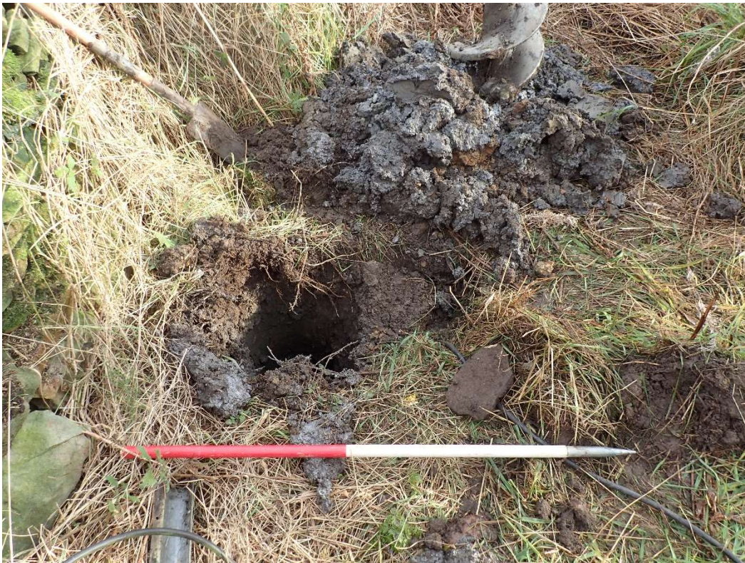
Photograph 2: Telegraph post hole after excavation with auger, looking east
