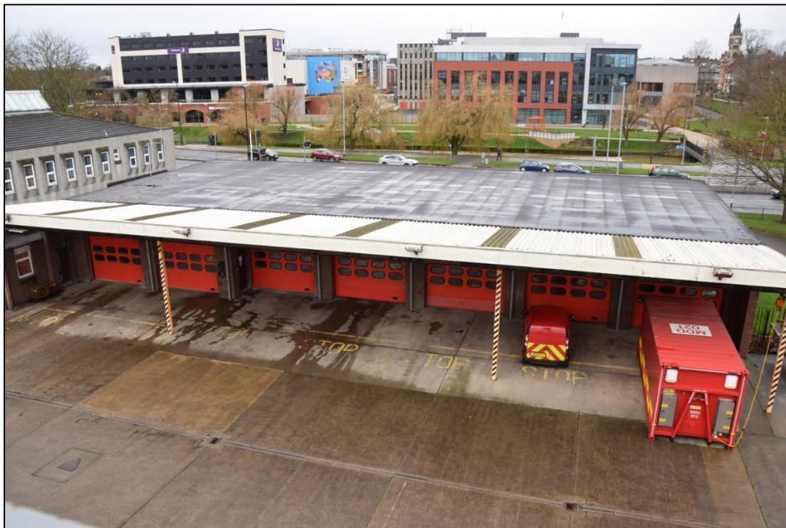
Photograph 14: The drill yard face of the garage and the canopy. A view looking west
