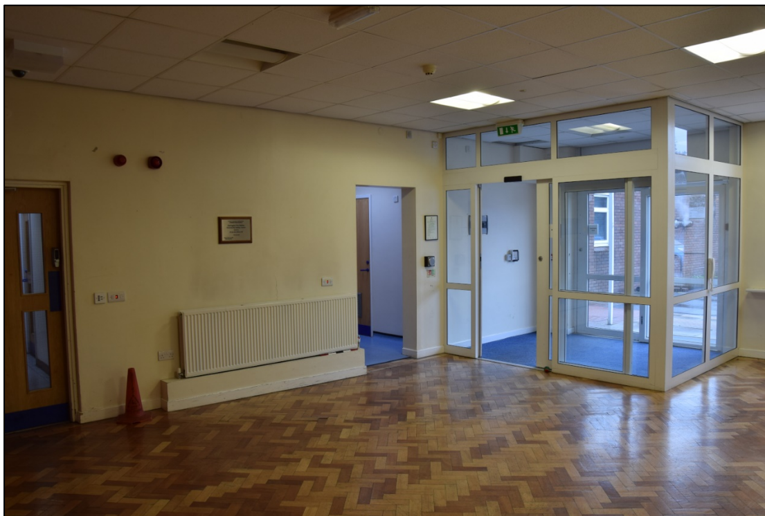
Photograph 22: Entrance foyer 5 in the former Community Safety Centre. A view looking north-east
