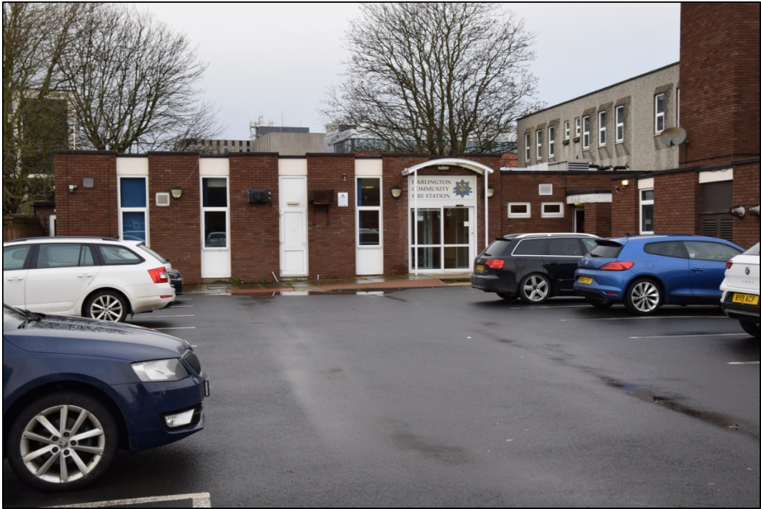
Photograph 11: The entrance to the former Community Safety Centre, seen from the car park
