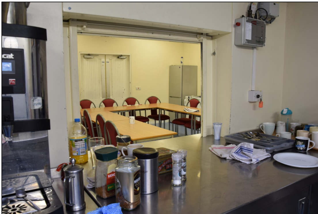
Photograph 26: The hatch between the kitchen and the mess room 11
