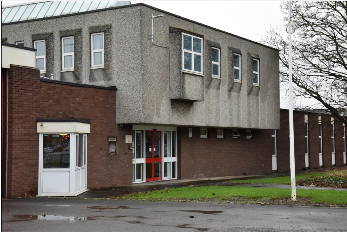
Photograph 9: The offices, seen from the north-west. The projecting ground-floor window of the watch office gives a view of vehicles leaving the station
