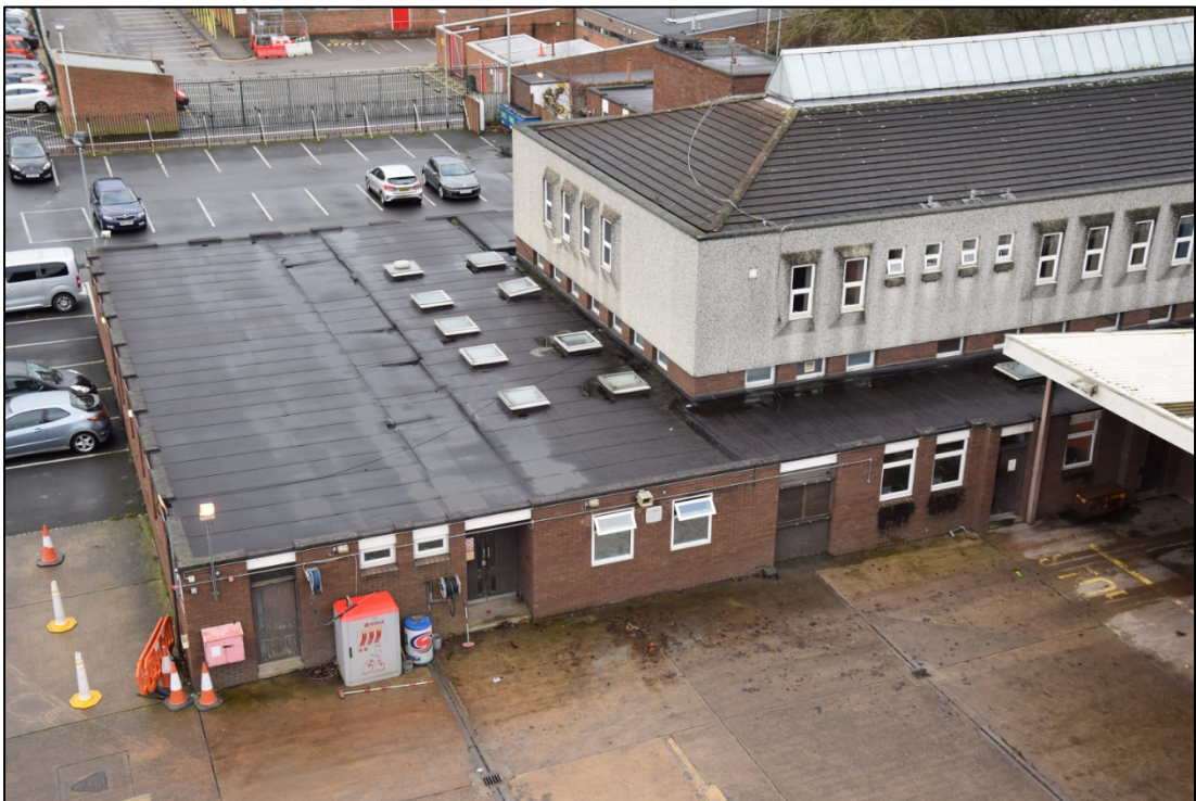
Photograph 12: The east wing of the building, between the drill yard and car park. Above, the long skylight runs over the central corridor and parts of the southern offices on the first floor
