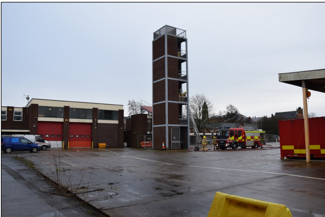
Photograph 2: The drill yard and tower with the ambulance station at the left
