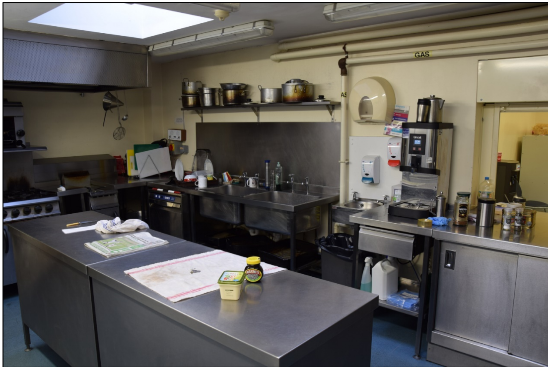
Photograph 25: A view looking north-west in the kitchen
