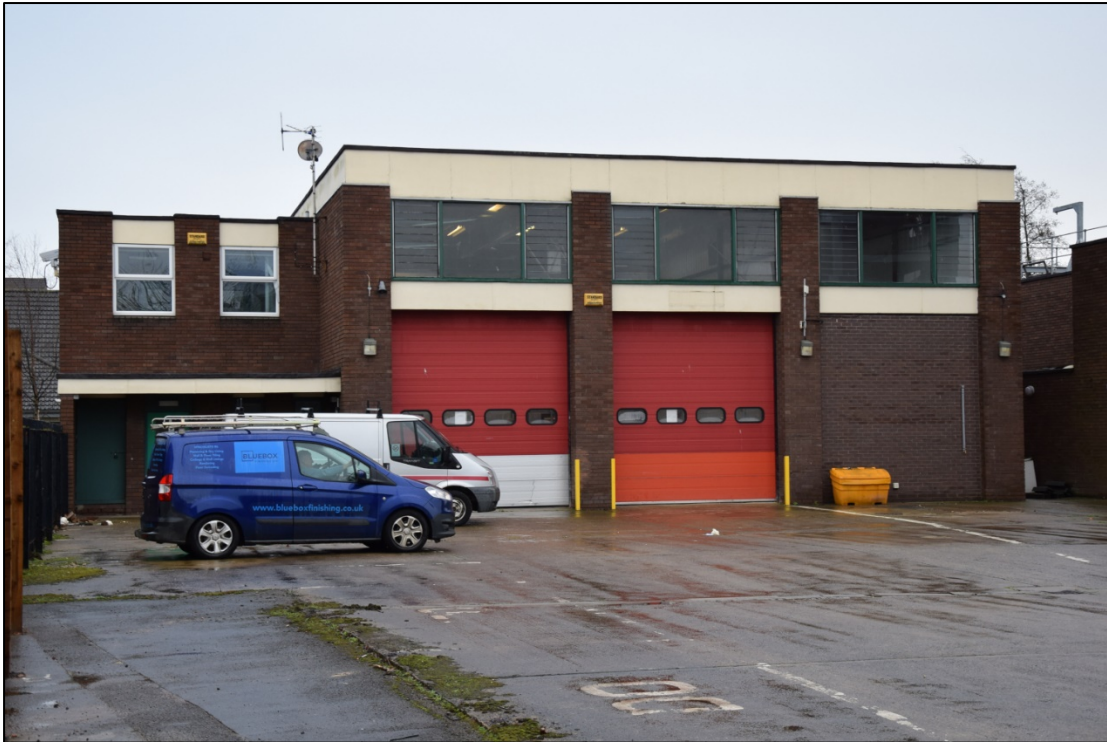
Photograph 3: The west face of the ambulance station, which was being refurbished at the time of this survey
