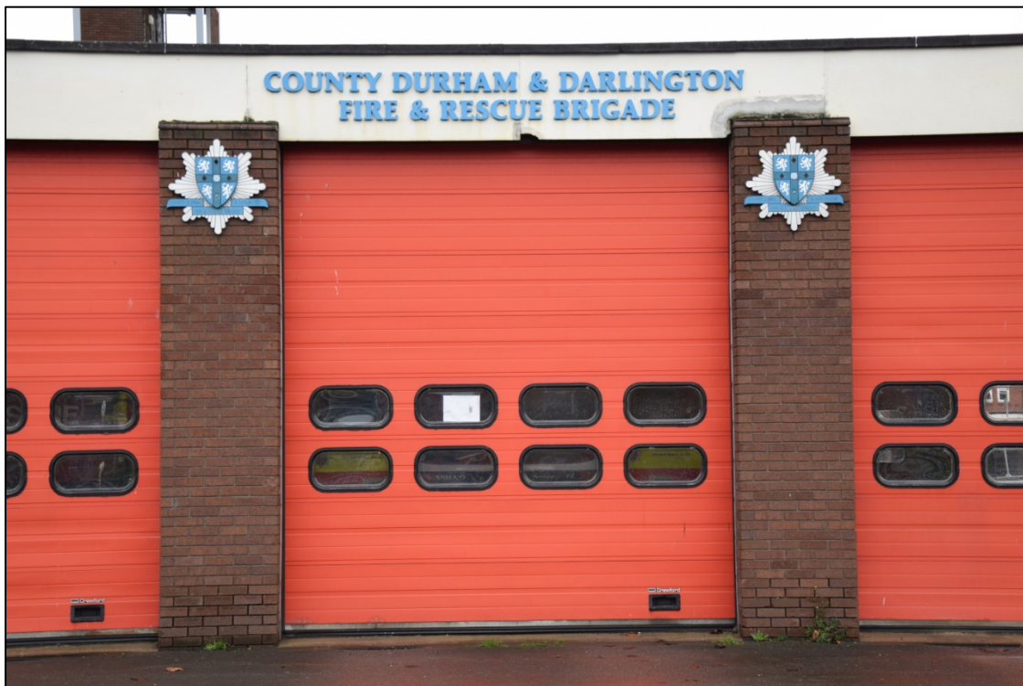
Photograph 8: The central bay of the engine garage
