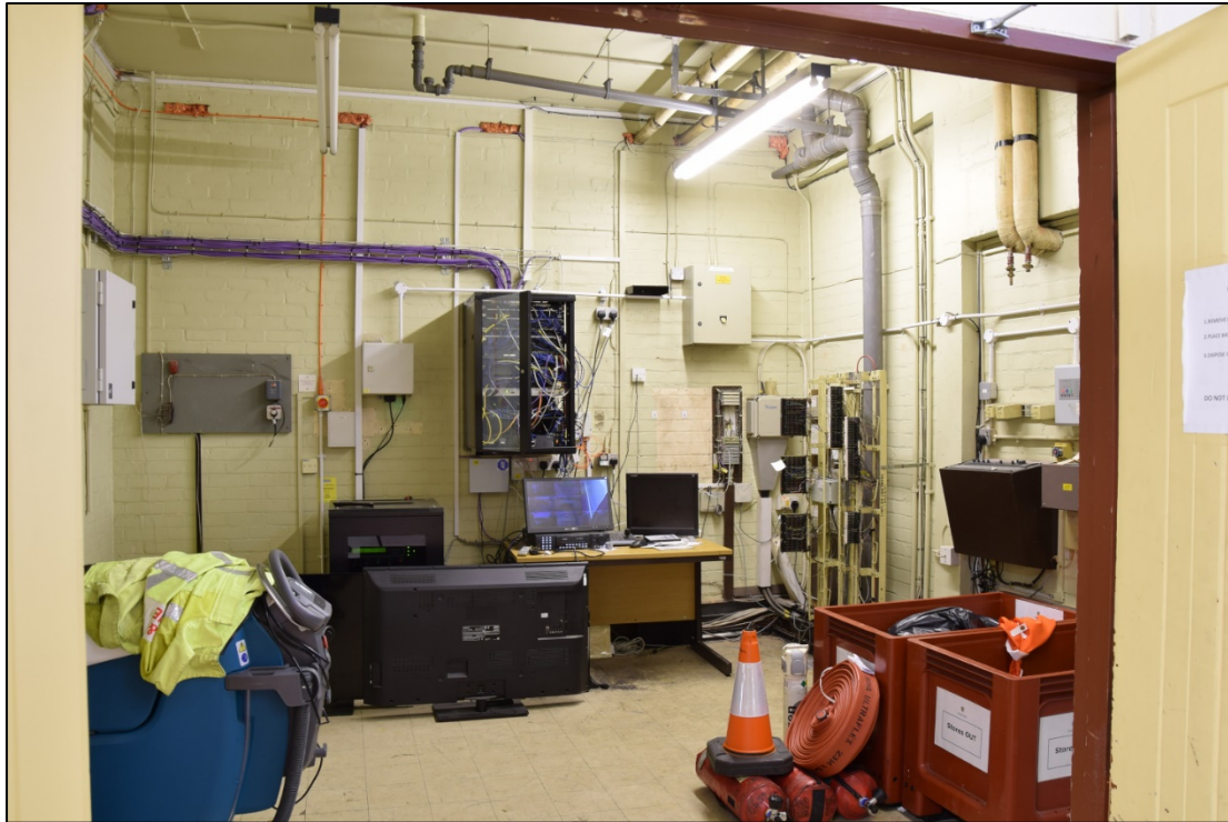
Photograph 33: Looking west into store room 18
