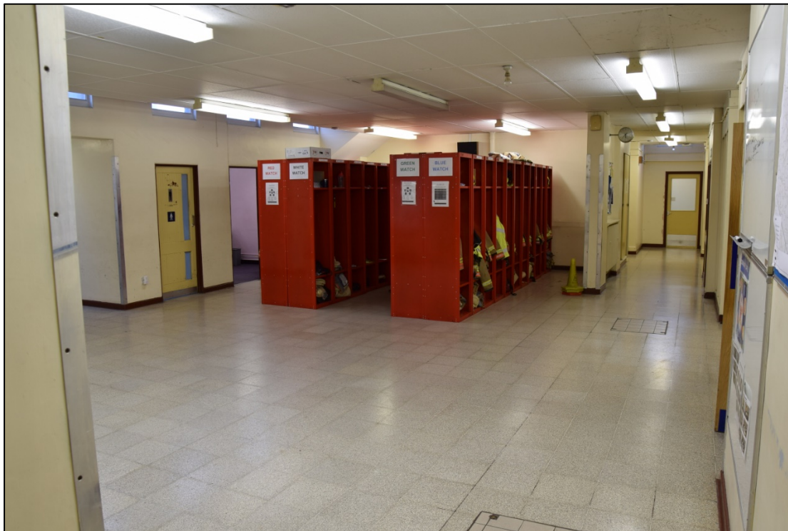
Photograph 34: The muster hall 19, seen from the north-west corner
