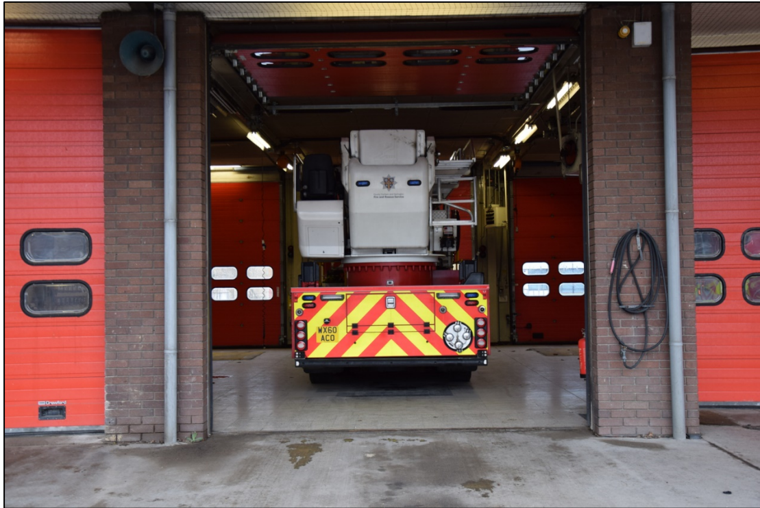
Photograph 47: The long eastern bays of the garage, seen from the drill yard
