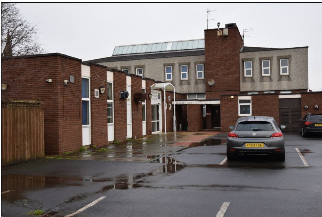
Photograph 10: The south end of the fire station, with the former Community Safety Centre rooms at the left. The central brick tower contains the secondary staircase and boiler flues from the plant room
