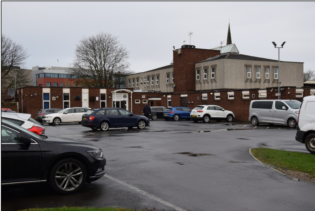
Photograph 5: The fire station seen from the south-east, across the car park
