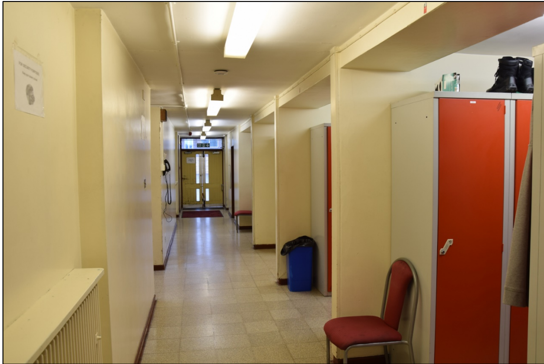
Photograph 45: Looking north-east along the locker room 29 towards the drill yard door
