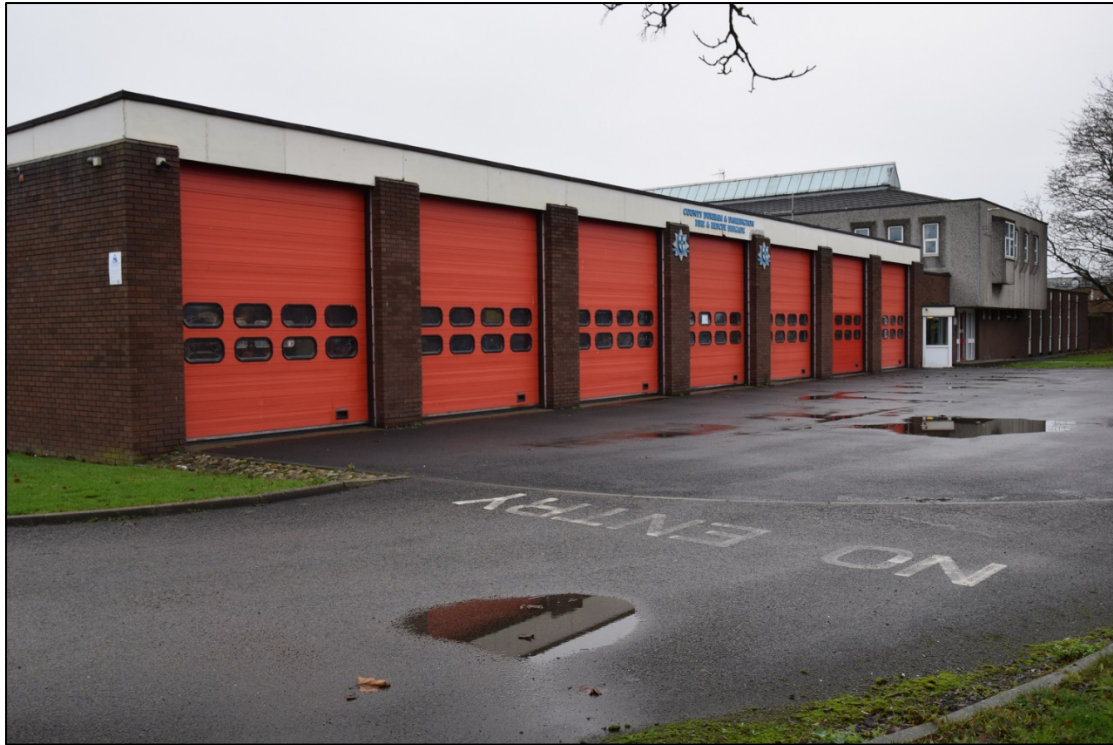
Photograph 7: The garage seen from the north-west
