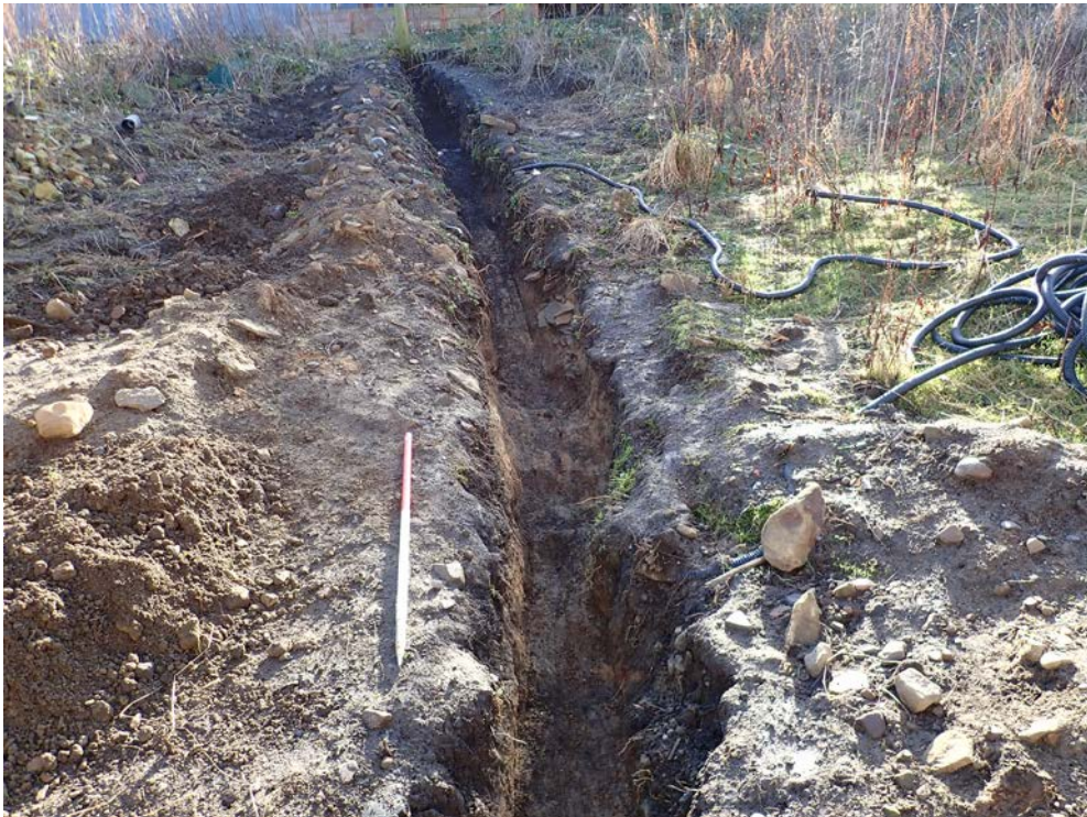
Photograph 2: Trench, looking south-east
