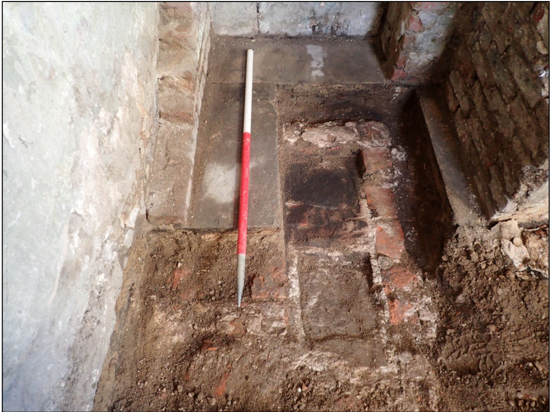
Photograph 37: The hearth for the copper was revealed when the flags were lifted
