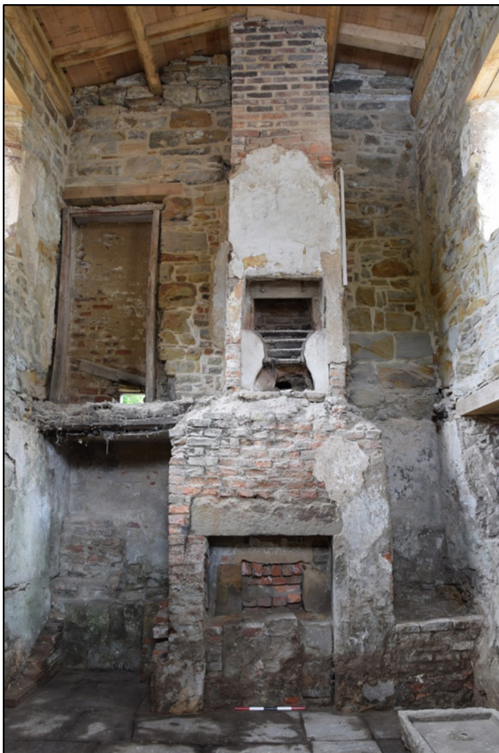
Photograph 33 (above): A later structure for a stone shelf or a sink, at the north-west corner of the ground floor
