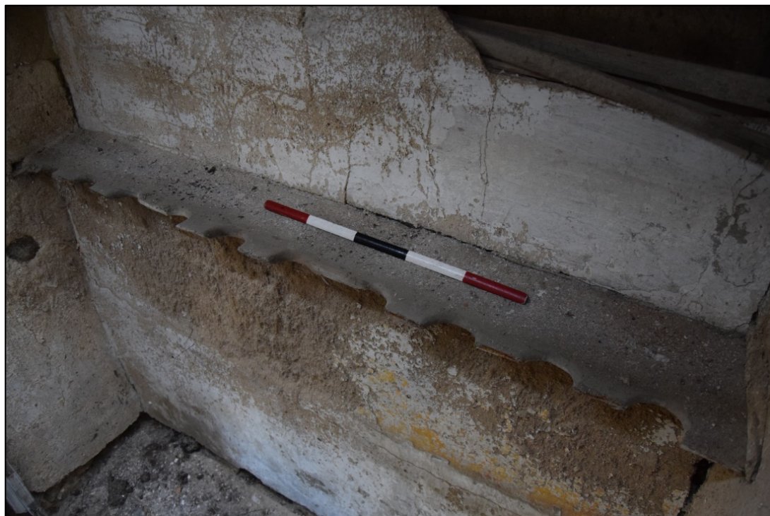
Photograph 46 (below): The remains of the shotgun rack in the upper window of the west wall
