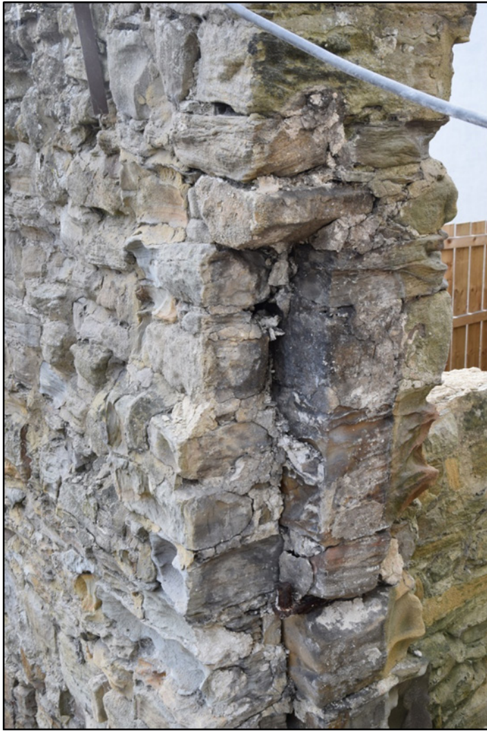
Photograph 49 (left): The rebate on the south side of the gateway; compare with Photograph 14. An iron hinge pintle can be seen towards the bottom of the picture
