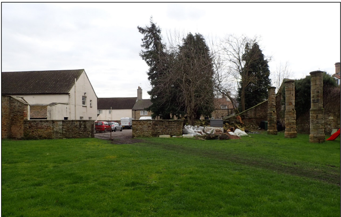
Photograph 4: The view from the north end of the west court, showing the west wall, sloping wall and three piers of the former Dutch barn hay shed
