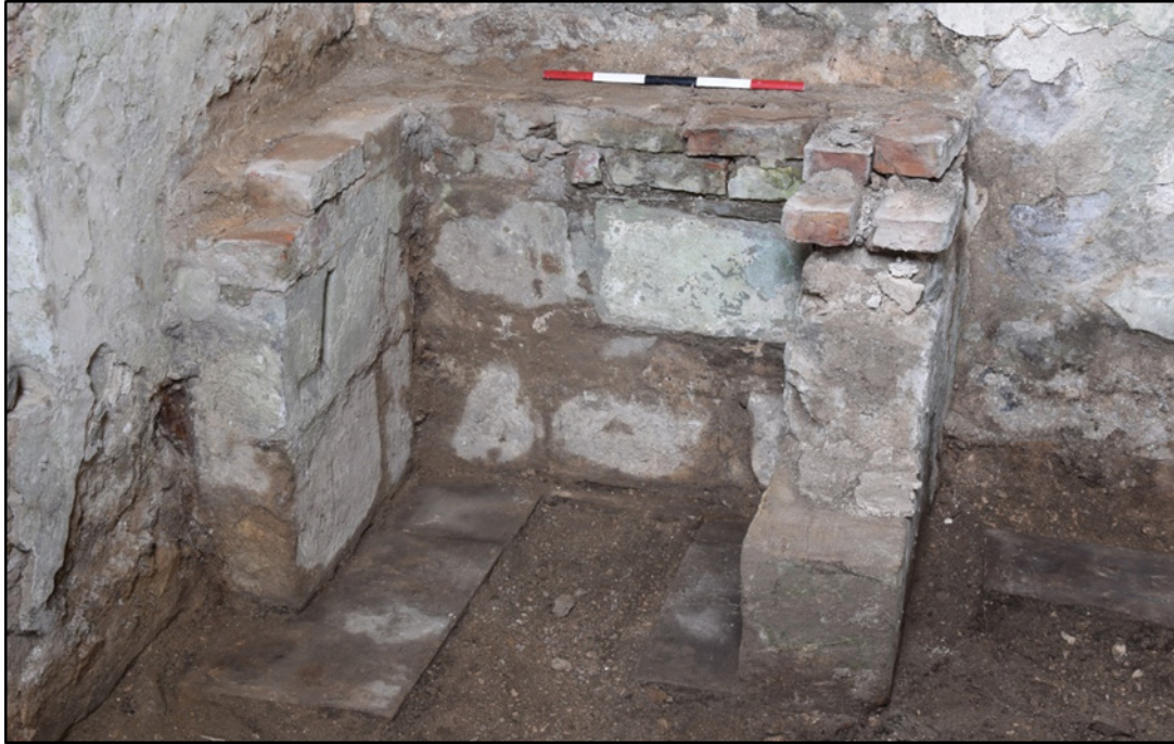
Photograph 33 (above): A later structure for a stone shelf or a sink, at the north-west corner of the ground floor
