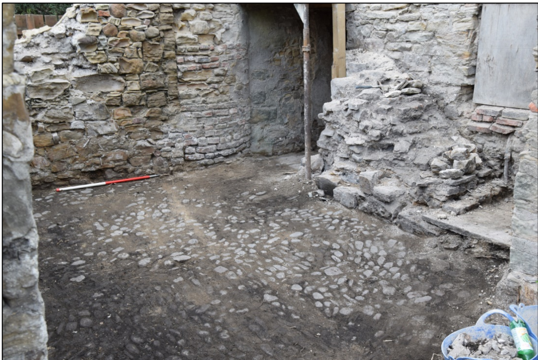
Photograph 52: The cobbled surface of the yard is above the level of the floor in the tower
