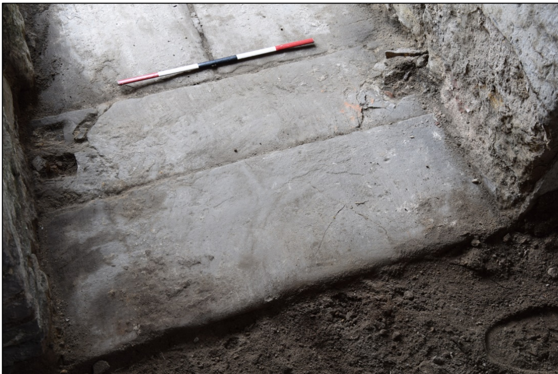
Photograph 40: The threshold and sockets for door frames; there was a step down to the flagged floor
