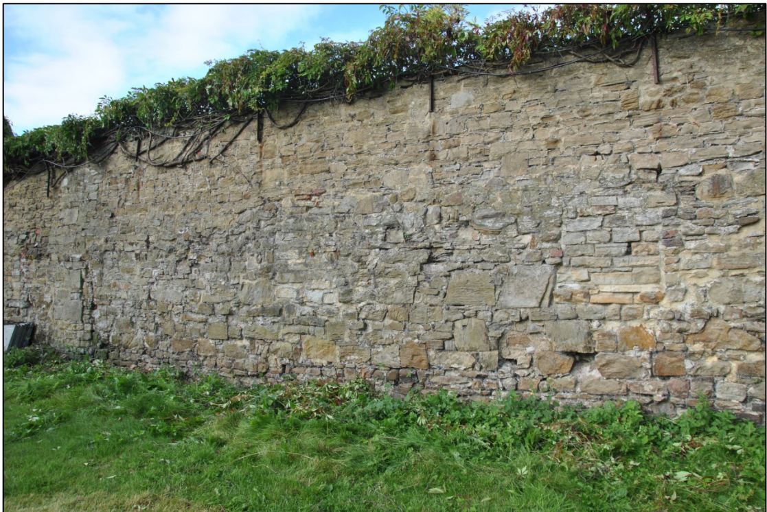
Photograph 12: The change in masonry [16] is visible above blocked openings [9] and [10] here
