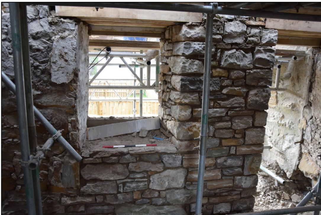
Photograph 44: The same wall after rebuilding, with a smaller window. The straight joint at the left continues below the new sill
