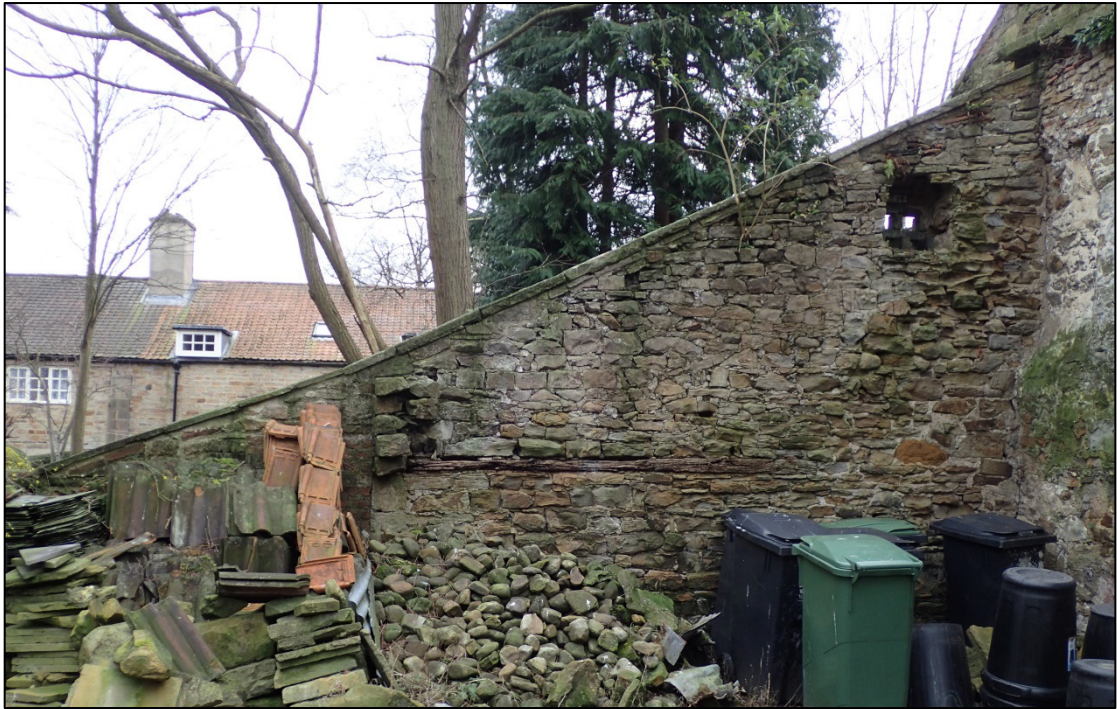
Photograph 3: The north face of the sloping wall and traces of the 19th-century cow-house. An old roof line visible beneath the dovecote opening, top right, is what remained of the privy shown on the 1830s drainage plan
