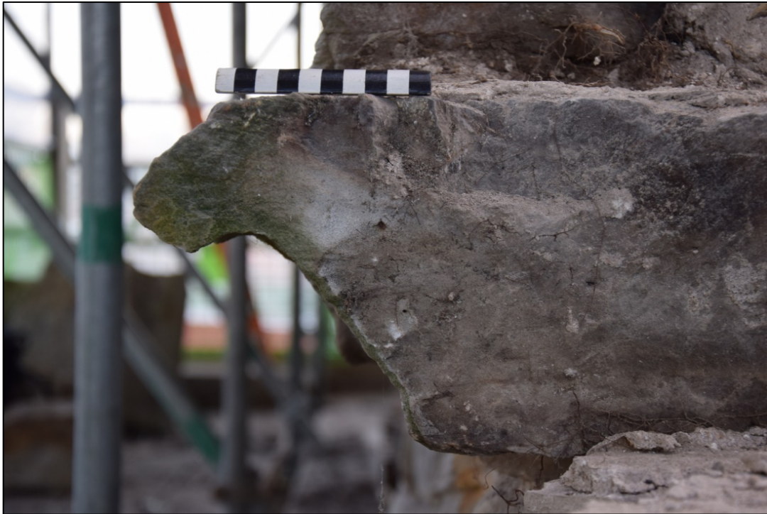
Photograph 29: One of the few undecayed sections of the string course
