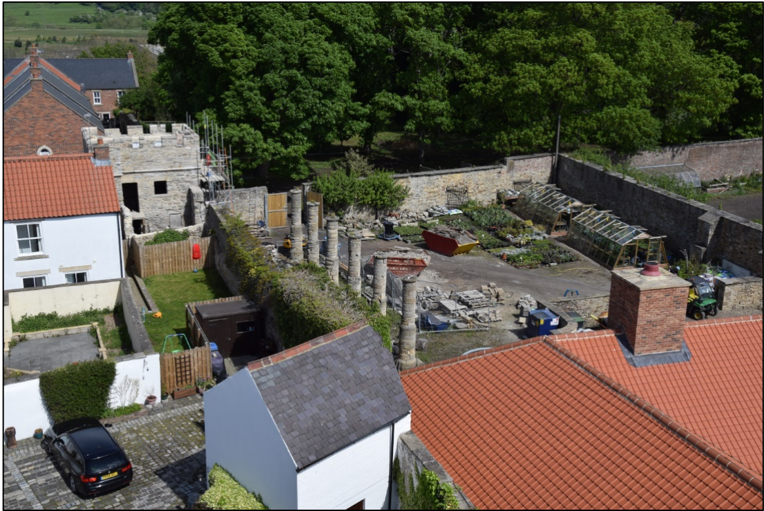
Photograph 1: The site seen from the Welcome Tower to the south-west. The mural tower is the battlemented building, top left, and the west curtain wall runs diagonally past the new red-roofed Energy Centre at the right
