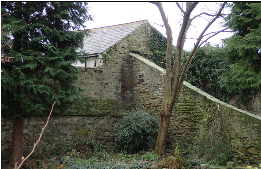
Photograph 2: The south end of the west curtain wall, seen from the south-east. The sloping wall running up to the gable of the building outside the site marks the south end of the old dung pit. Note the brick chimney in the angle between the stone walls
