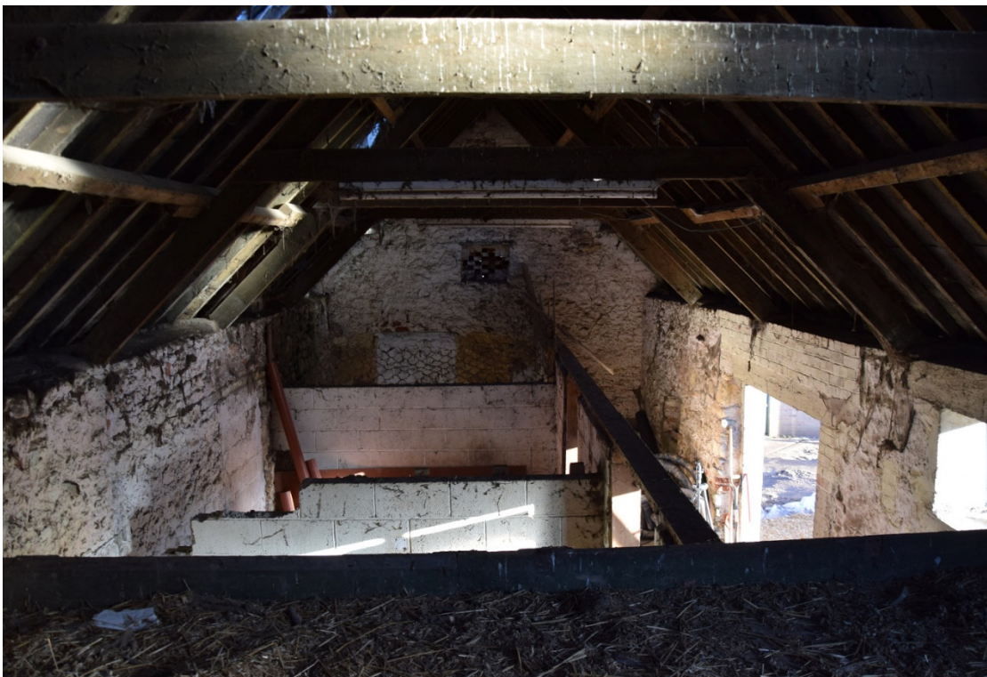
Photo 24: A view looking east in the old barn. The low walls are modern insertions
