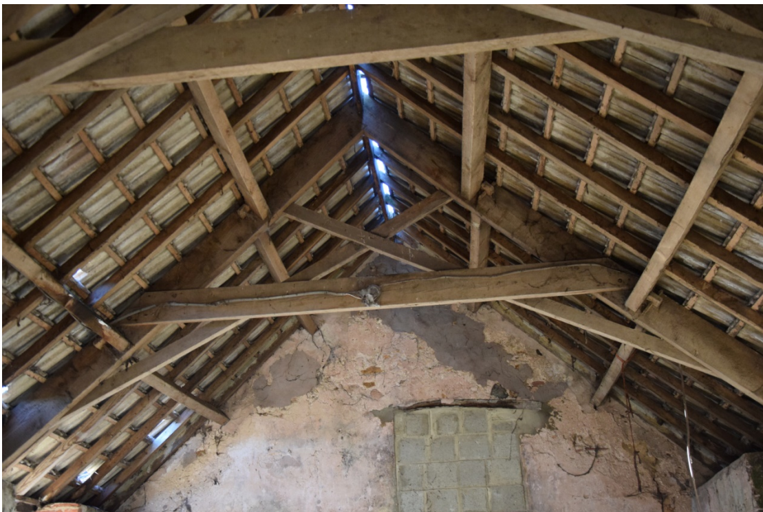
Photo 14: The roof trusses have small scissor braces above the collar beams
