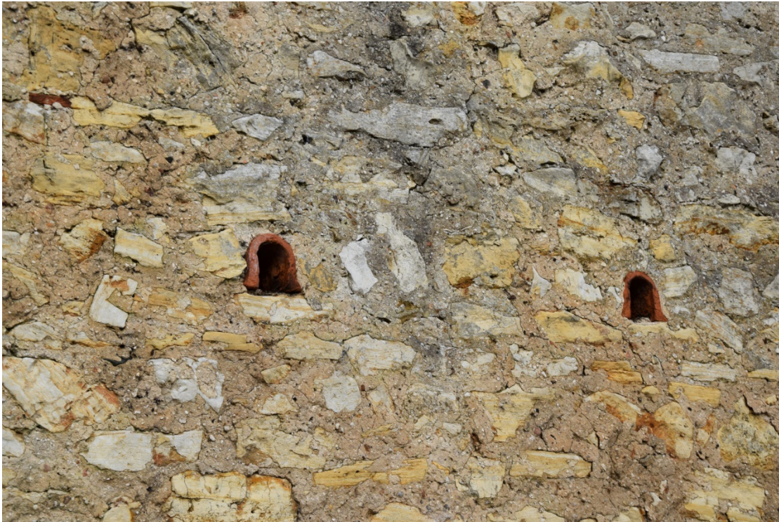
Photo 5 (above): Old horseshoe field drains used as ventilators for the byre
