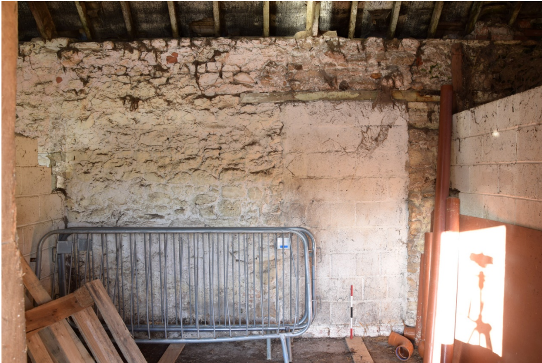
Photo 29: A blocked north door in the middle room
