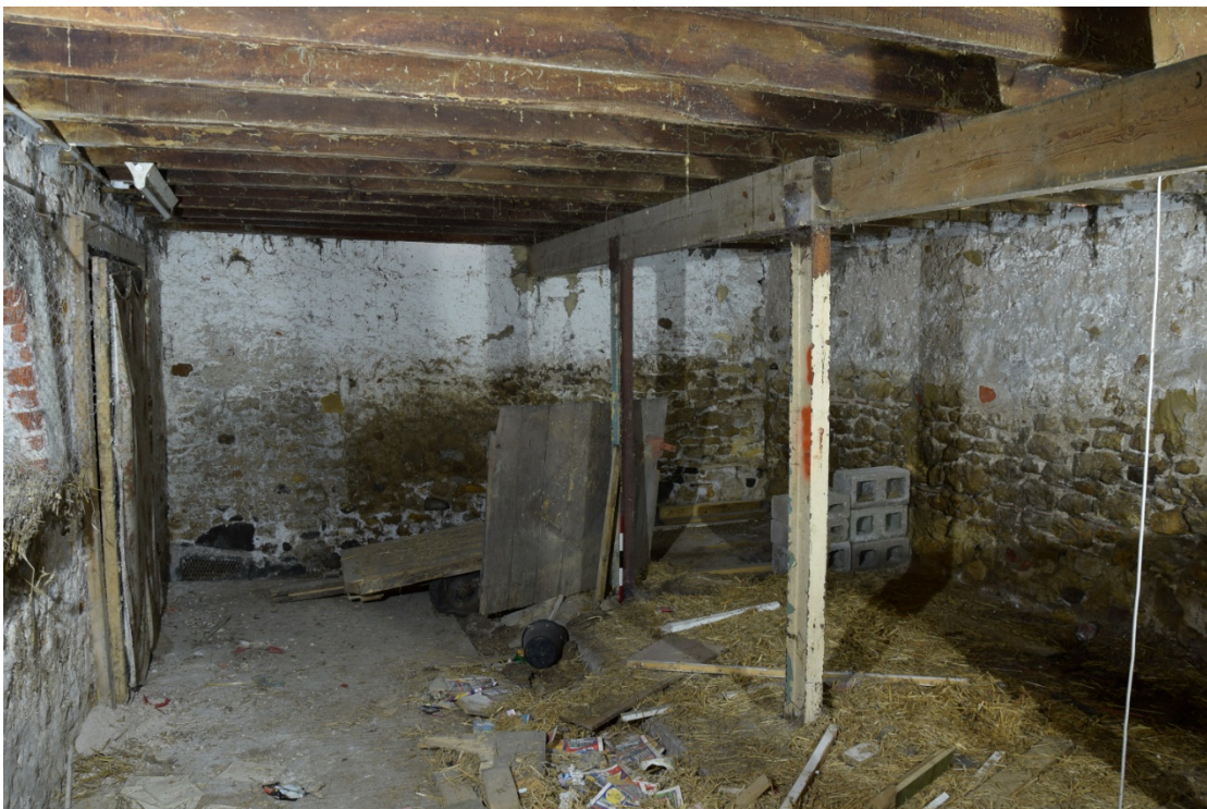
Photo 10: The interior of the byre seen from the north-west corner. The black bucket is lying in the drain at the back of the stalls
