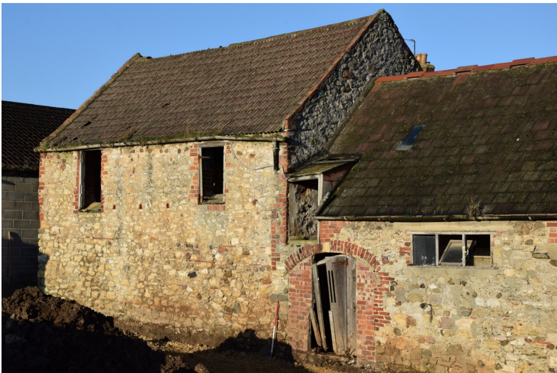
Photo 4: The lower pitching door at the south-east corner of the byre is a later alteration
