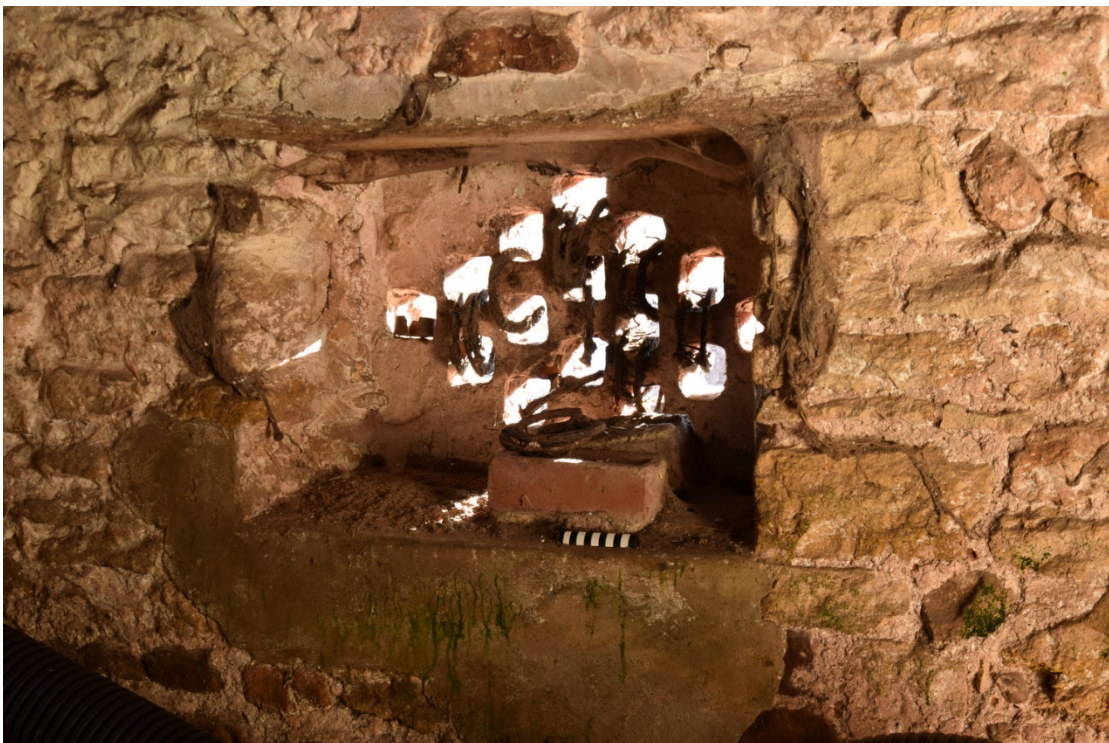
Photo 20: The inside of the ventilator
