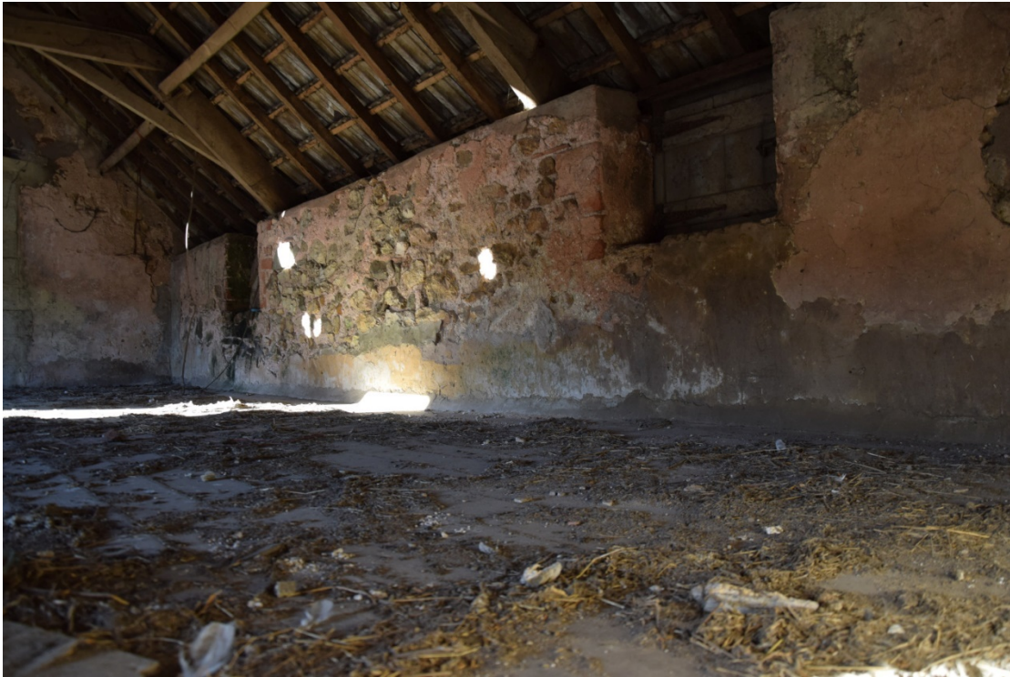
Photo 15: Small windows in the north wall of the loft
