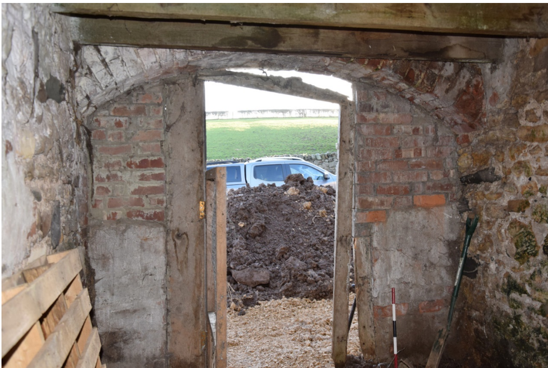
Photo 26: Modern brickwork reduces the size of the old arched door
