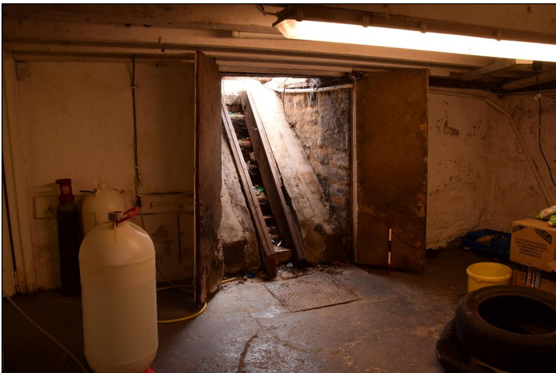
Photograph 38: The east wall of the cellar and the barrel drop
