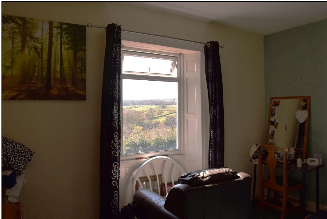
Photograph 31 (above): The bedroom has panelled window splays like those seen elsewhere in the building
