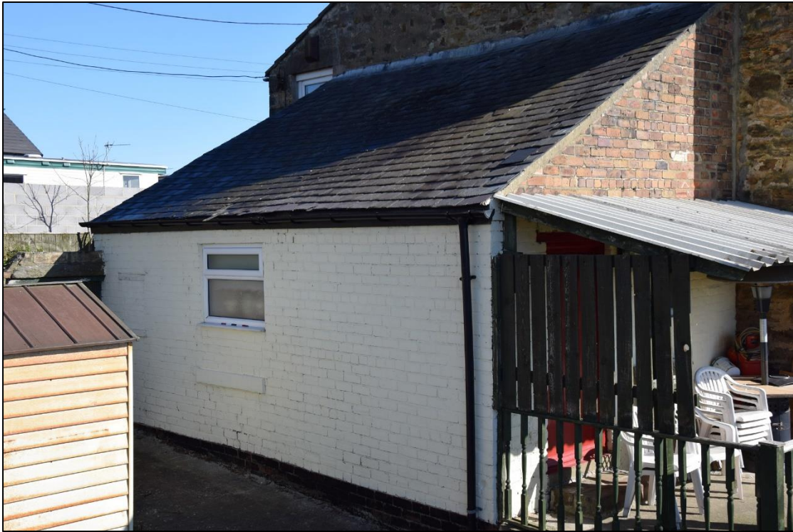
Photograph 9: The west end of the games room has a small blocked opening at the extreme left and a reduced window opening at the centre
