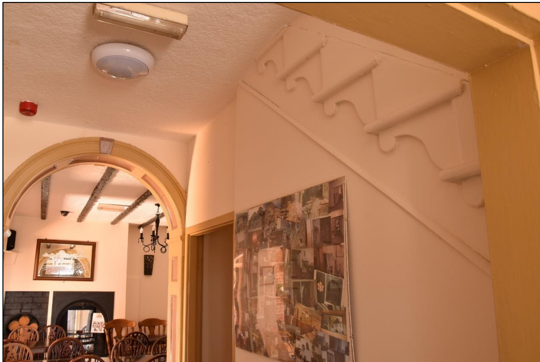
Photograph 23 (above): Moulded tread ends on the exposed stairs in the hall.
