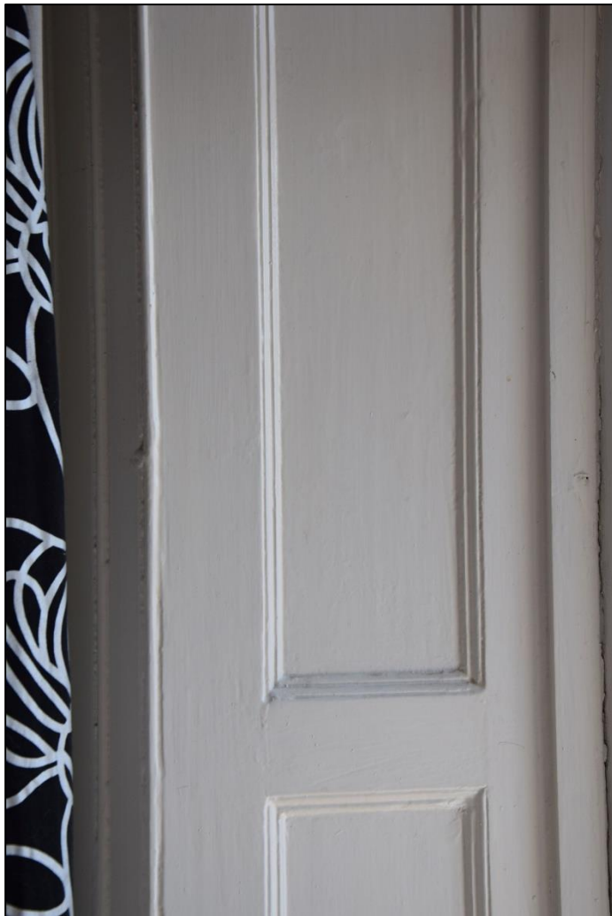
Photograph 31 (above): The bedroom has panelled window splays like those seen elsewhere in the building
