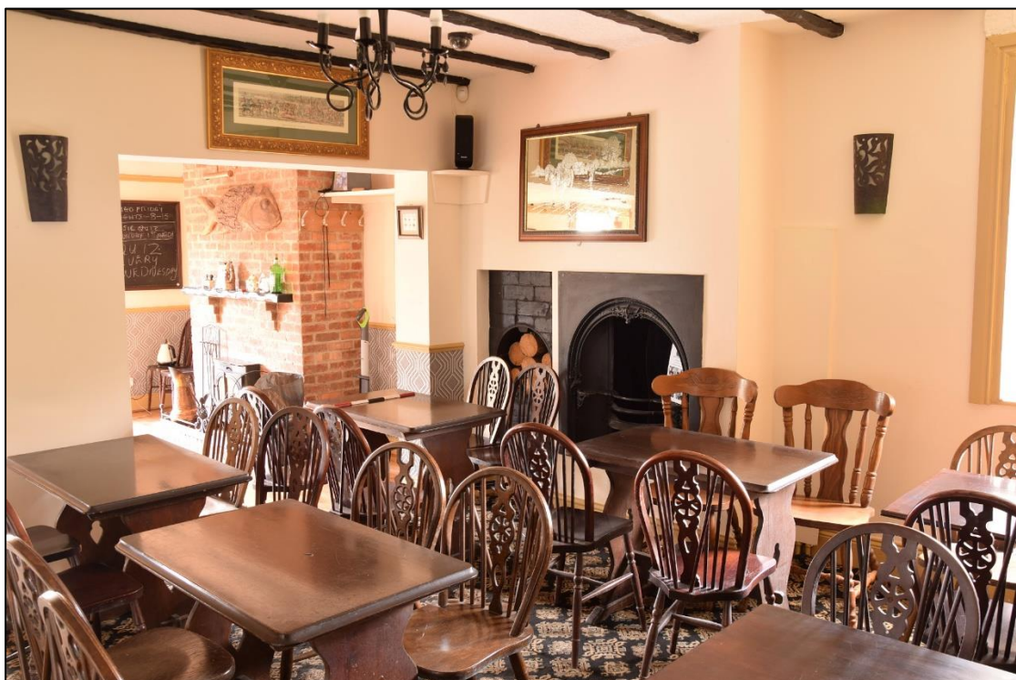
Photograph 18: Both of the chimney breasts in the west wall of the bar have been altered
