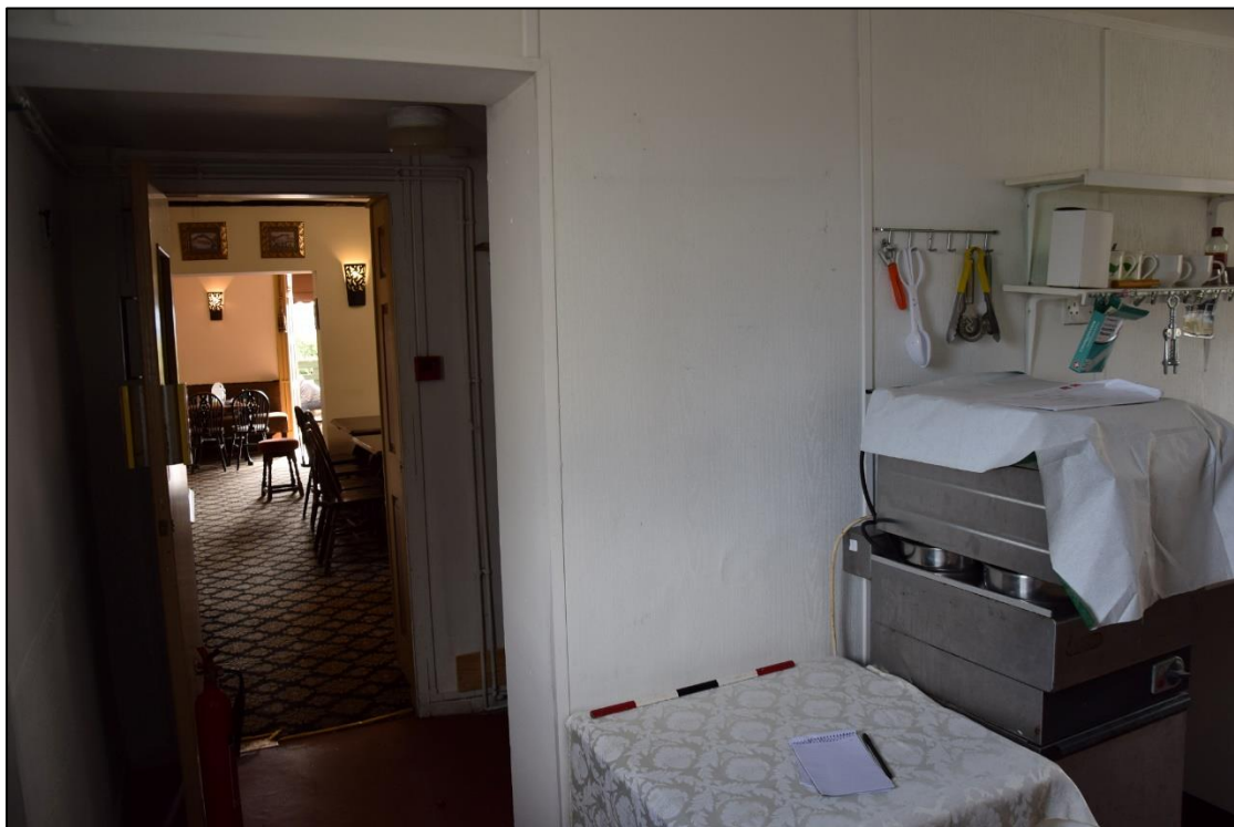
Photograph 20: A view looking south-west from the kitchen. The space beside the door is the old back passage of the original house
