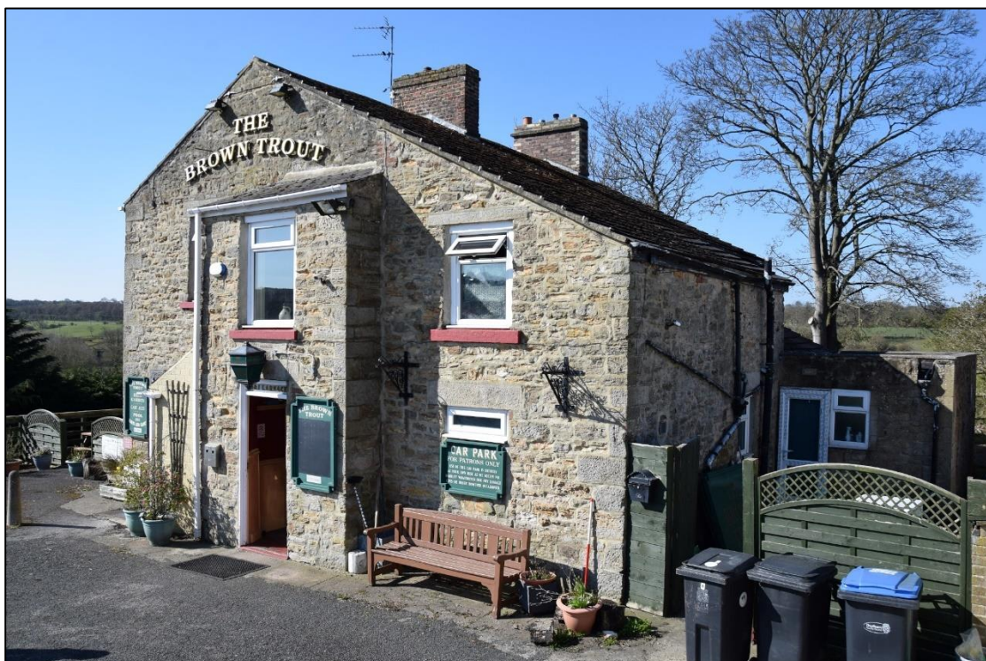
Photograph 2: The substantial two-storey rear outshut at the middle of this view does not run the full length of the building
