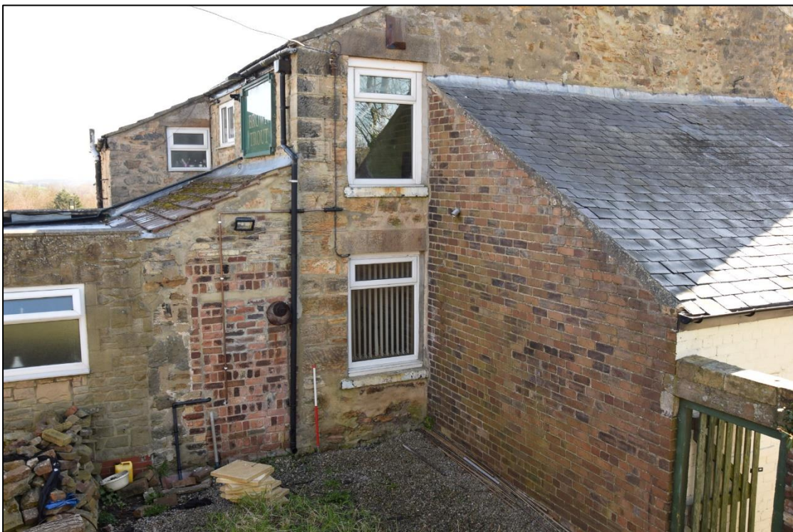
Photograph 10: The north-west corner of the building, showing modernised windows and the bricked-up door of the rear passage
