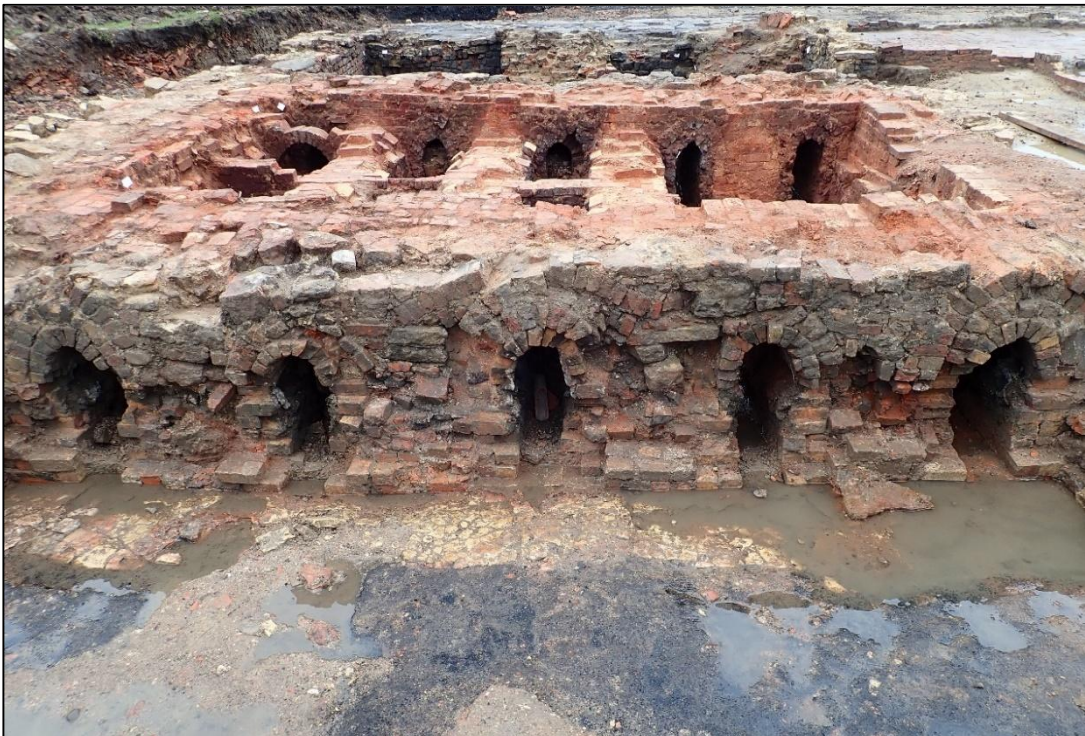
Photograph 20: The north face of the Scotch kiln. Fan-shaped areas of purplish heat-affected brick can be seen above the stokeholes in the far wall
