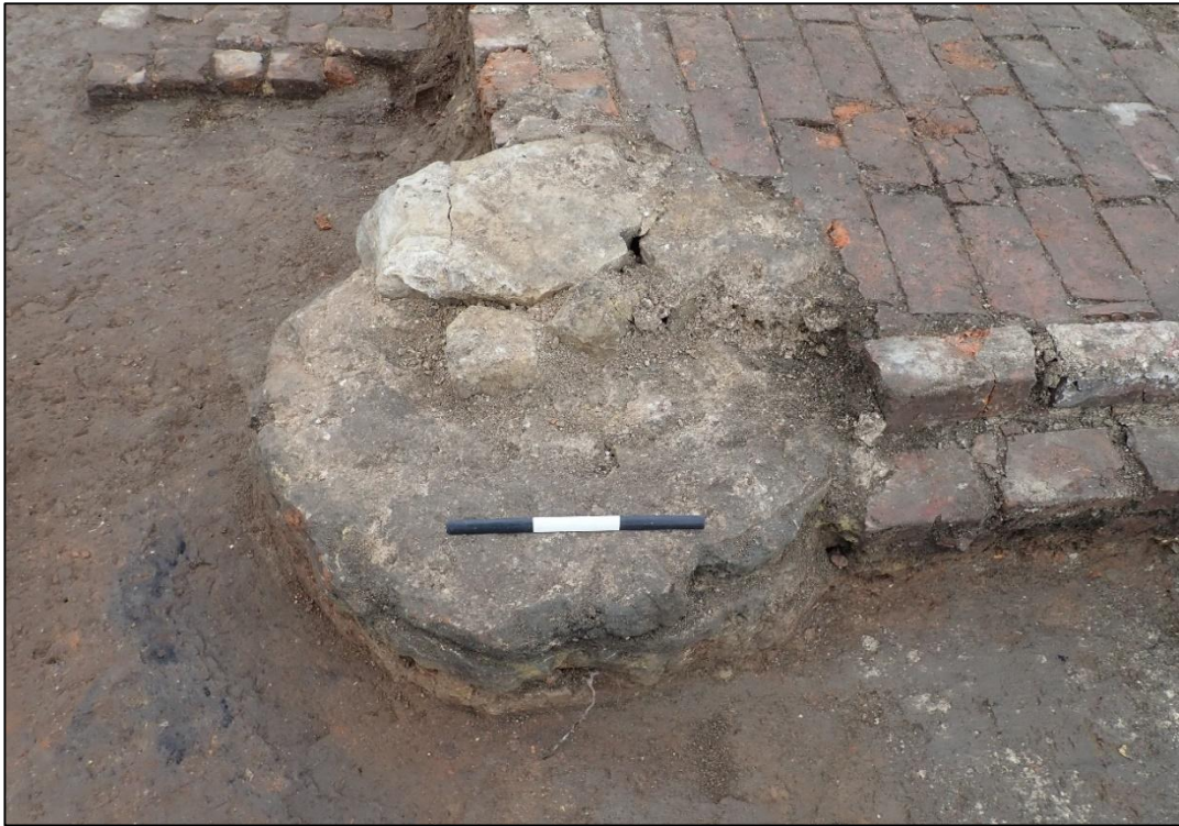
Photograph 33: Plinth [F91], the central support for the roof of the moulding shop. A view looking south
