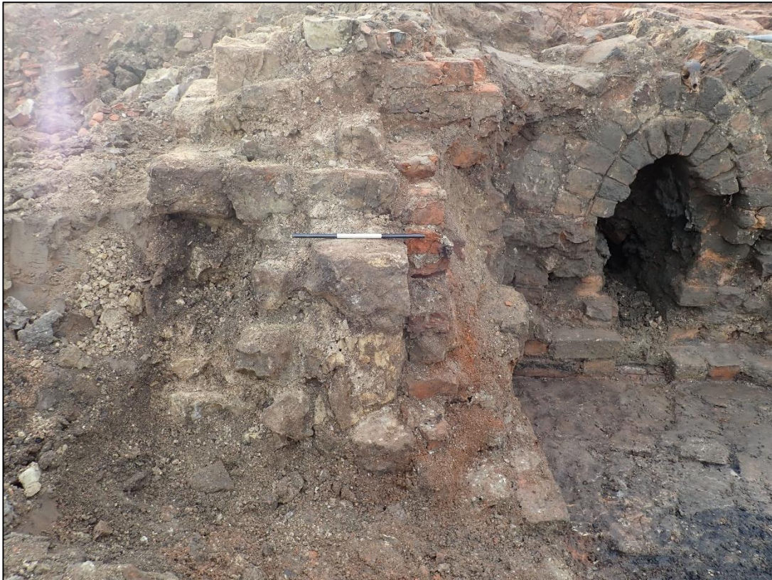
Photograph 9: The east wall of furnace room 57 is stone with a brick lining. A view looking south
