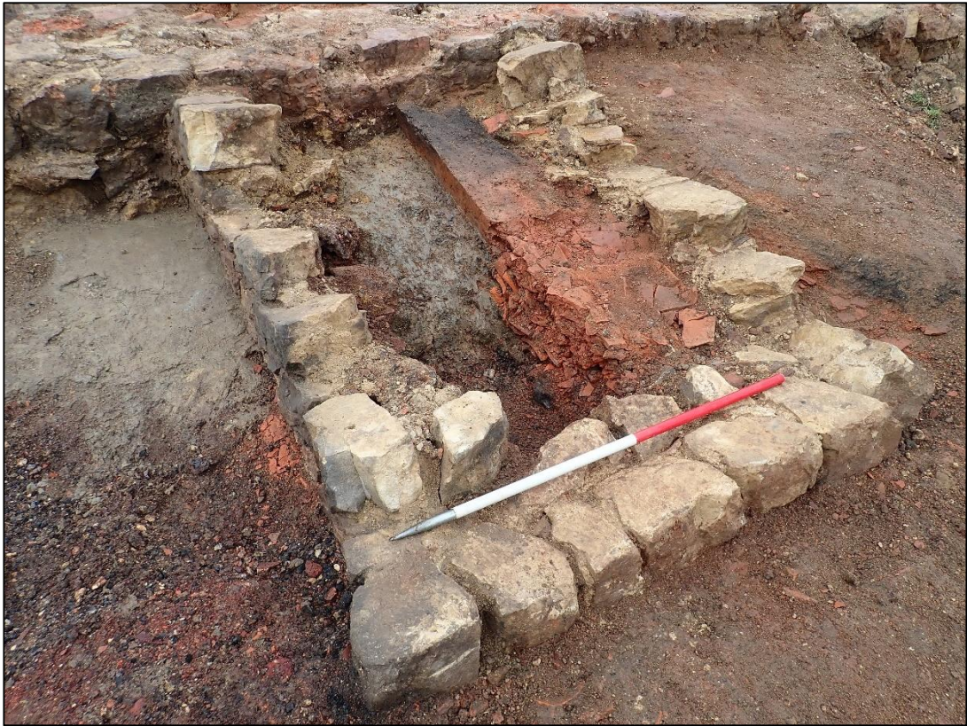
Photograph 31: The foundations of the buttress [F165] at the east end of the kiln have cut through the waste tile fill of the clay pit in the foreground. A view looking north-west
