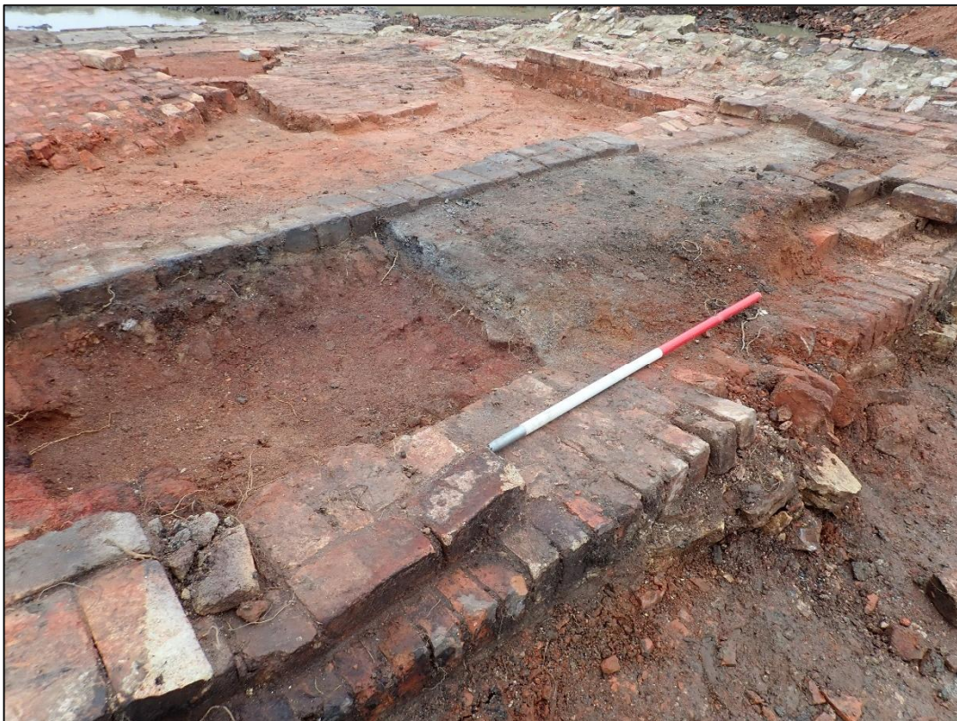
Photograph 78: The base of the outer wall of the Newcastle kiln [F205] and the thinner flash wall [F203]. Part of the grey firing waste deposit [204] has been excavated. The kiln door was around the far end of the scale. A view looking west
