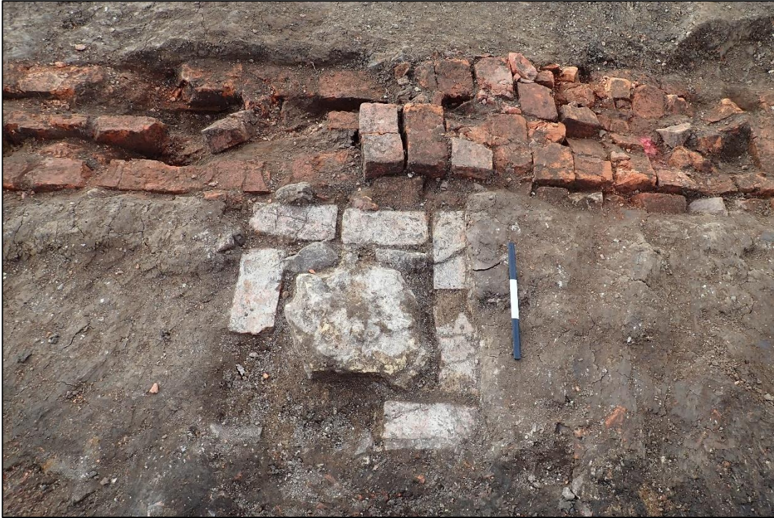
Photograph 53: [F23], one of the brick and stone plinths that carried the roof supports in the drying shed 30. A view looking west
