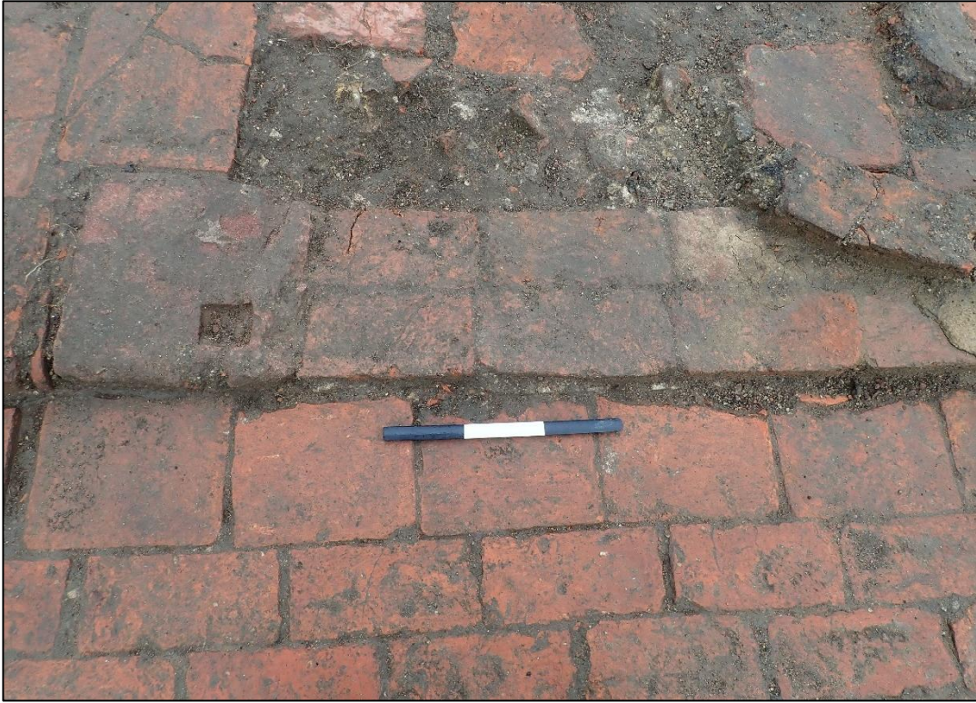
Photograph 35: A socket for a jamb or a hinge beside the door between rooms A and B. A view looking north: 300mm scale
