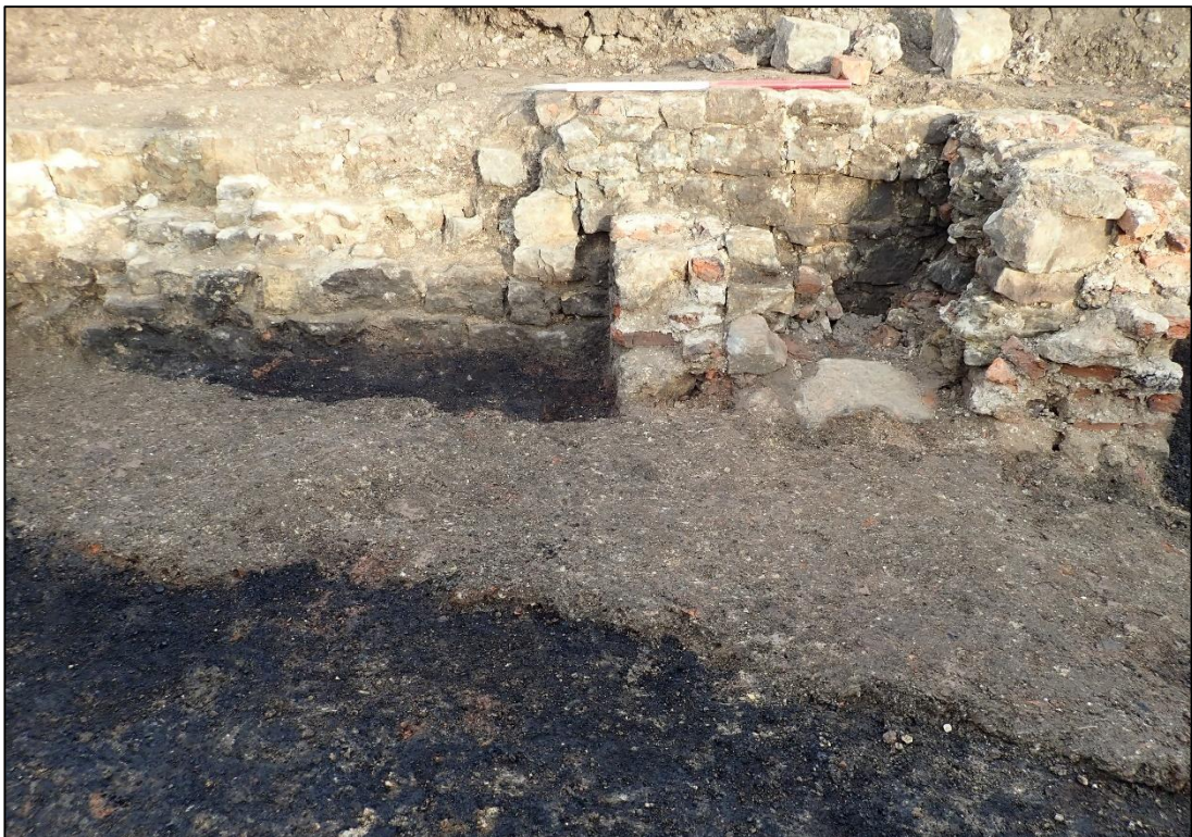
Photograph 26: The damaged support block or buttress [F63] against the north wall of furnace room 57
