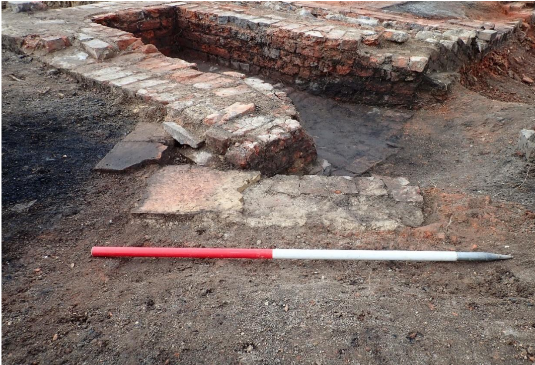
Photograph 81: The smaller hearth between the long walls has evidence of burning on its brick floor [F218]. In the foreground is an unexplained section of wall [F197], set at an angle to the rest of the Newcastle kiln
