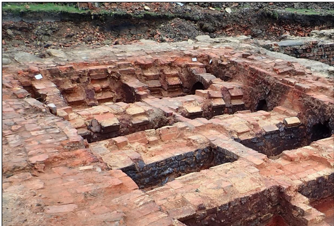
Photograph 18: An oblique view of the east end showing the relationship between furnace arches, the external walls and the 'old man'. The kiln floor was just below the bottom of the white labels on the far wall
