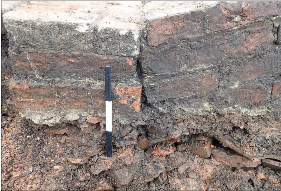
Photograph 77: The north-west kiln lining wall [F201] is not bonded with the sloping brickwork of the chamber. 300mm scale
