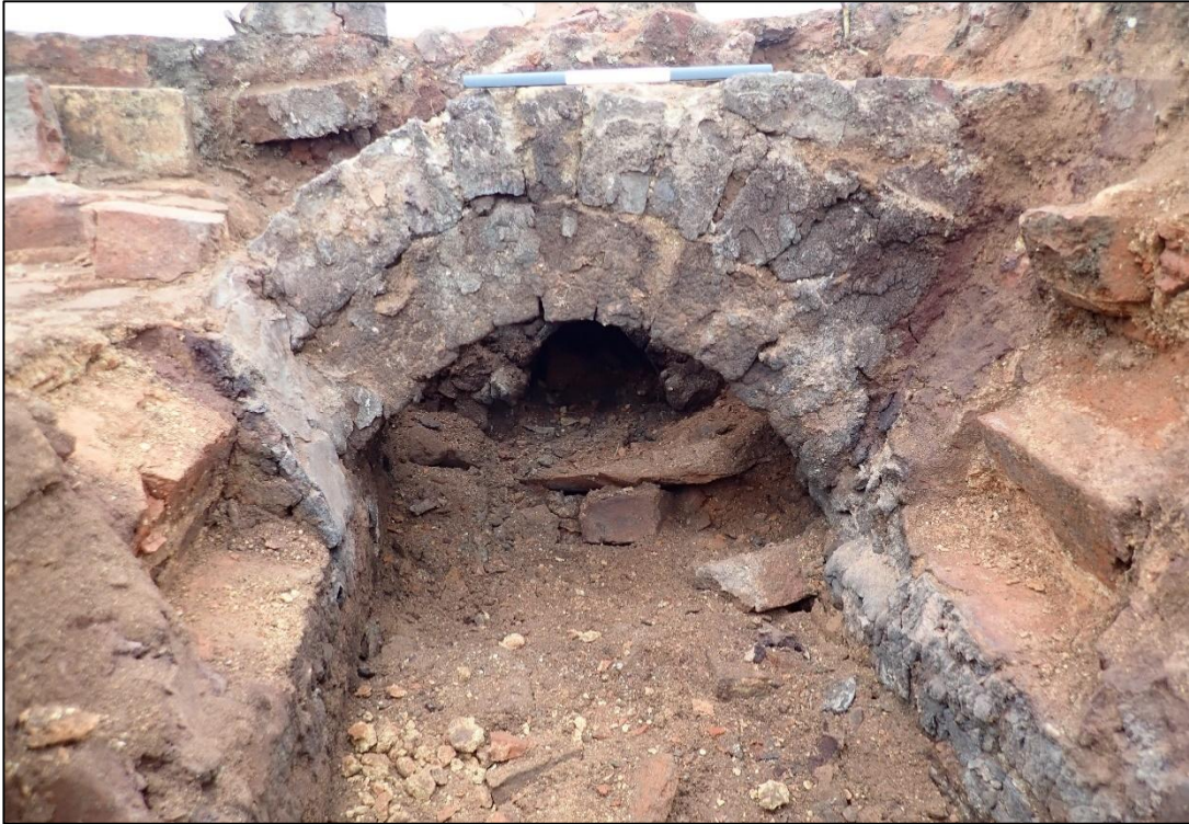
Photograph 19: One of the two surviving furnace arches. The 300mm scale is lying on the old kiln floor. A view looking north
