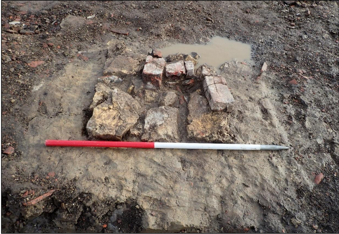
Photograph 67: One of the damaged plinths that were almost all that remained of the unheated drying shed 220
