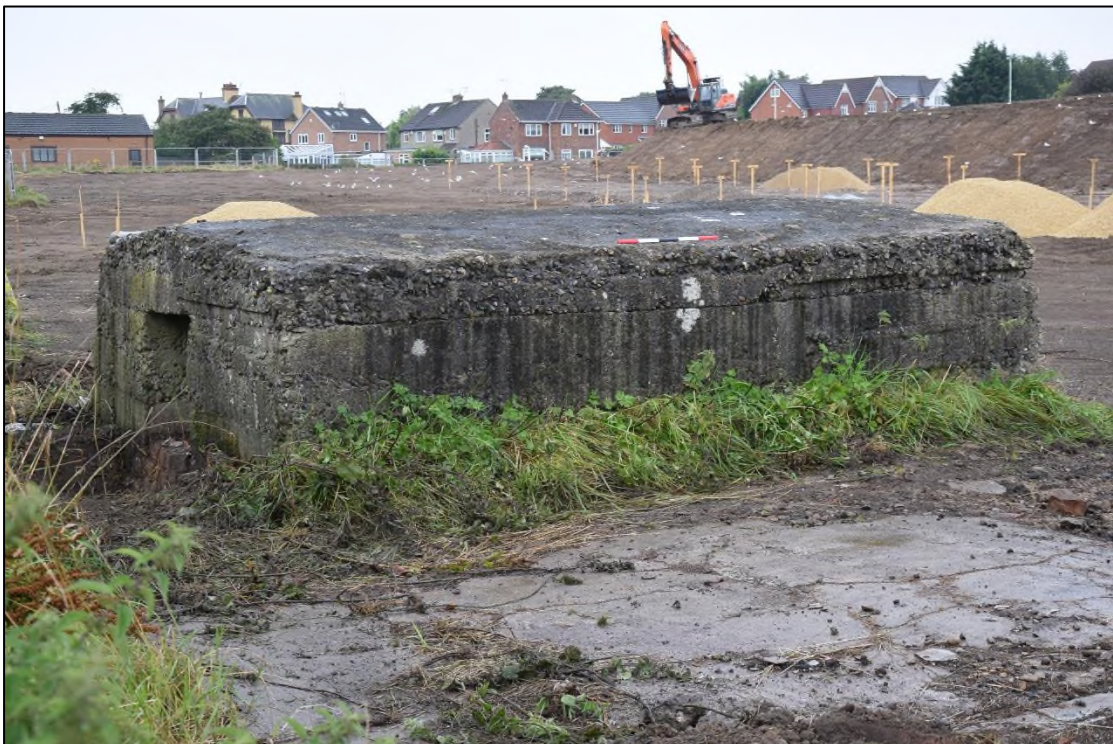
Photograph 4: The north and east faces of the structure, with the door at the left. The concrete in the foreground is the floor of a demolished shed
