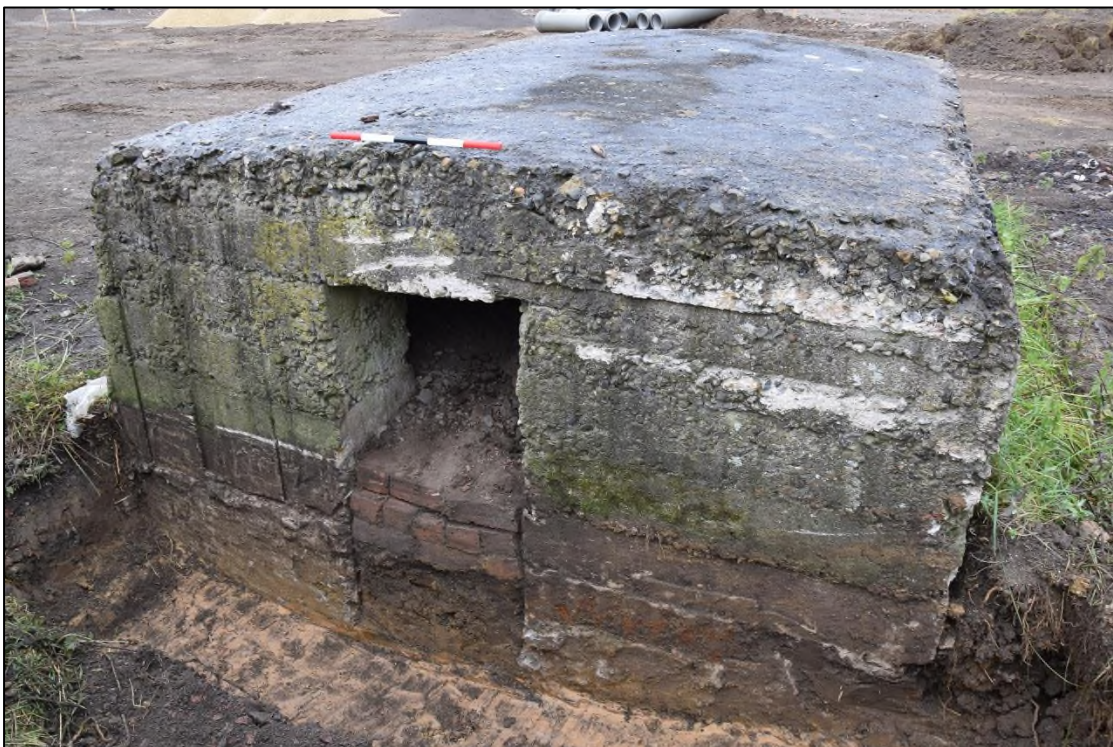
Photograph 14: Clay and bricks have been used to close up the lower half of the door. The walls rest directly on the natural yellow clay subsoil
