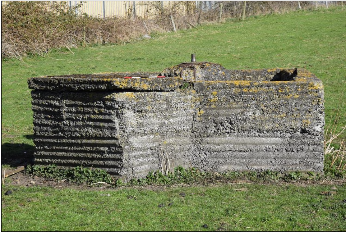
Photograph 7: Similar construction evidence can be seen in this contemporary structure, a Home Guard spigot mortar emplacement at Wolsingham, Co Durham
