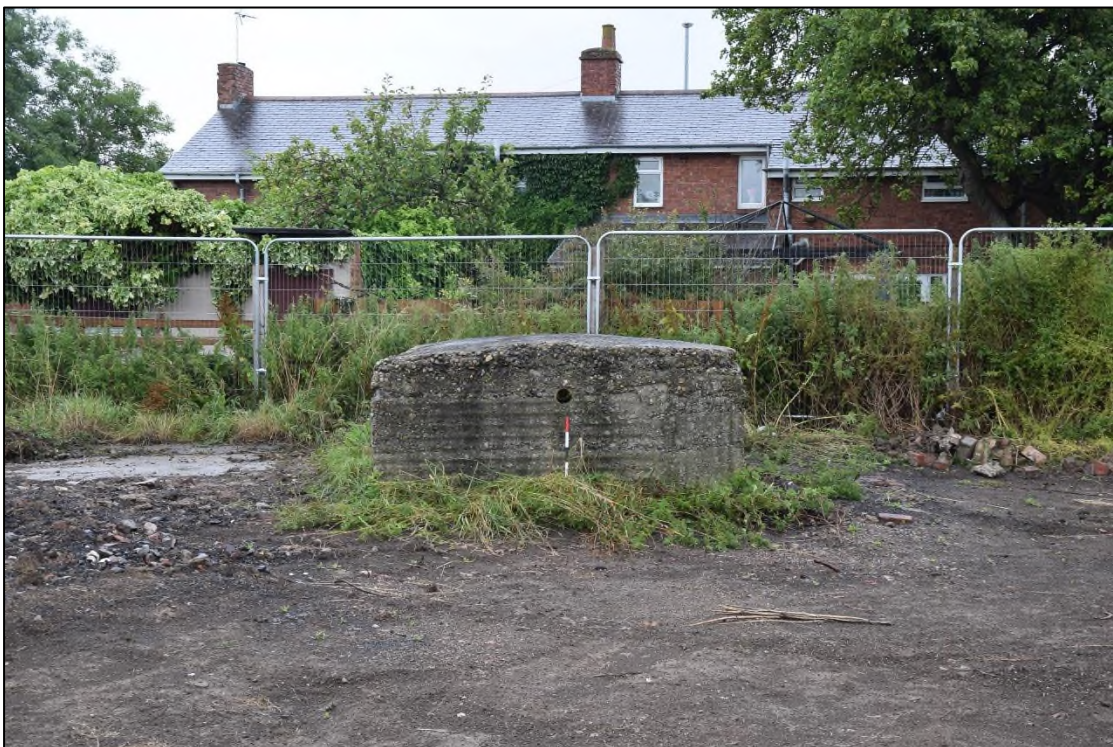
Photograph 2: The shelter and the houses, seen from the west. Note the ventilation pipe and the marks of corrugated iron shuttering in the concrete. The scale is 0.5m long
