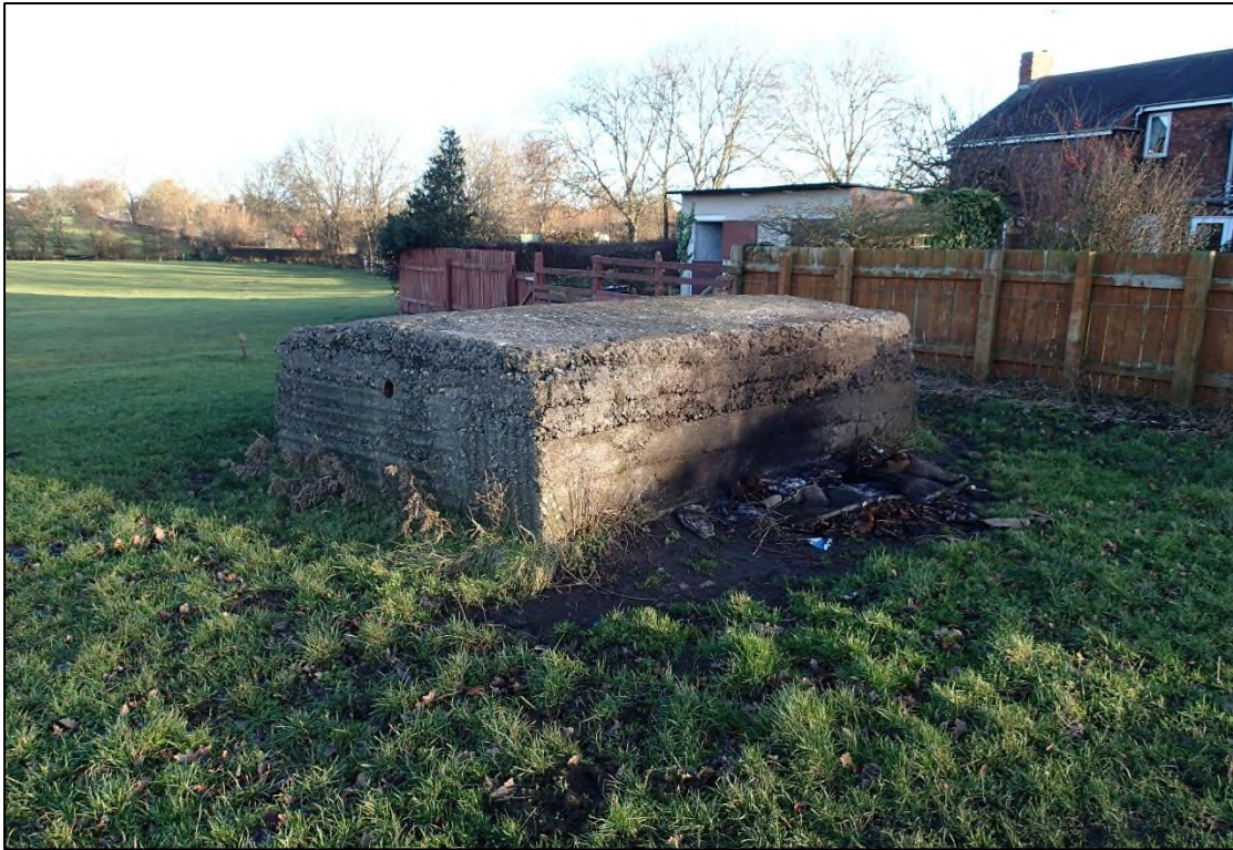
Photograph 1: The air raid shelter before the start of development work, with one of the two smallholding houses in the background. Photo taken by Catrin Jenkins in 2015
