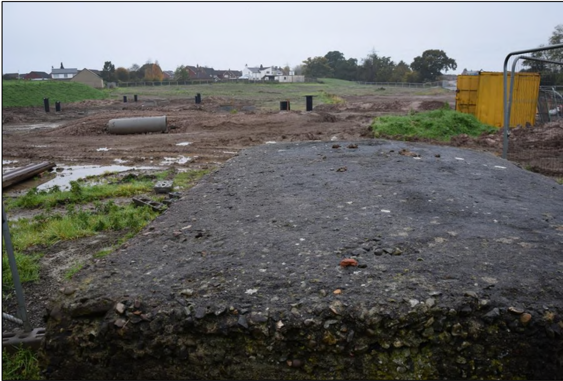
Photograph 3: A view looking west across the roof of the shelter. The white building in the distance is another pair of semi-detached smallholding houses
