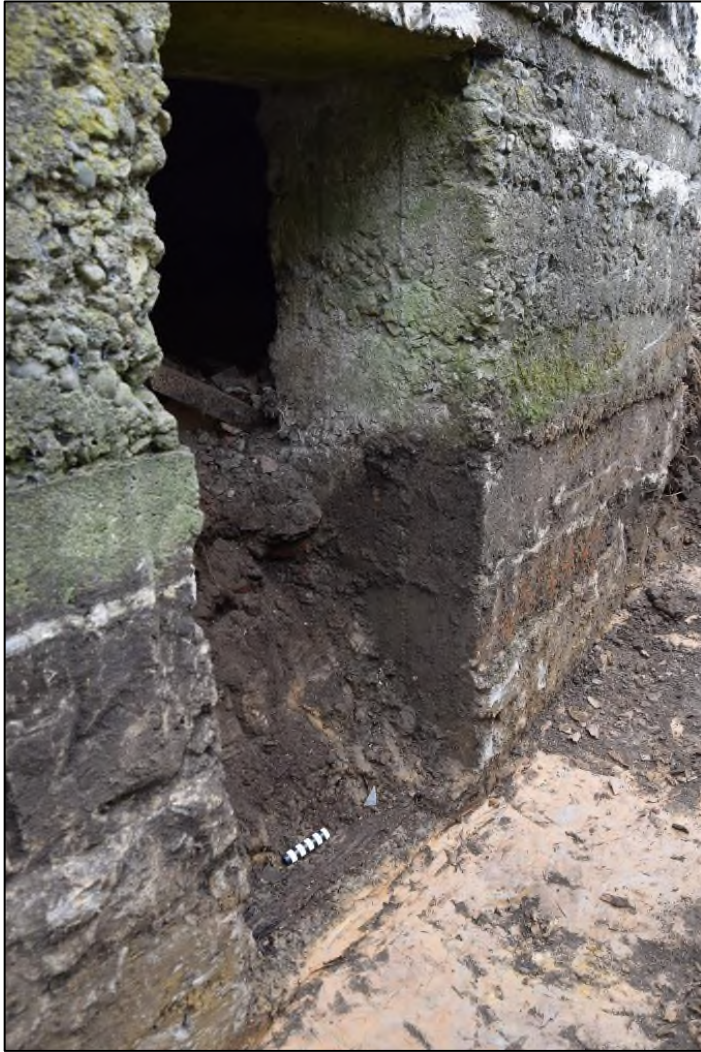
Photograph 15 (left): An oblique view of the door during excavation. Scraps of decayed wood from a door frame are just visible beside the scale. Note the rough construction of the walls and the absence of fixings for the door or its frame
