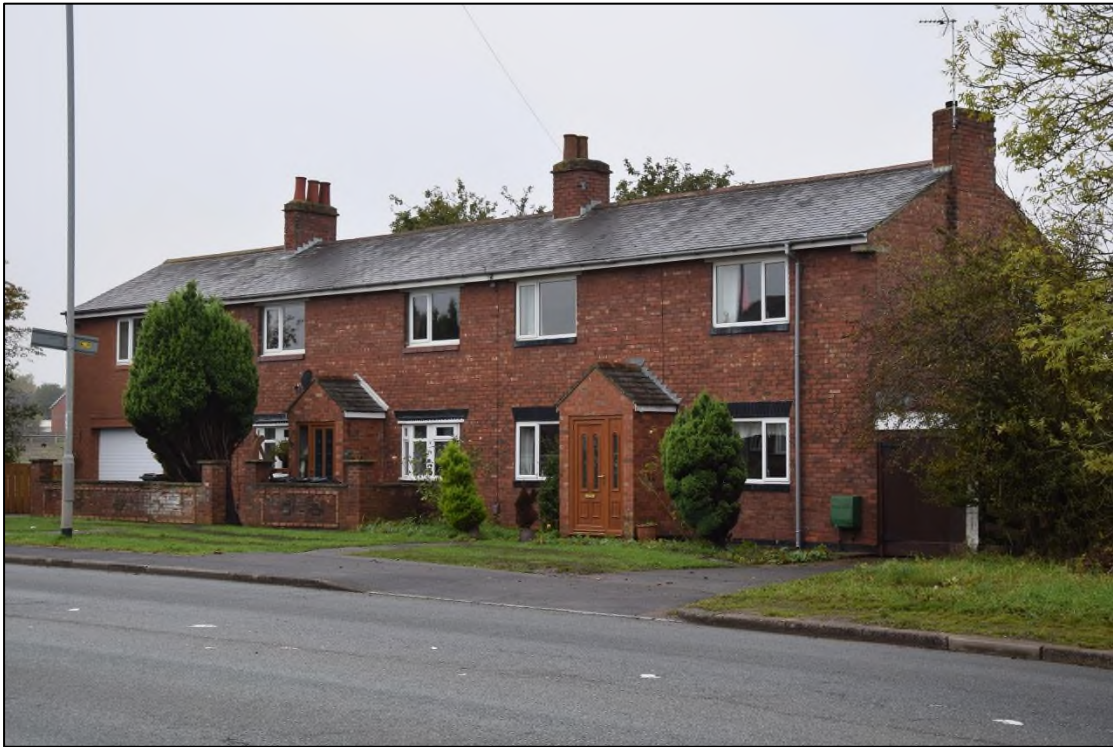
Photograph 17: The two former smallholding houses at the front of the air raid shelter site. The porches and the bay beyond the left-hand chimney are later additions
