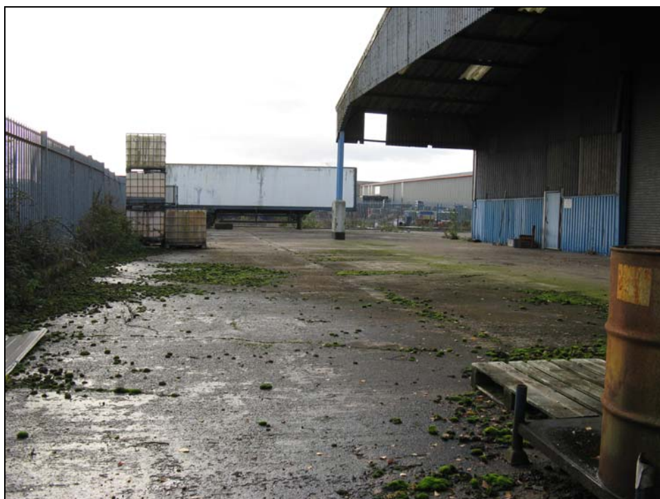
Figure 7 View to south showing warehouse and hard standing
