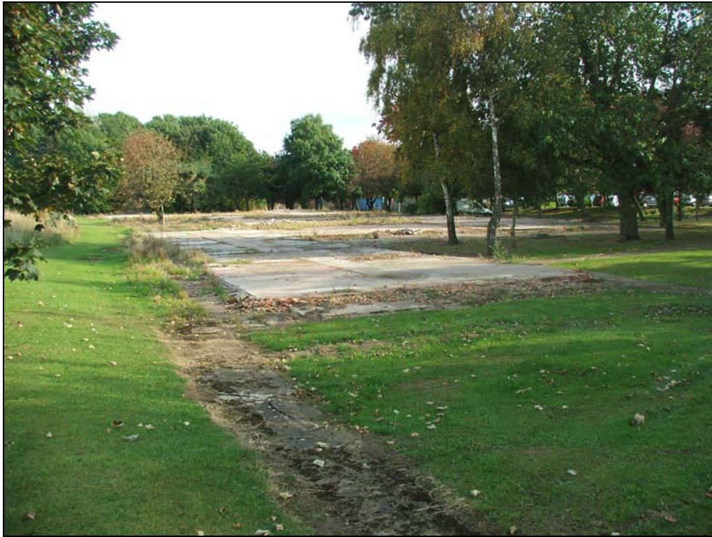
Figure 12 1960's building foundations, looking south-east
