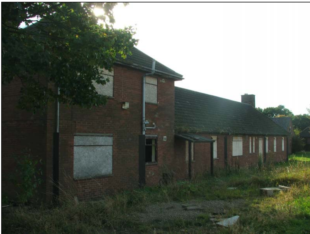
Figure 13 Derelict building, looking south-west
