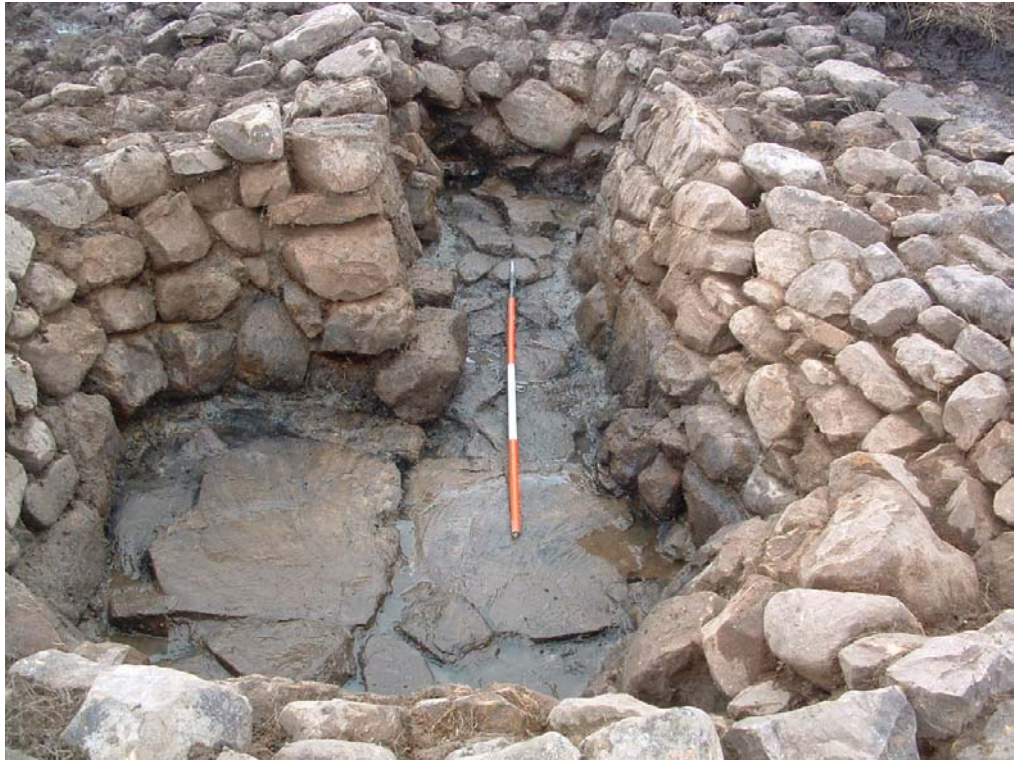
View of corn-drier looking SW; wall repair [F13] can be seen bottom-right.
