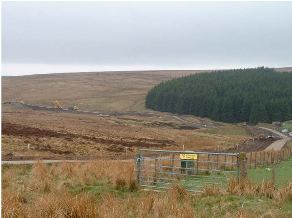
Typical road improvement in progress, Road WW-XX, looking SW
