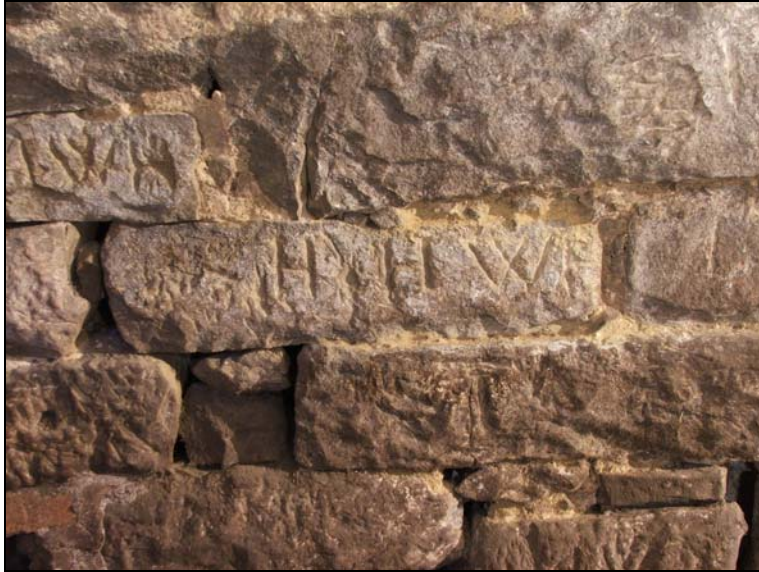
Figure 4 Detail of the lower block, graffito 4
