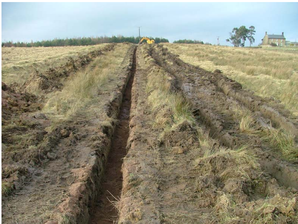
Cable trench 2, looking NNW
