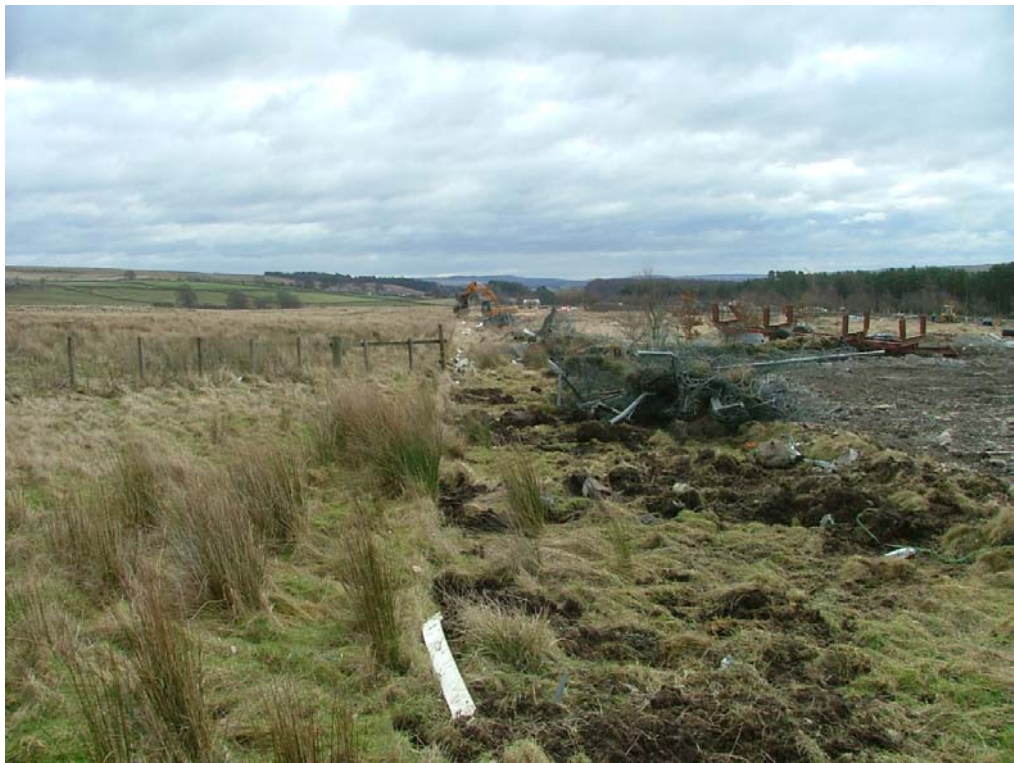
Fence removal operation, looking E
