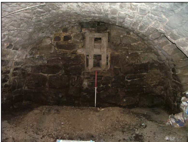
Figure 9 A wider image of the above view, illustrating some of the collapsed roofing vault. 1m scale.
