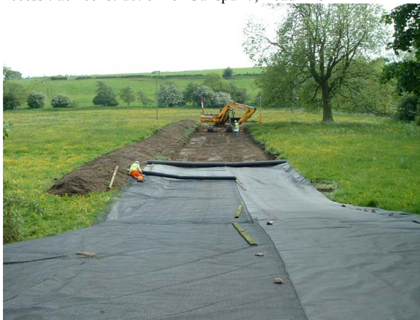
Access track construction for Gunspur 7, Road B-C
