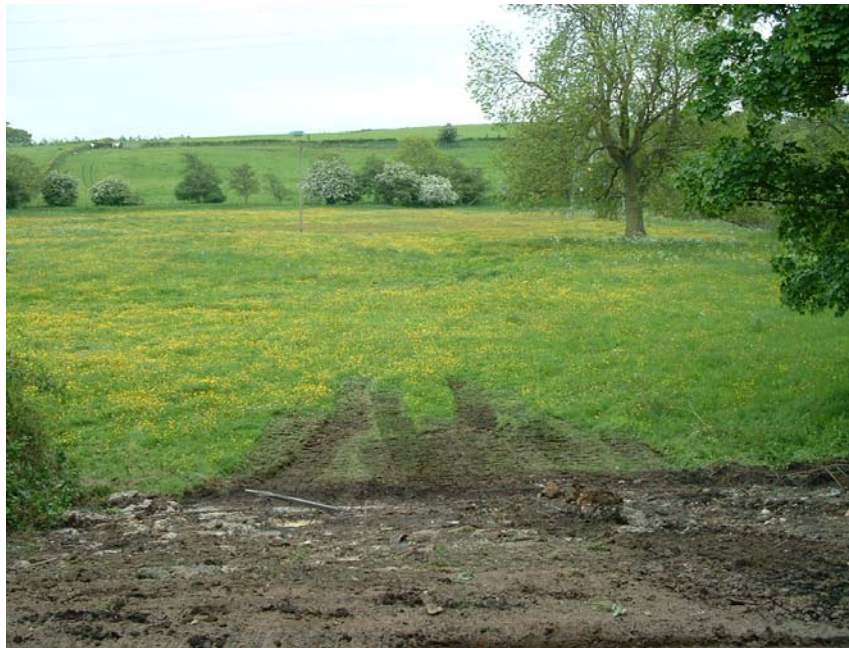
Access track construction for Gunspur 7, Road B-C
