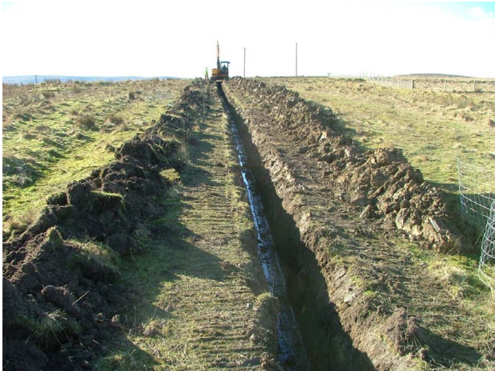
Cable trench 1, looking SW
