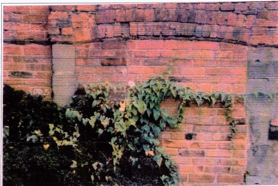
Plate 9 Bricked up fireplace in boundary wall to the rear of 9 St Owens Street
