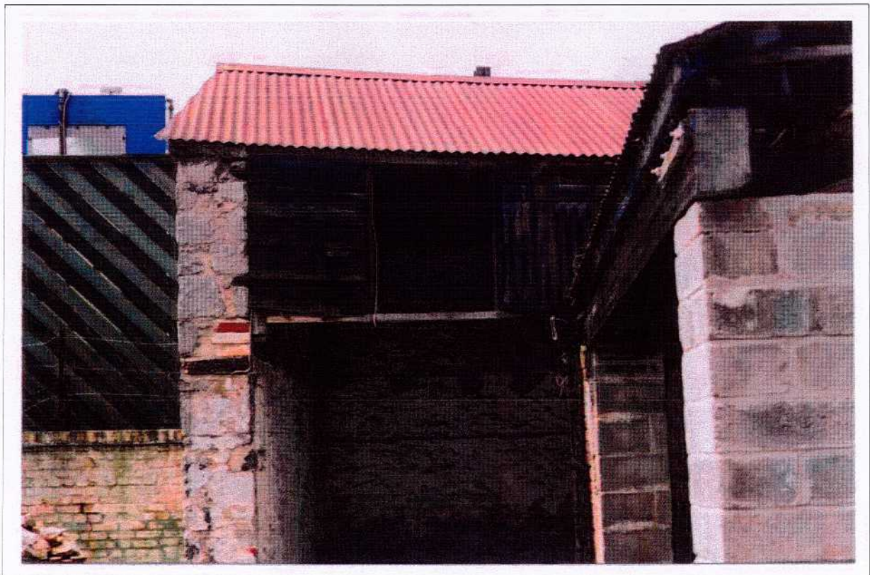
Figure 25. Structure 3, north/south range. Replacement cross-beam and breeze-block pillars to open-fronted section.
