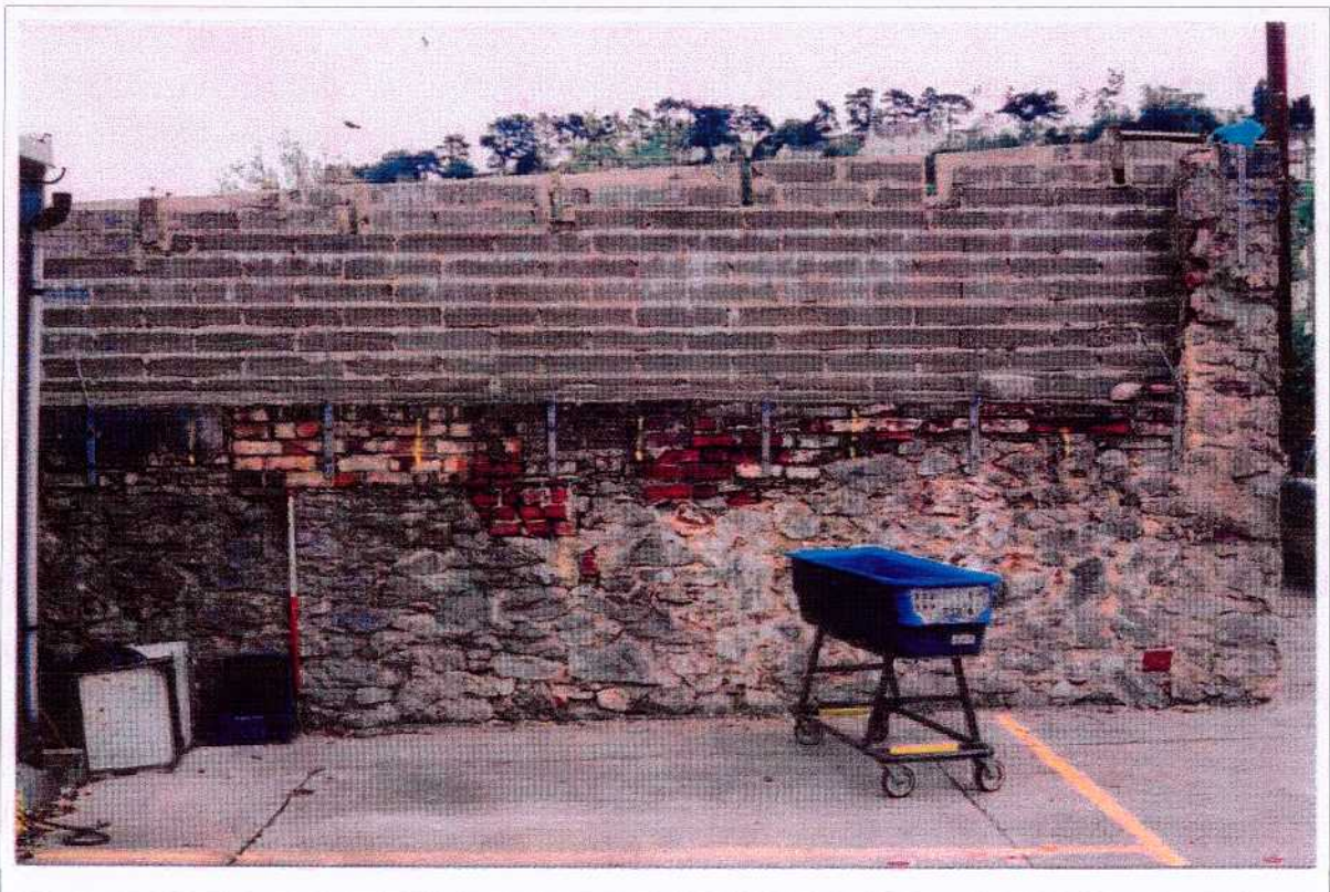
Figure 21. Structure 2. Northern wall, north-facing elevation, showing breeze-block wall of late 20th-century sectional building.
