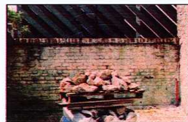
PLATE 15----- L/30/2005-17-8412 BRICK WALL AND RAISED COBBLE AREA
