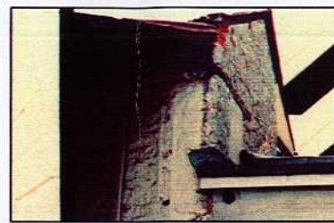
PLATE 5----- L/30/2005-36A-8405 CORNER DETAIL OF BLOCKED WINDOW/DOOR
