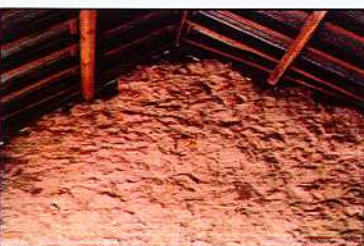
PLATE 18----- L/30/2005-24-8412 DETAIL OF ROOF AND GABLE END
