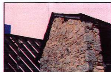
PLATE 14----- L/30/2005-12A-8413 VIEW OF GABLE END
