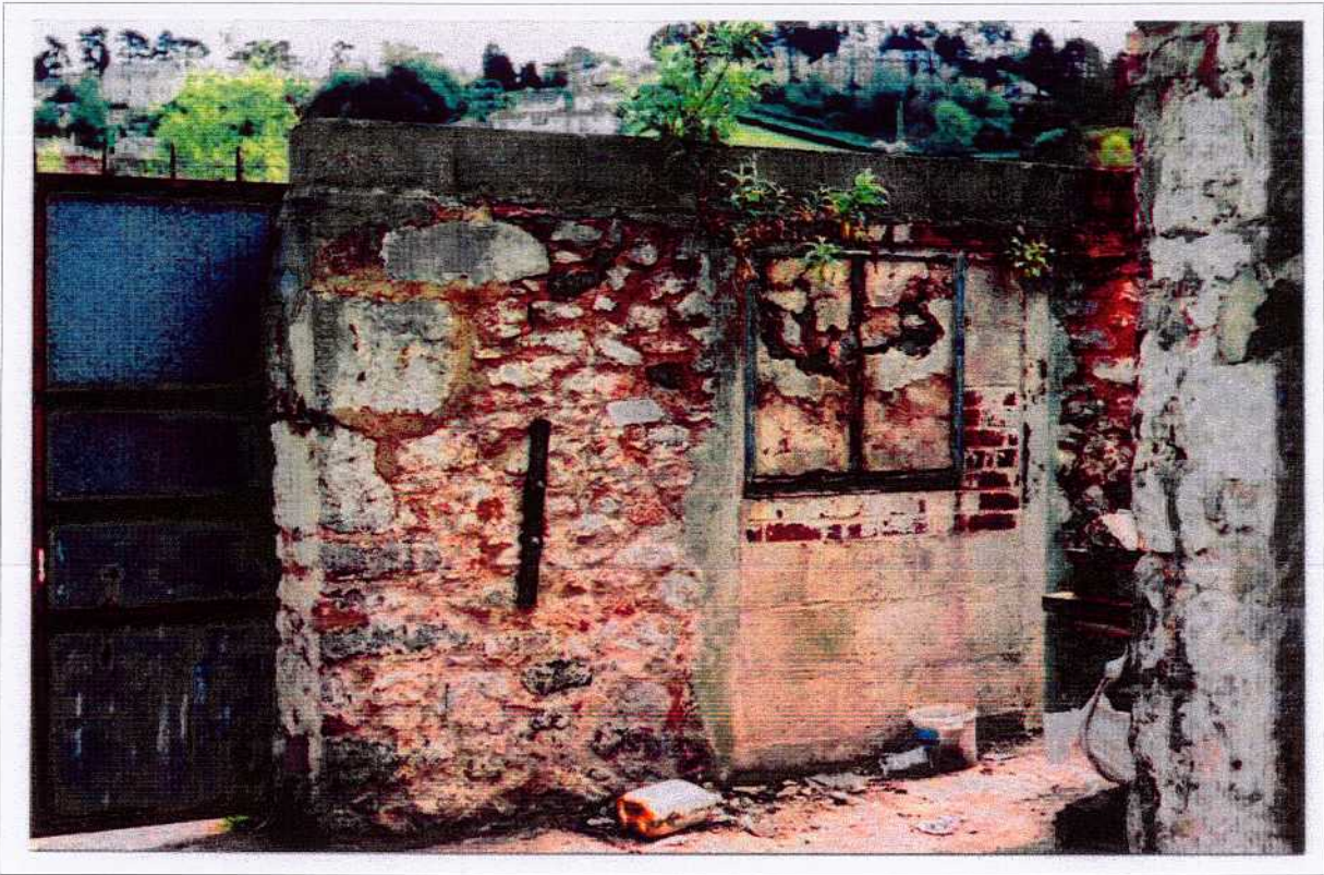
Figure 20. Structure 2. Northern wall, north-facing elevation. Blocked opening.
