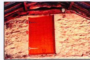
PLATE 7----- L/30/2005-33A-8412 HAYLOFT DOOR AND ROOF DETAILS
