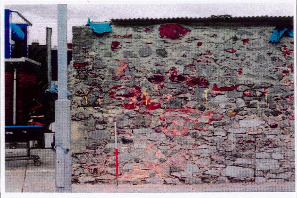
Figure 22. Structure 2. Western wall. West-facing elevation showing different finishes.
