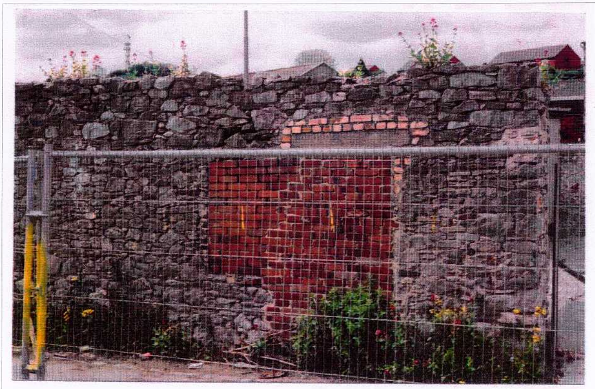
Figure 23. Structure 2. Southern wall, south-facing elevation. Blocked opening.
