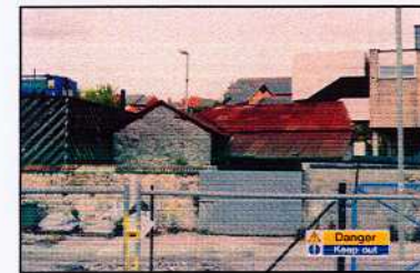
PLATE 10----- L/30/2005-14A-8413 GENERAL VIEW OF BUILDING
