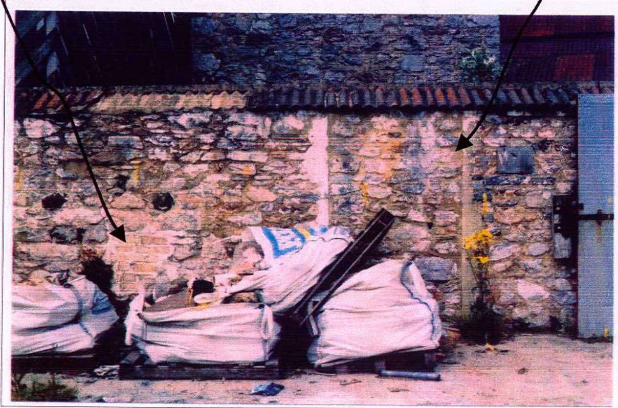
Figure19. Structure 2, north wall. South-facing elevation showing blocking and possible blocked fireplace.
