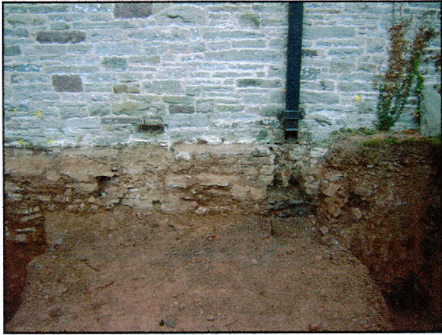
Plate 1 - Foundation levels of north aisle. Camera direction south.
