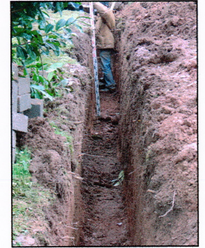
Plate 4 - General shot of service trench. Camera direction NNW.
