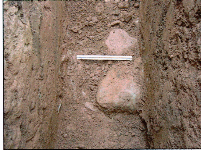
Plate 2 - Possible wall feature (108). Camera direction north.
