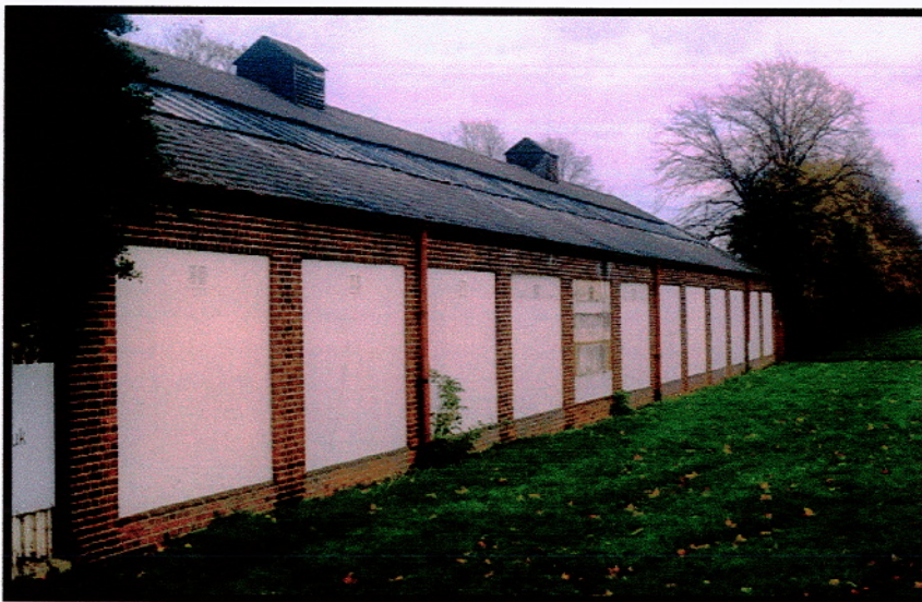
Plate 2 - Rear of Saddling building. NE facing. Photo 109/26
