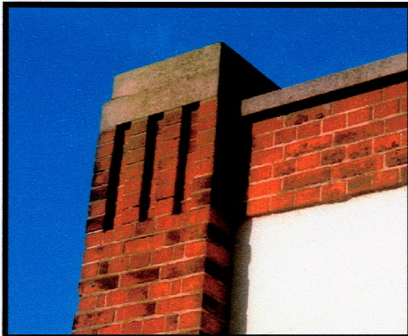
Plate 7 - Accommodation Block. Brick detail on corner pillars of building. 110/34
