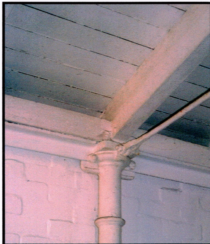
Plate 5 - Veterinary Block interior. Iron roof support. Photo 150/15
