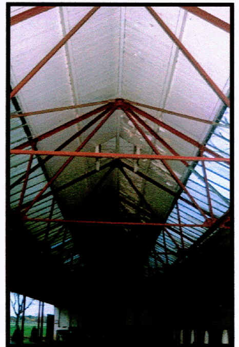
Plate 3 - Detail of Saddling building roof. E facing. Photo 150/29
