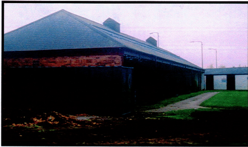
Plate 1 - General view of Saddling building. SW facing. Photo 150/20
