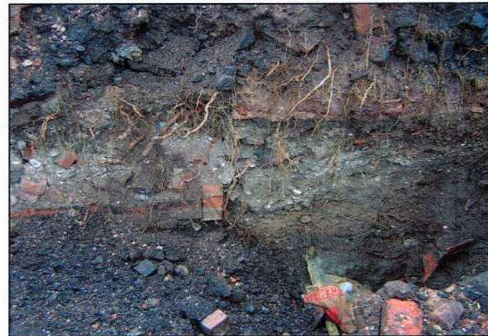
Plate 10. Brick wall exposed during excavation of foundations.
