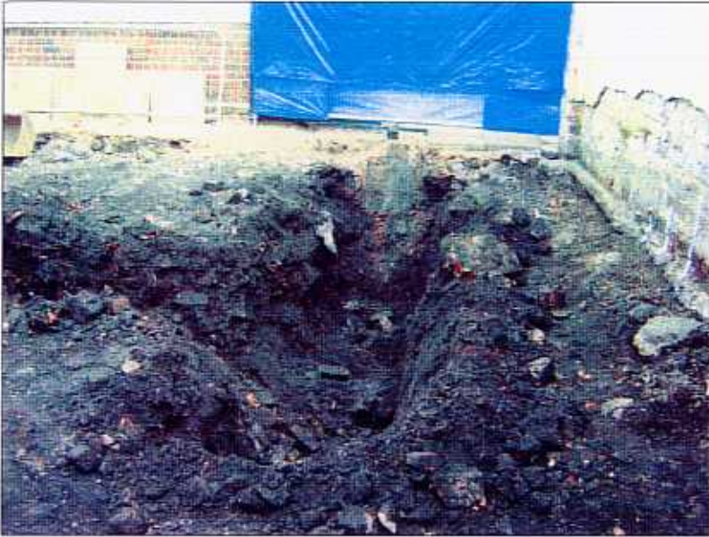
Plate 1 General view of trench 1, facing North.
