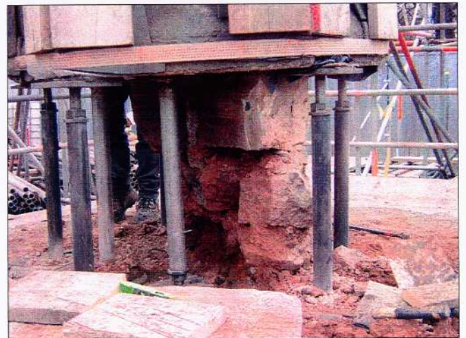
Plate 4, After partial removal of the key stone, exposing the iron tie rod and its securing lead/pebble plug.
