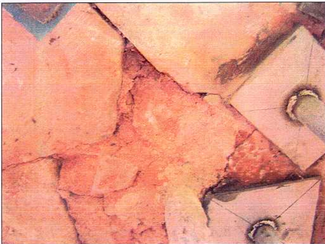
Plate 3, Construction of hexagonal pediment, viewed from below, lead plug encasing iron rod at the bottom of the picture.
