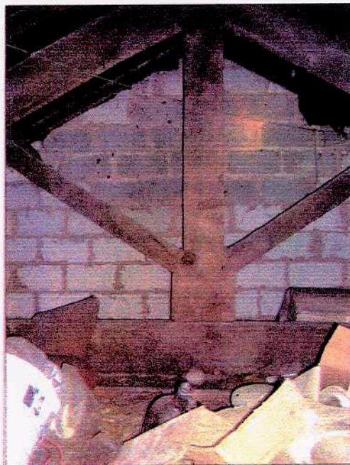
Figure 12. Internal roof structure
