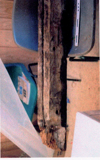
Plate 13, Moulded timber re-used as a lintel from the doorway between Rooms 1 and 2 (showing the good side).
