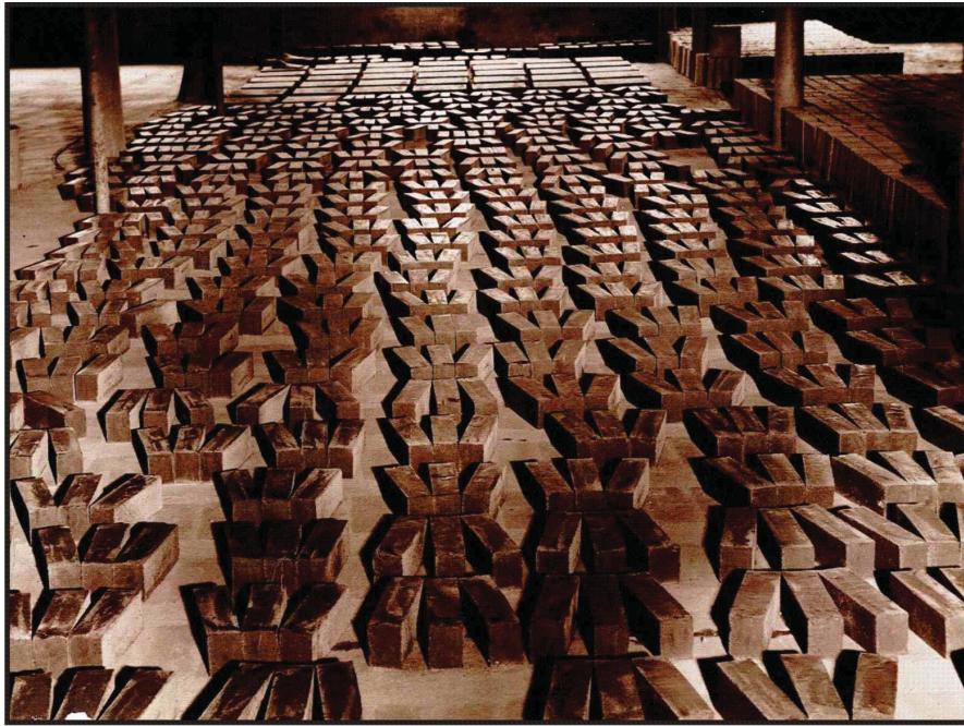
Plate 8. Bricks drying on hypocaust floor
