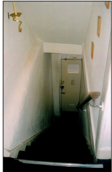
c. Inserted stairwell
