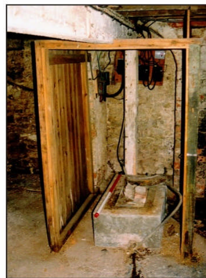
e. Gas boiler mounting
