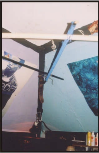
c. Roof beams above no. 13 Union Street
