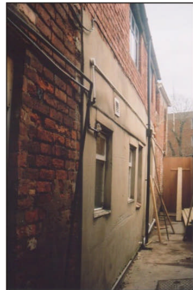
d. Original access to Bastion house
