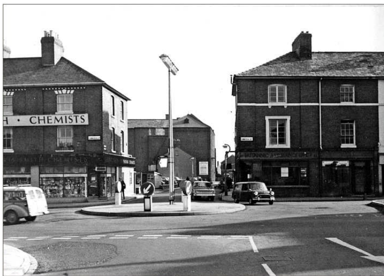
b. Leonard Johnson's urban landscape (Pre 1967). Looking SE along Bath St, Old Mill in background. Graham Roberts Survey - Hereford City Council.
