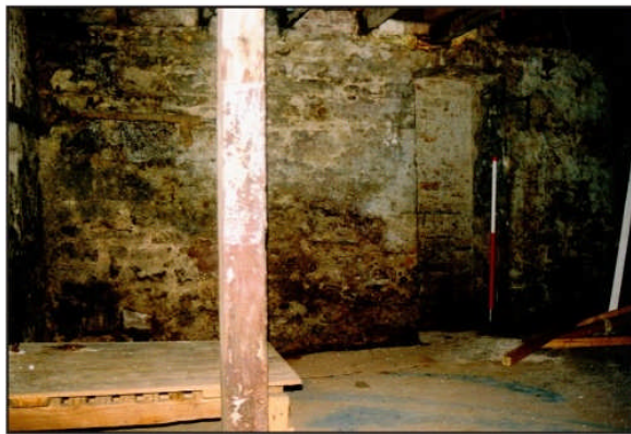
c. Niche in cellar wall
