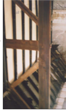
Plate 17. The truss in the granary, bolted from below, the raking struts lean out from the tie beam, not the king post as with the cottage truss.
