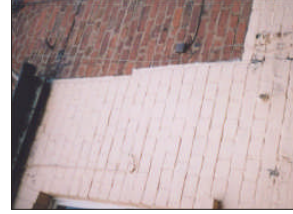
Plate 3. Construction break between the cottage and No 13 (North wall).
