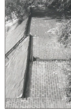
Plate 4. Construction break (to the left) at the west end of the cottage and the east end of number 13, South Street (South wall).
