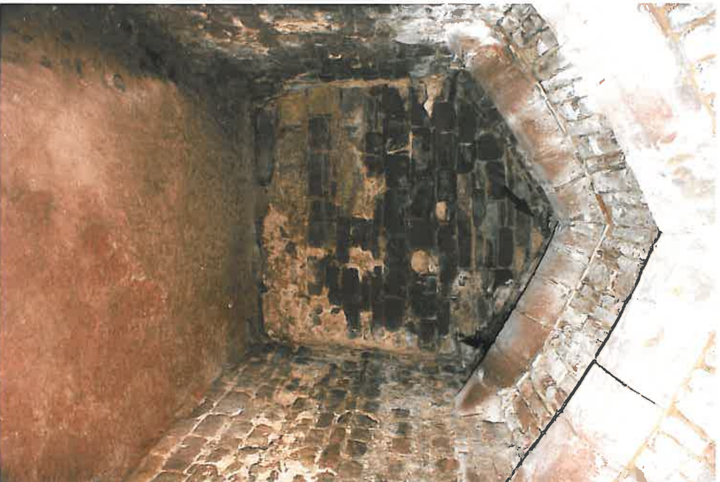
Plate 3. Hole at the top of rear dungeon wall and red sandstone bedrock surface
