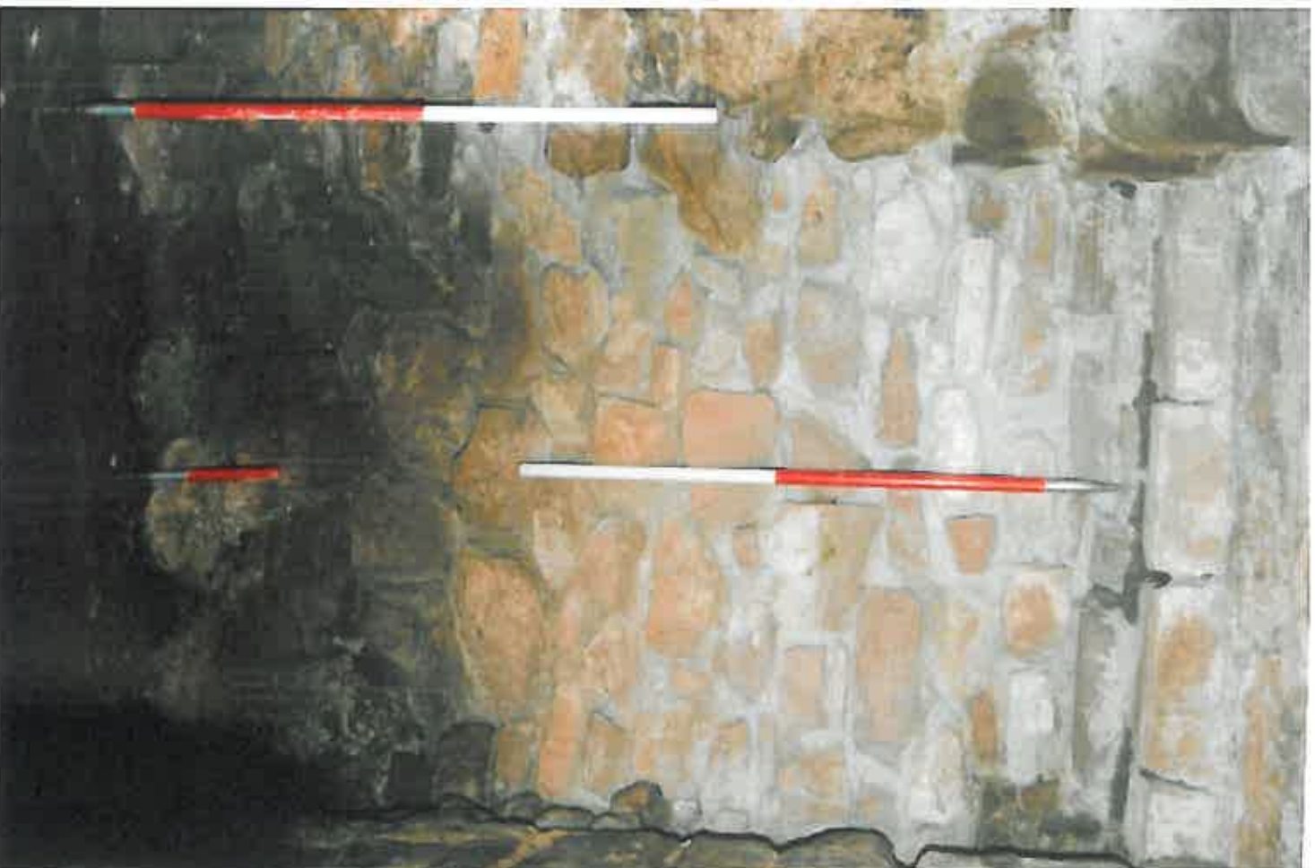
Plate 5. The resealed opening on the northwest wall leading to the keep
