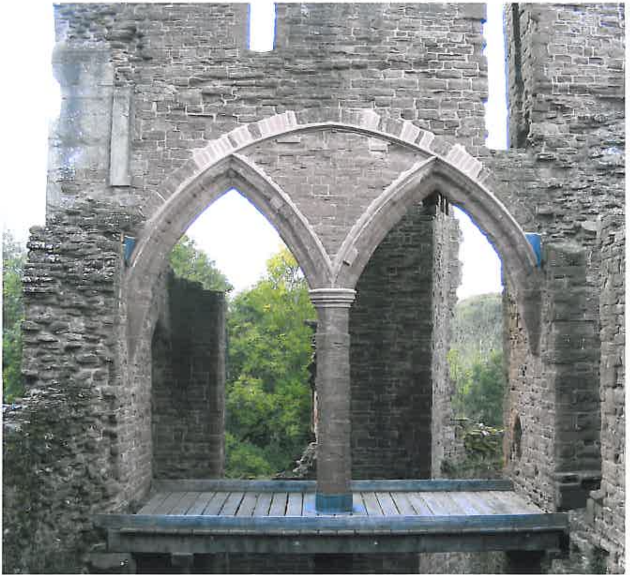
Plate 7. The Solar Arch after remedial works
