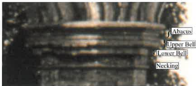
Plate 2. Enlargement of the capital from the c. 1868 photograph with added description of the four moulded components. The effects of erosion are clearly visible on the upper and lower Bell. (Photograph courtesy of George Eastman House. Ex collection A E Marshall)
