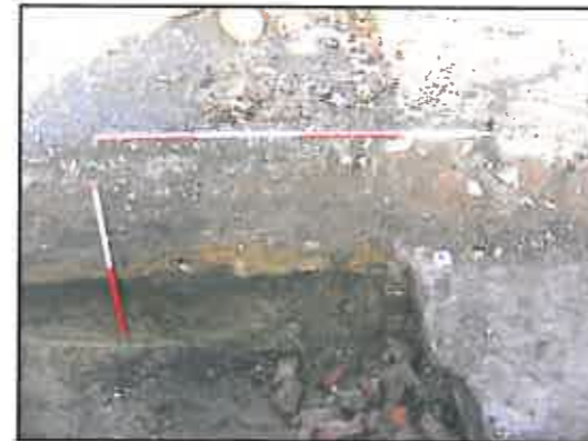
Plate 7, Trench 2, facing north, shows the remains of the (collapsed) wall [206], concrete [208] and adjacent stratified deposits.
