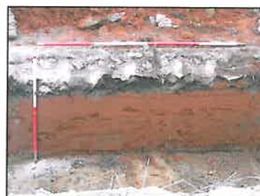
Plate 17, Trench 5, facing south, shows thickness of the concrete, the scalpin sub base and the underlying red sand that was directly overlying natural clay.
