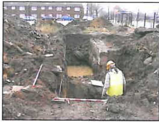
Plate 1, Trench 1, facing south, note the large concrete pile along the western edge of the trench.
