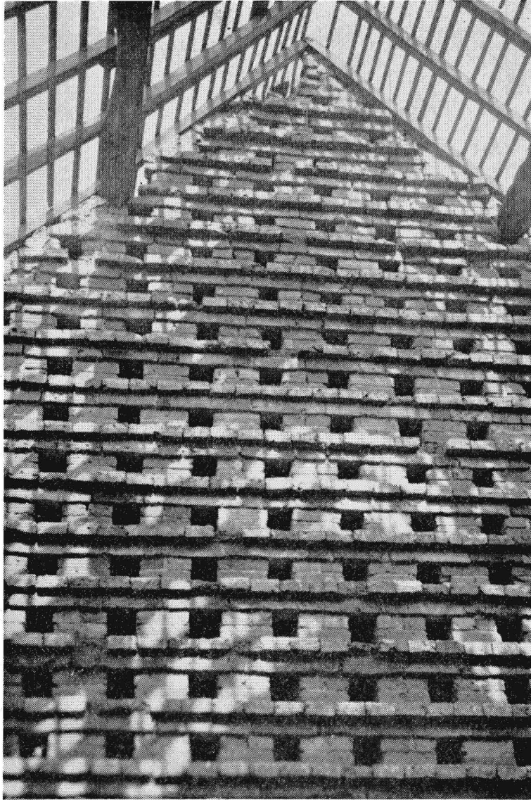
Dovecote at Court Farm, Houghton-on-the-Hill
