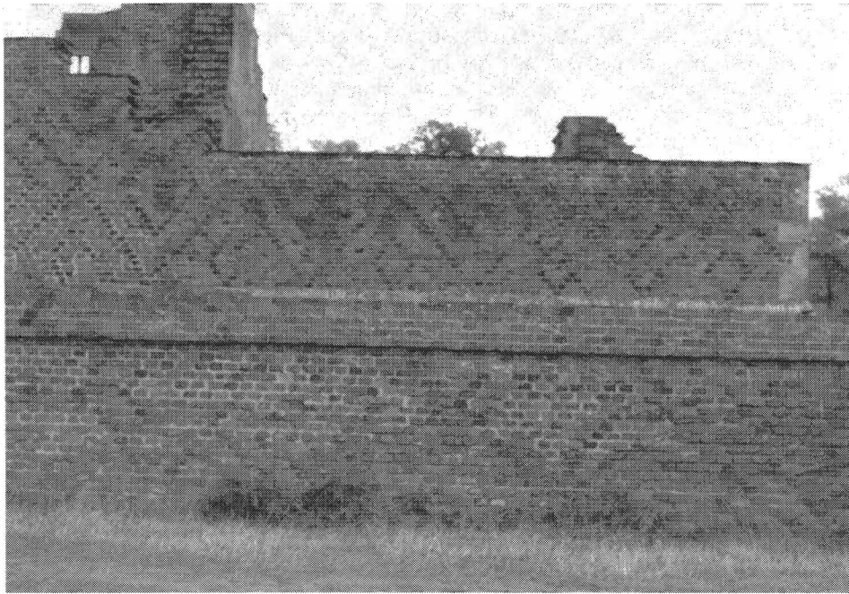
2. Diaper work on Bradgate House, Bradgate Park.
