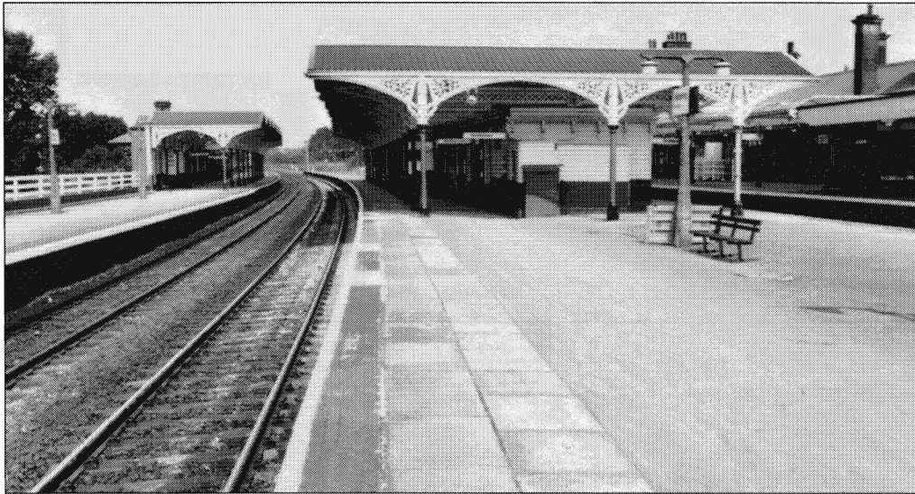
5. And this view of Kettering shows how the ironwork on three of the four platforms is identical to that on Wellingborough's northbound platform. Also to be seen is the quite different new work on the extreme right-hand side (the architect for this being Charles Trubshaw, who was also responsible for Leicester London Road station). (author's collection)
