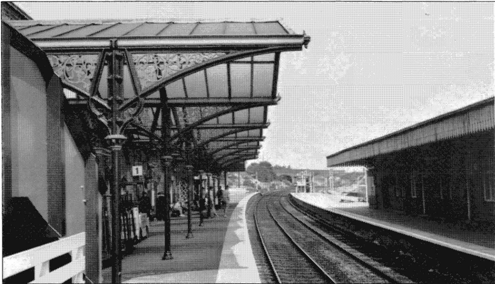
4. This view of Wellingborough (looking north) shows the original ironwork of the canopy on the down (northbound) platform and the much newer work on the island platform serving the up line. (author's collection)
