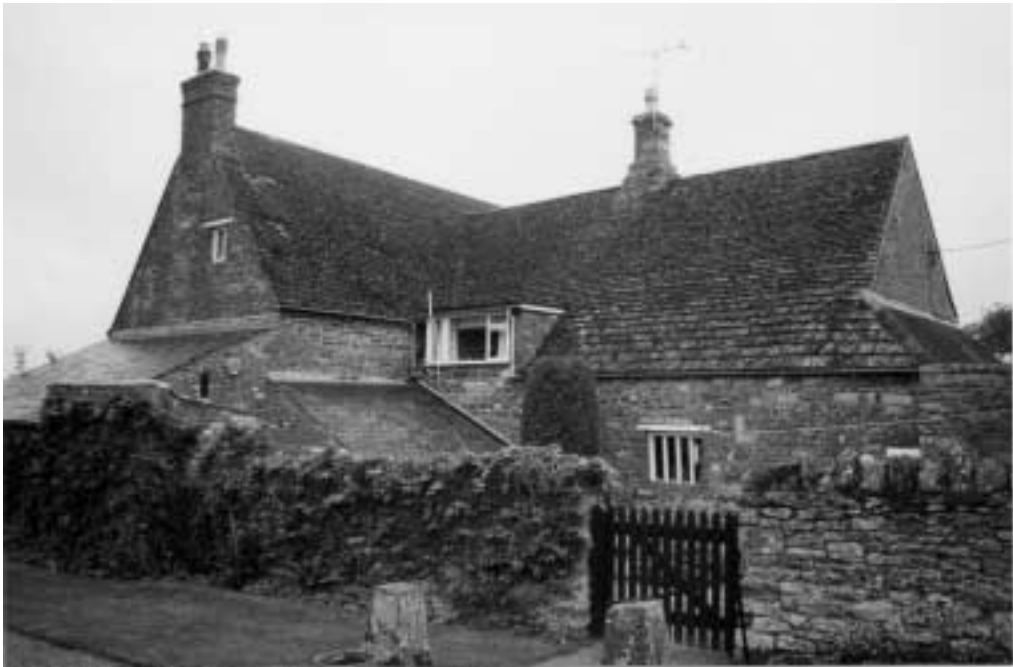
5. View of cross wing and hall from north-east
