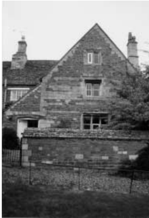
15. West gable of cross wing, with deeply moulded solar window
