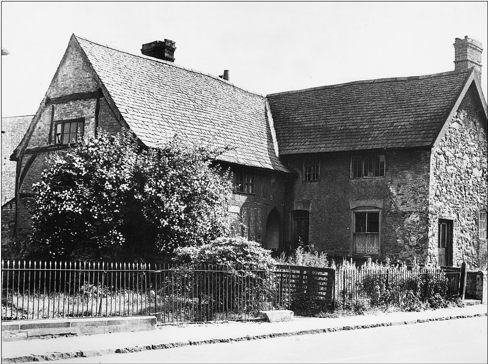
8. The 'Old Ship' prior to demolition in 1955 (LLRRO copyright).
