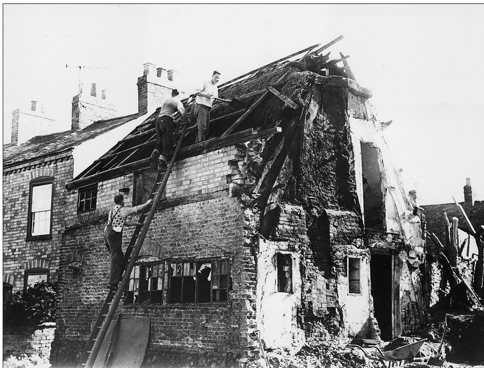
10. Cruck revealed by demolition of cottages during extension of Crown Inn in 1960 (LLRRO).
