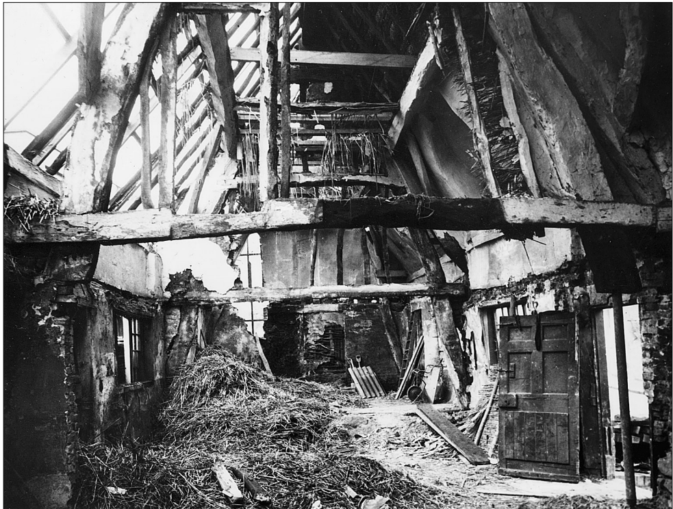
9. Cruck frame at 10–12 Bradgate Road during demolition in 1957 (LLRRO copyright).
