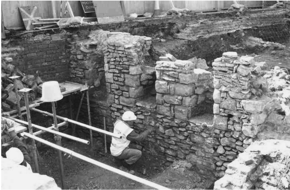
Fig. 9. The undercroft: western internal wall elevation.
