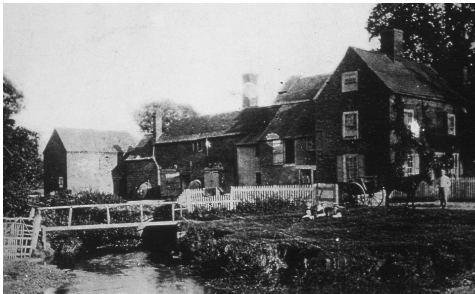
Fig. 9. Photograph of the nineteenth-century mill buildings, looking south. Note the brick culvert and the two millstones either side of the door of the central building. Date c. 1892 (after Ashton 1977)
