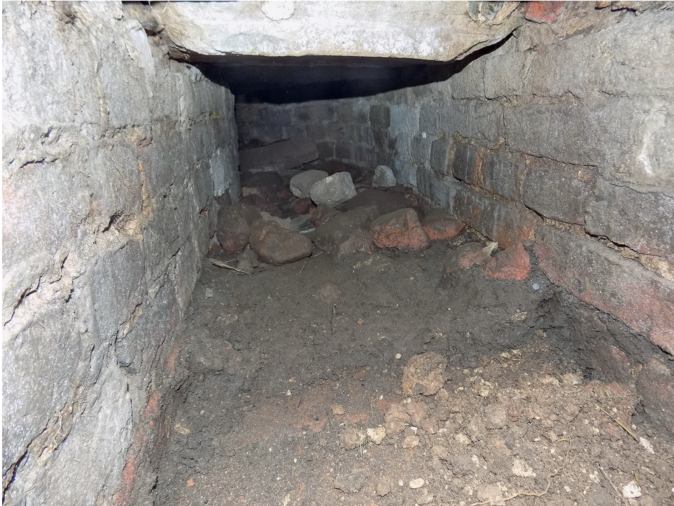
Fig. 19. A view inside the drain.
