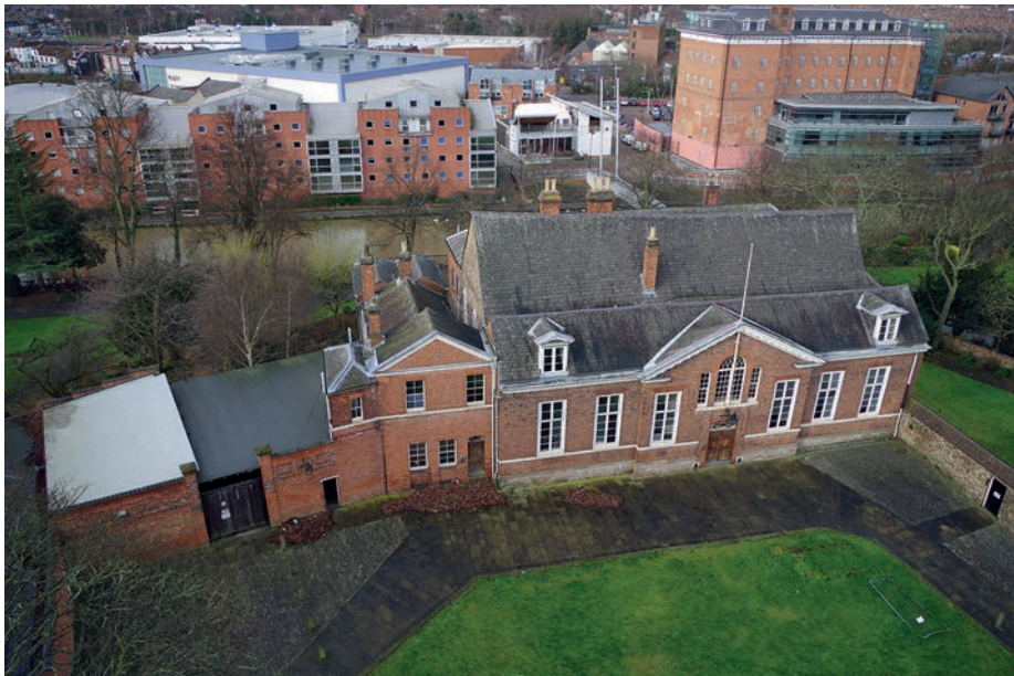
Fig. 2. Leicester Castle Hall from the east, with the new façade of c.1695. John of Gaunt's Cellar lies under the flat-roofed buildings to the left. Image by N Finn.
