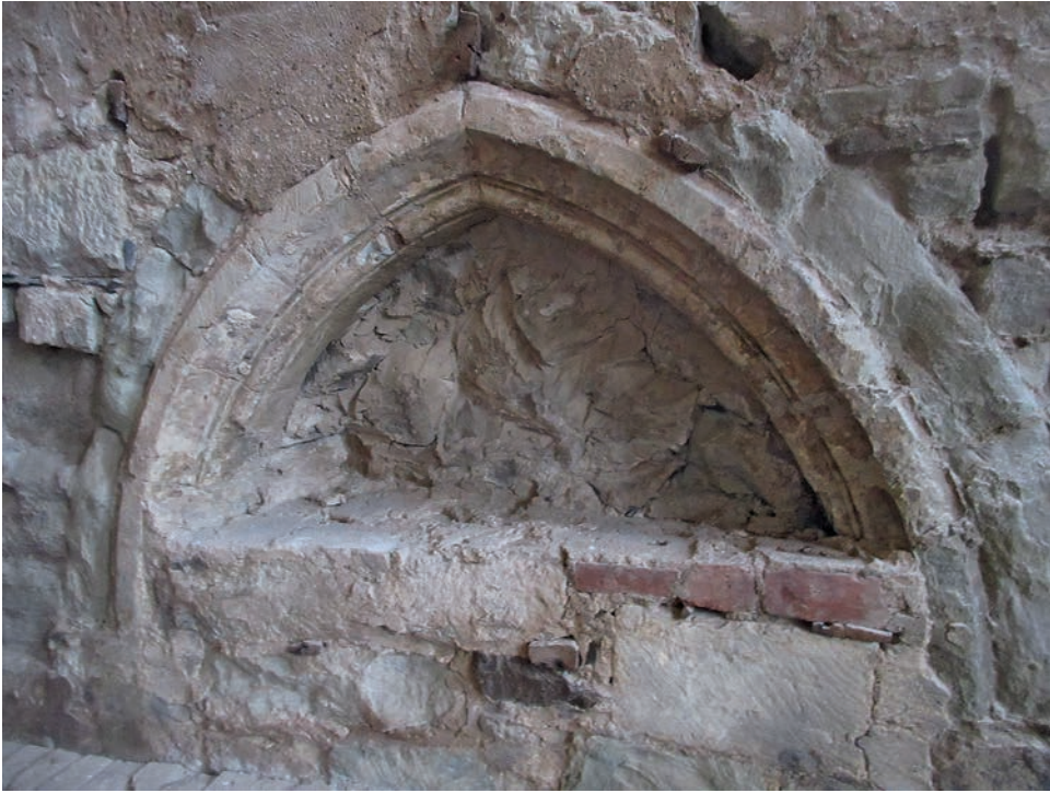
Fig. 21. One of the blocked doorways in the north gable, as uncovered in 2016. Image N Hill.
