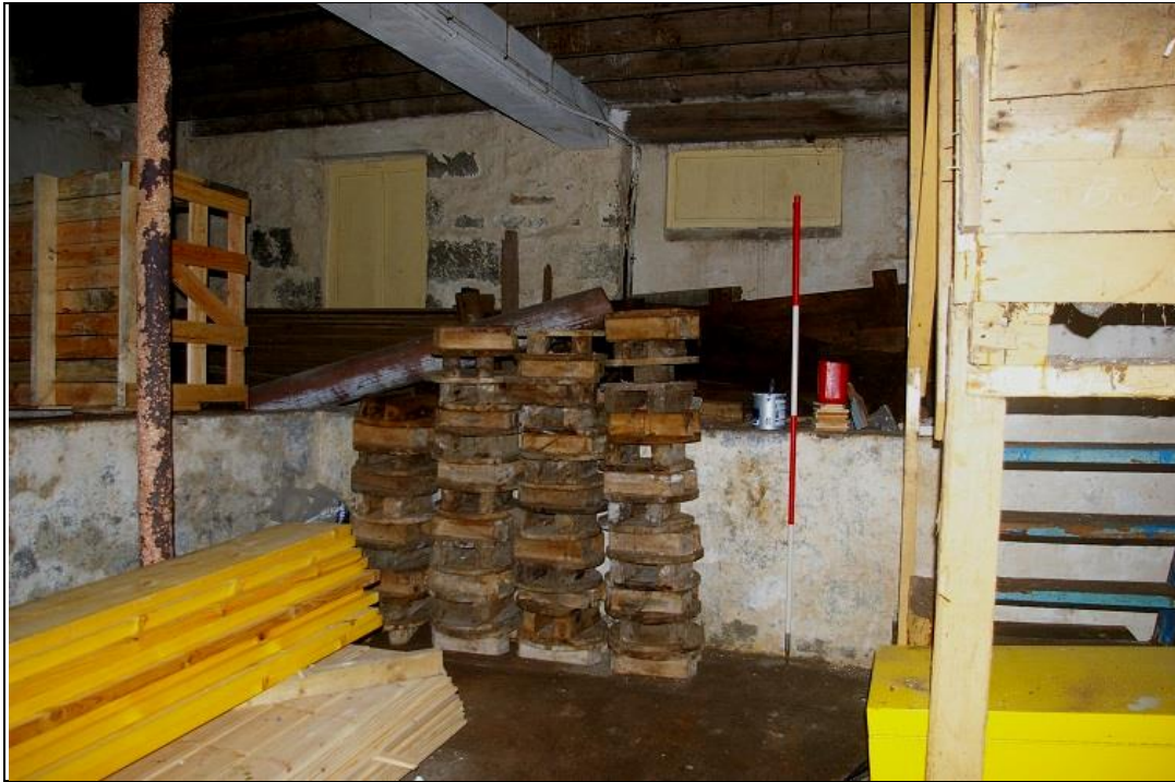
13. THE GROUND FLOOR OF THE BUILDING IS NOT FITTED OUT WITH CONCRETE FISH PITS TO THE SOUTH-WEST AND NORTH-WEST WALLS, AS WELL AS THE SOUTH-EAST FULL HEIGHT PARTITION, EVIDENCING A LATER CONVERSION TO A FISH CELLARS (2M SCALE); FROM THE EAST.
