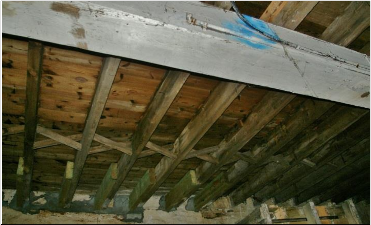
17. THE CEILING IN B1A, WITH RAFTERS BRACED BY X-NOGGIN SUPPORTS.
