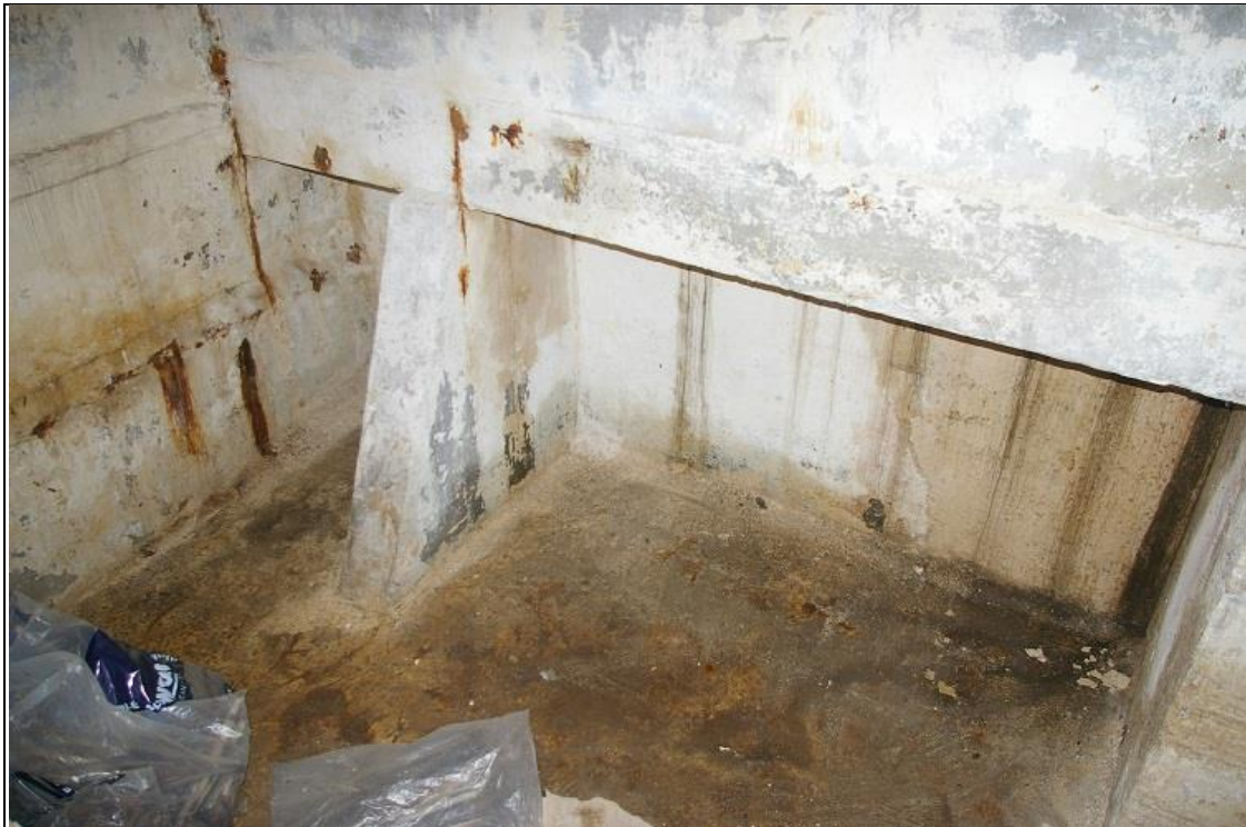
14. THE DEEP PIT TO THE SOUTH-EAST ENCLOSED BY FULL HEIGHT CONCRETE PARTITIONS; FROM THE WEST.
