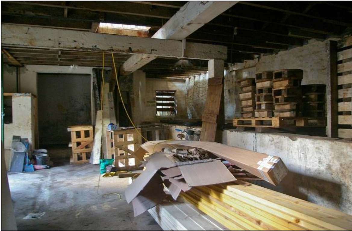
FIGURE 4: THE GROUND FLOOR OF THE BUILDING WITH THE CONCRETE PITS FOR FISH ALONG THE SOUTH-WEST WALL; FROM THE NORTH.
