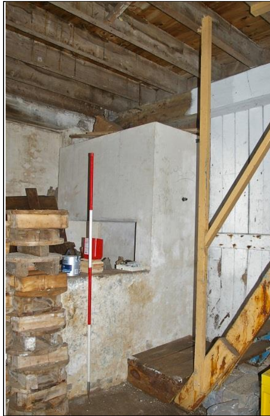
15. THE STAIRCASE AND BOARDED PARTITION, WITH CONCRETE FISH PITS AND TANK (2M SCALE); FROM THE SOUTH.
