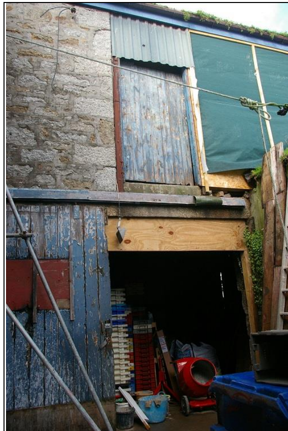
FIGURE 10: BUILDING 1B - ADJACENT AND ADJOINING B1A; FROM THE SOUTH-EAST.
