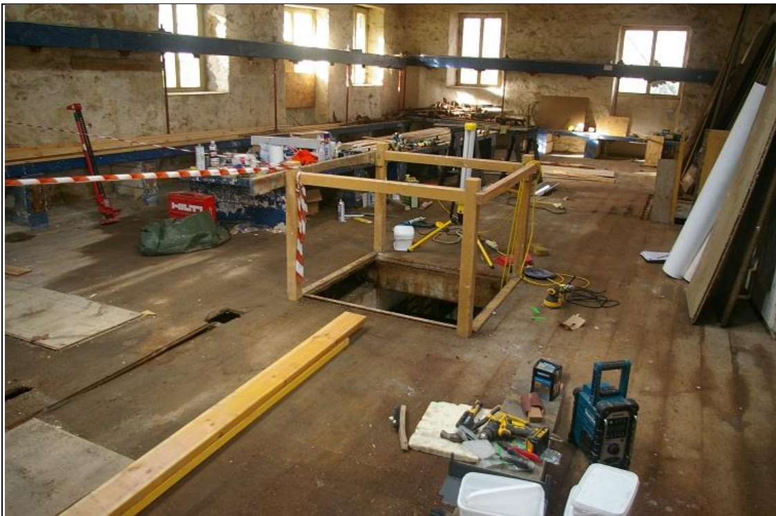
24. THE BOARDED FLOOR OF B1A, WITH CENTRAL HATCH; FROM THE EAST.
