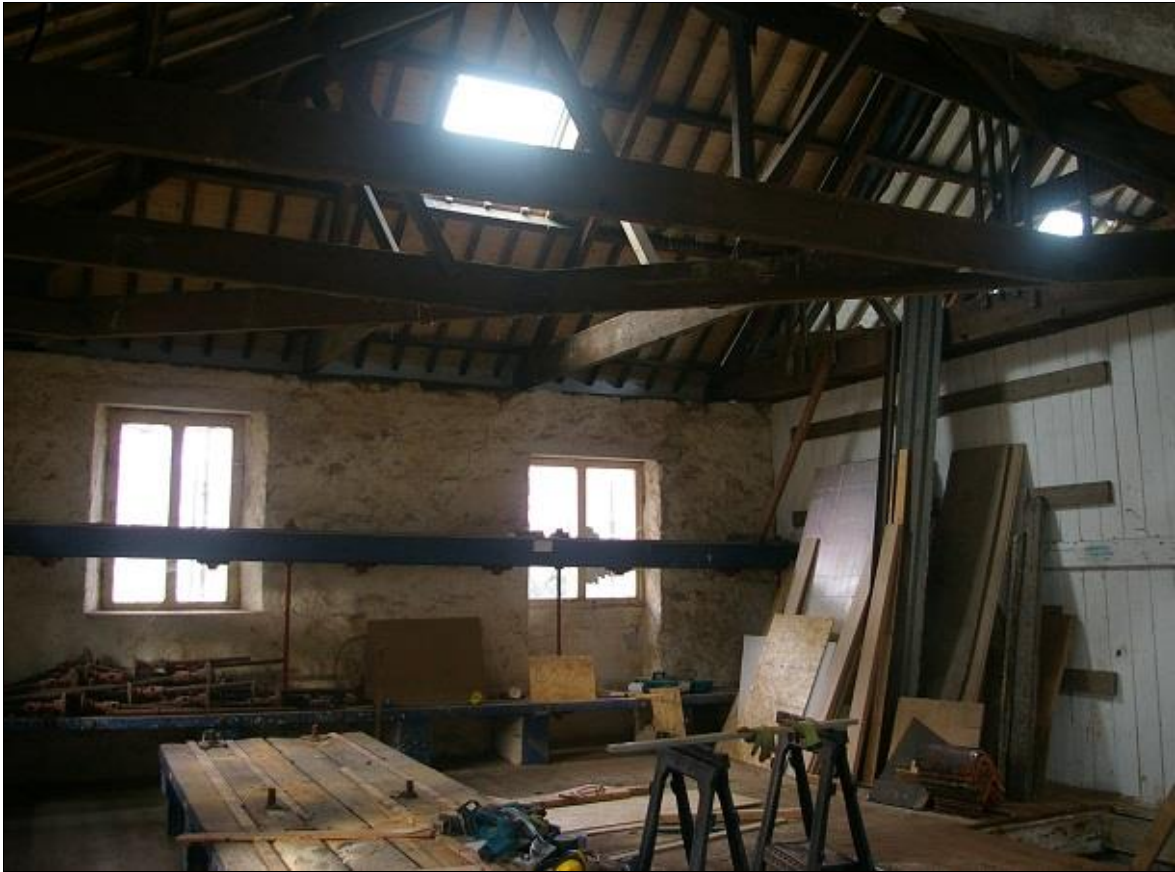
FIGURE 7: THE NORTH-WEST WALL OF THE BUILDING, WITH BLOCKED LOADING DOORS AND BOARDED PARTITION OF THE L-SHAPED RANGE, EVIDENCES THE JOINT FUNCTION AS FORMER SAIL LOFTS OR WAREHOUSES; FROM THE SOUTH.
