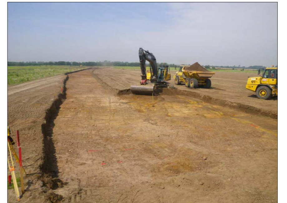
Plate 12: Working shot of Site
