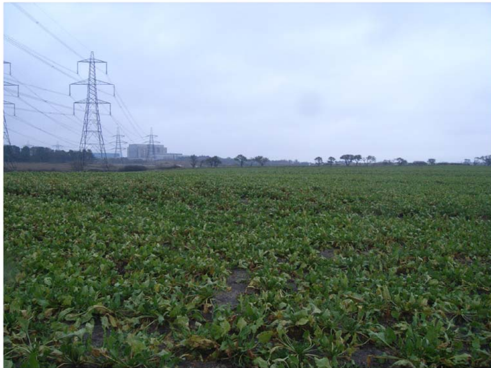
Plate 4 Location of substation 2
