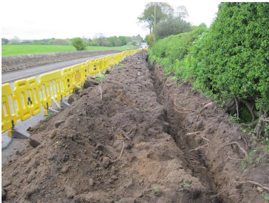
Figure 21: Post-excitation shot of Trench 3 from its western end, looking east
