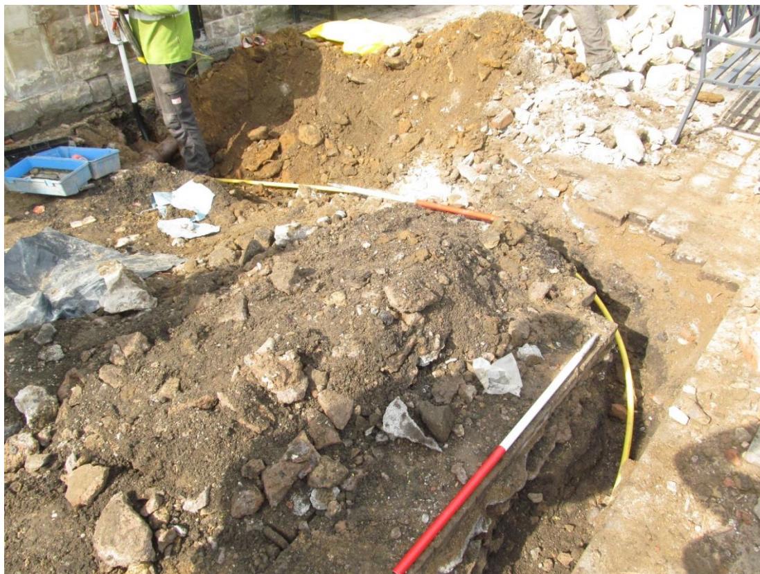
Figure 24: Overall view of new gas pipe, looking south-west. 2 x 1m scale
