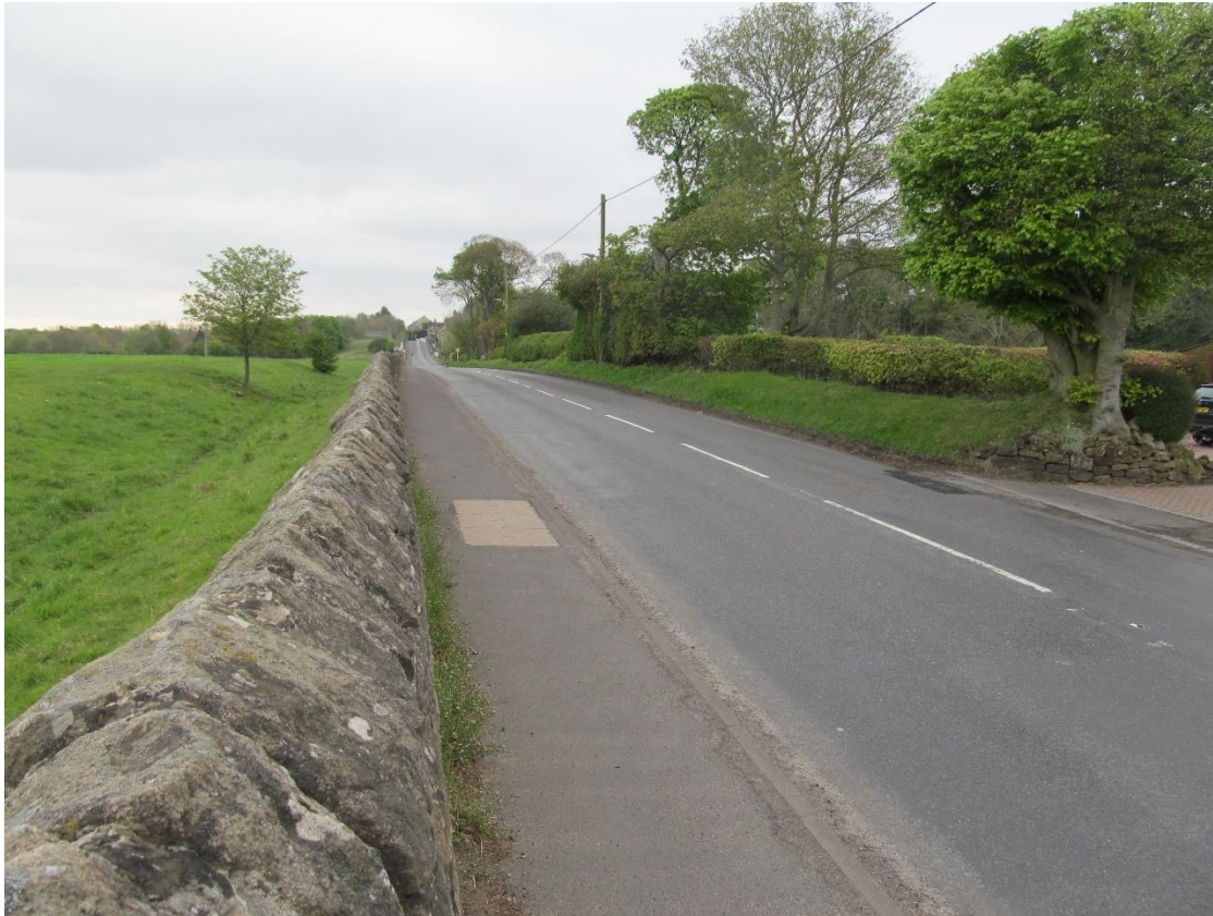
Figure 4: Pre-excavation view along Military Road from the western end of the excavation, looking east-south-east
