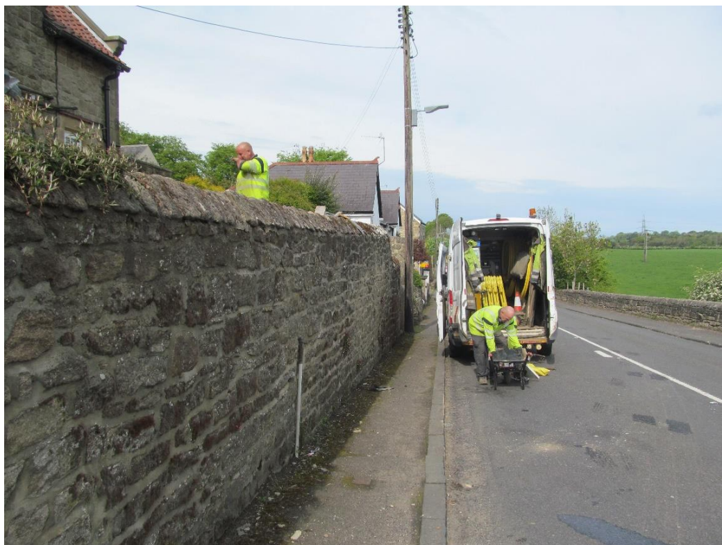
Figure 25: Differentiation in height between the garden of 11a Military Road (left of frame) and Military Road (right of frame), looking west
