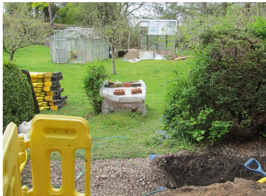
Figure 12: View over Trench 4's southern end, showing greenhouses in the centre background and the rise of the vallum bank to their left
