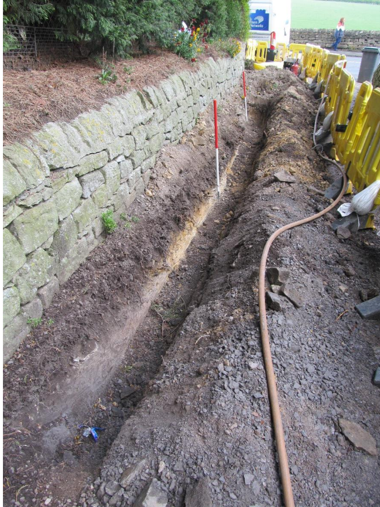
Figure 15: Trench 8, looking north. 2 x 1m scale
