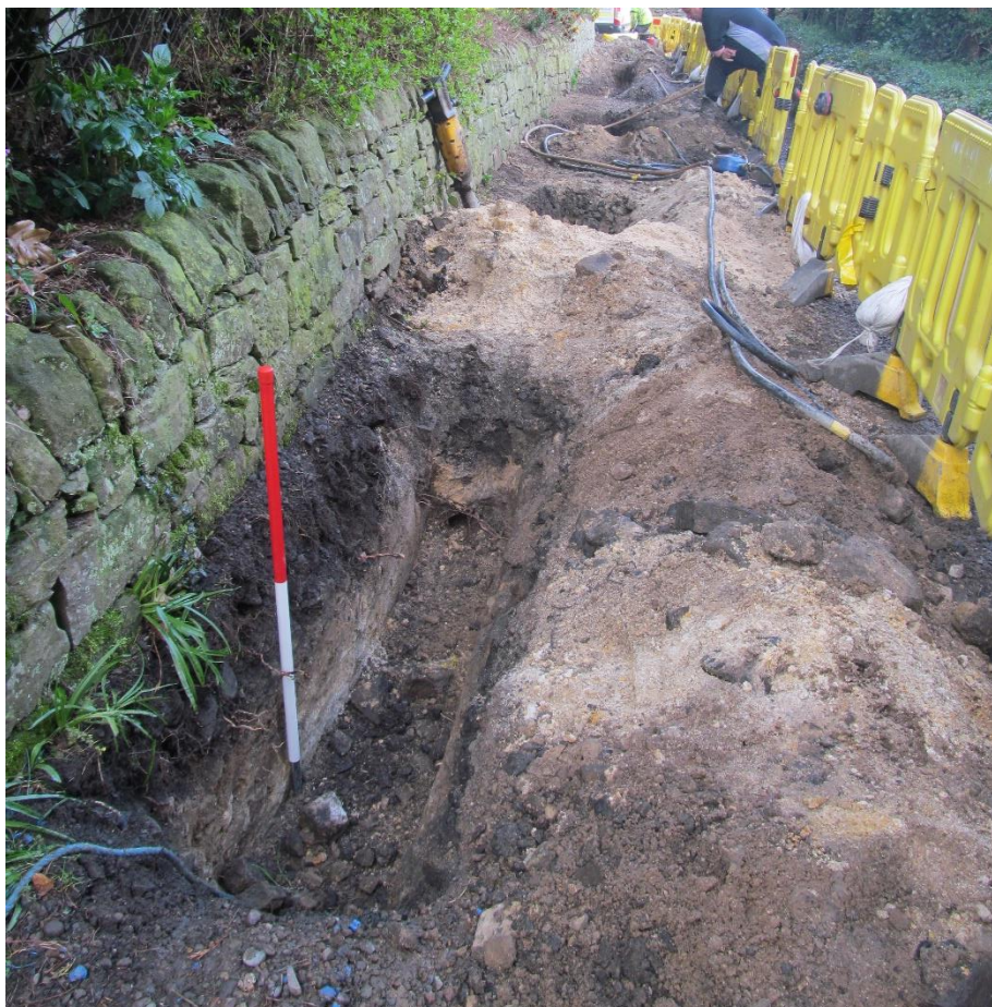
Figure 13: Trenches 5 (foreground) to 8 (background), looking north. 1 x 1m scale
