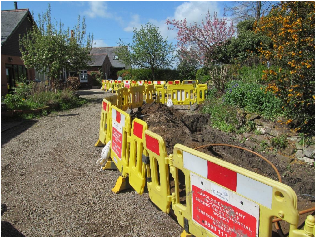
Figure 17: View of southern end of the PDA once excavated, looking south-west
