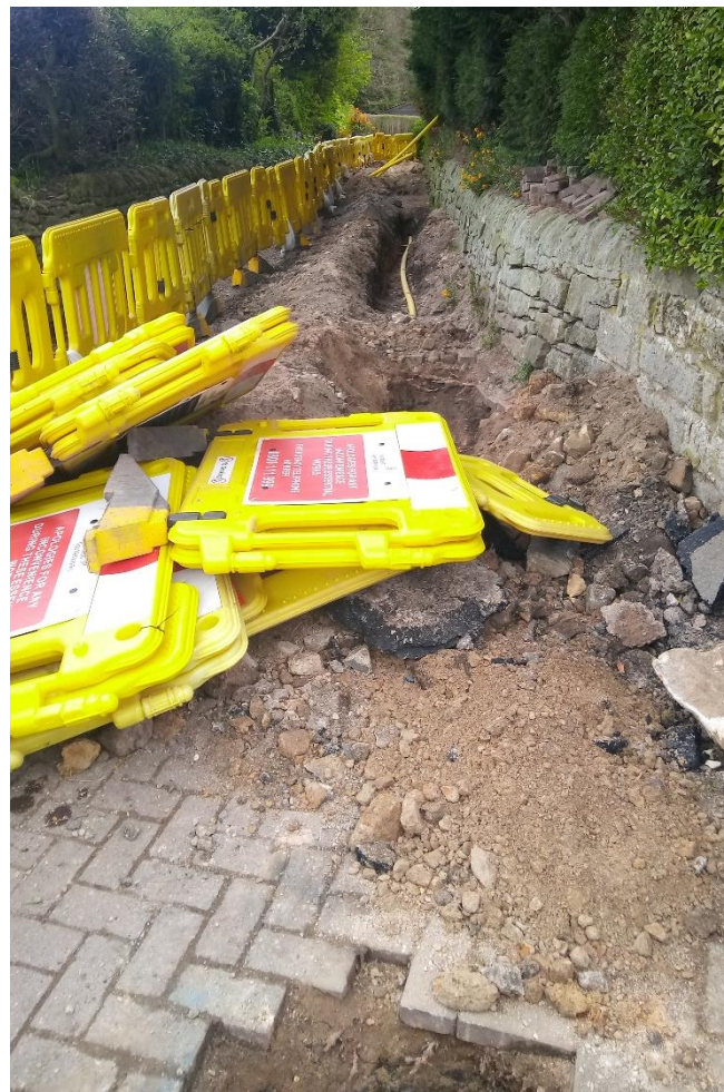
Figure 18: View of northern end of the PDA once excavated, looking south
