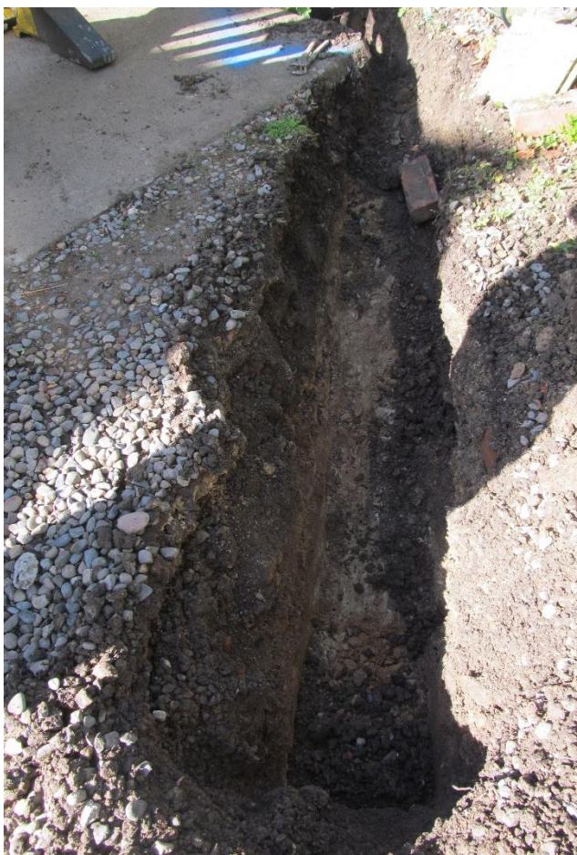
Figure 5: Trench 1, looking south-west. Unscaled.
