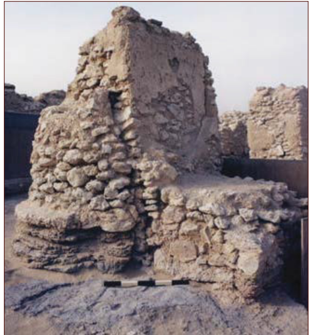
[41] The south-east wall of the temple. The Phase 3 rebuilding is visible in the SE wall of the temple: the Phase 1/2 wall can most clearly be seen to the west (left side) of the altar, at the bottom. It is separated from the Phase 3 wall in this area by a packing of hard mortar used as foundation material. At both the west and east end, the original south wall was retained in the rebuild. Both the Phase 1/2 altar and the Phase 3 southern altar are shown, separated by our modern plasterwork which underpins the latter.
