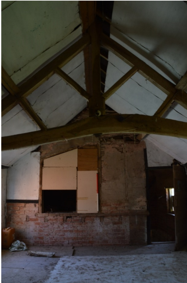
Plate 21: First floor, Barn A. Vernacular king post truss with inserted room or storage space in background
