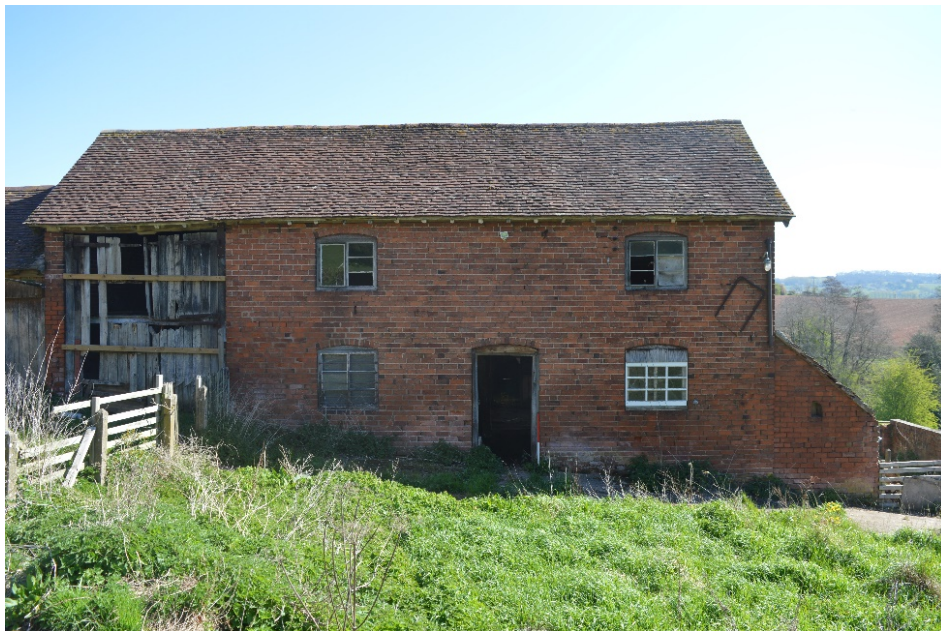
Plate 5: Western elevation of Barn A (1m scale)
