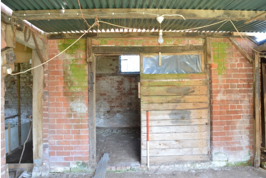
Plate 12: Lean-to at rear from south
