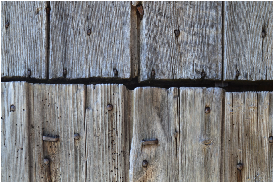
Plate 20: Iron nails on stable door in Barn B
