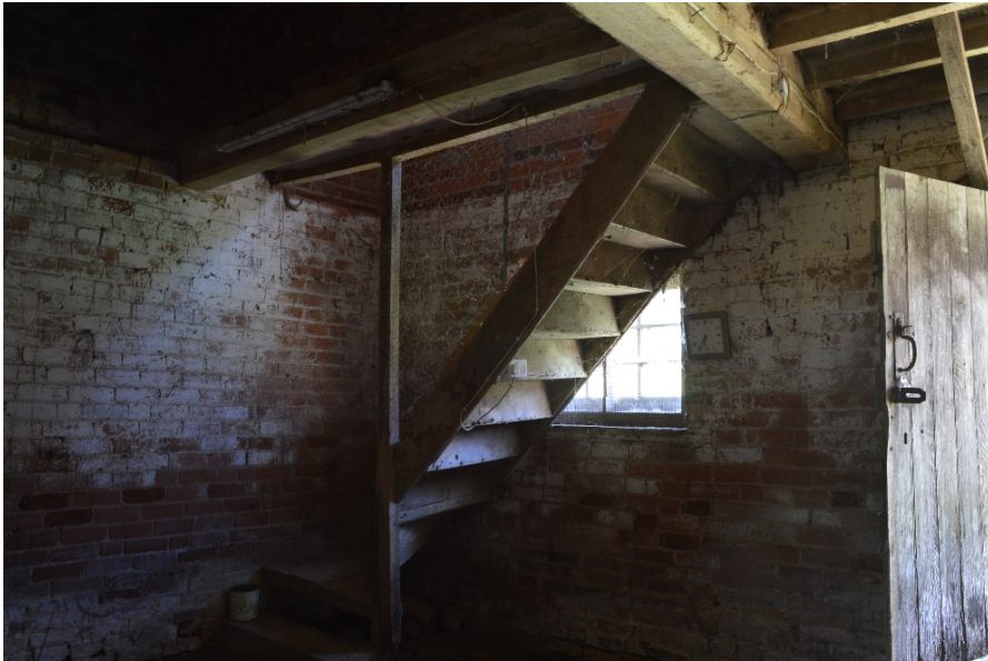
Plate 10: Wooden stairway in south-west corner Barn A
