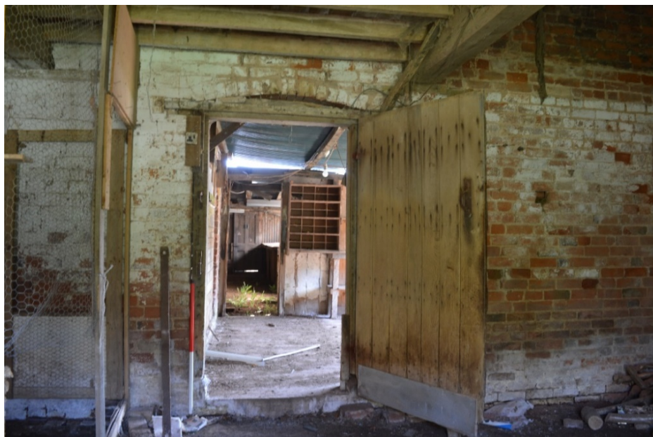
Plate 9: Rear door in Barn A
