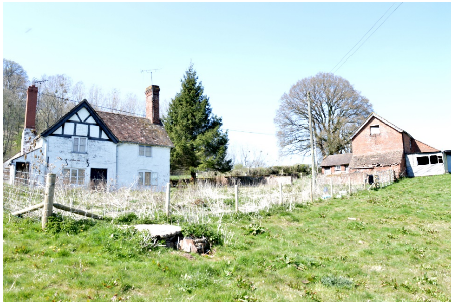
Plate 3: Furnace Farmhouse and barns from south-east
