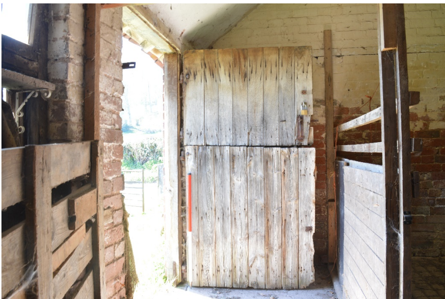
Plate 19: Stable door in Barn B
