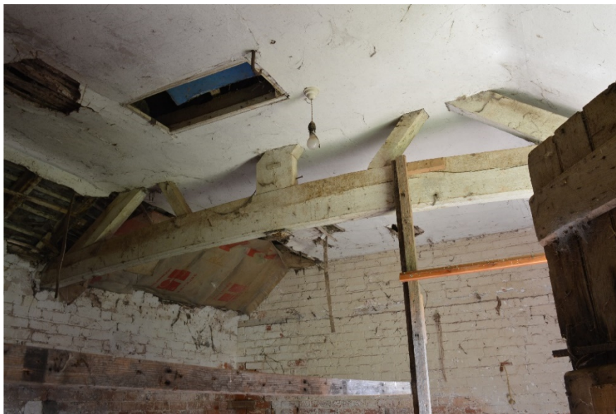
Plate 17: King post truss partially obscured by an inserted ceiling, Barn B
