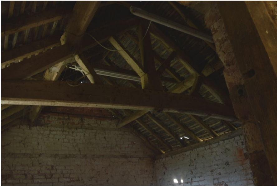
Plate 18: King post truss in the western shed in Barn B
