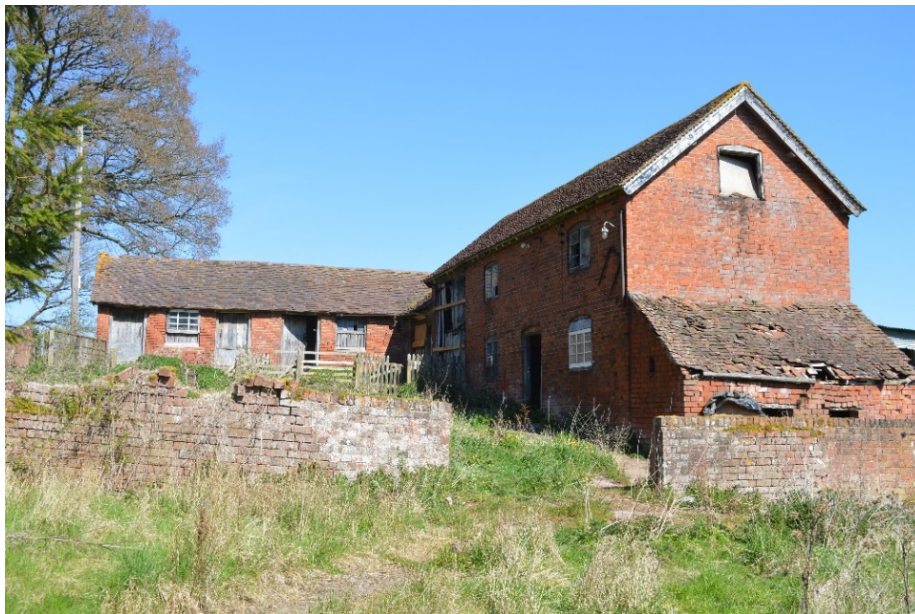
Plate 7: South-south-east facing elevation of Barn B
