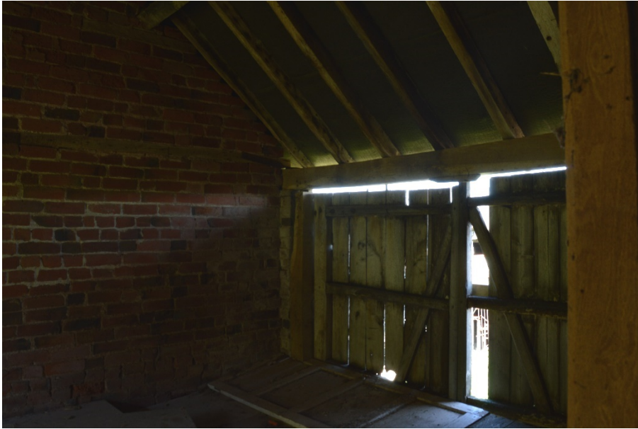
Plate 23: Inserted floor in threshing barn, Barn A.
