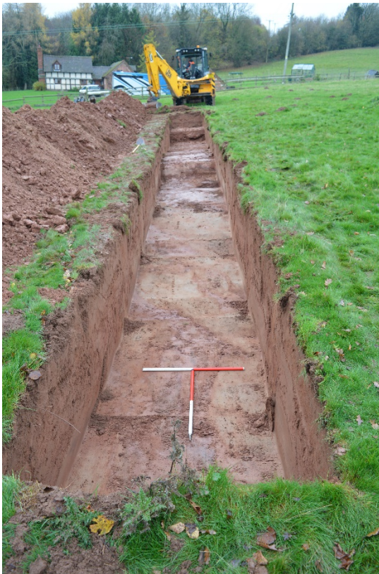
Plate 4 – Trench fully excavated, from north
