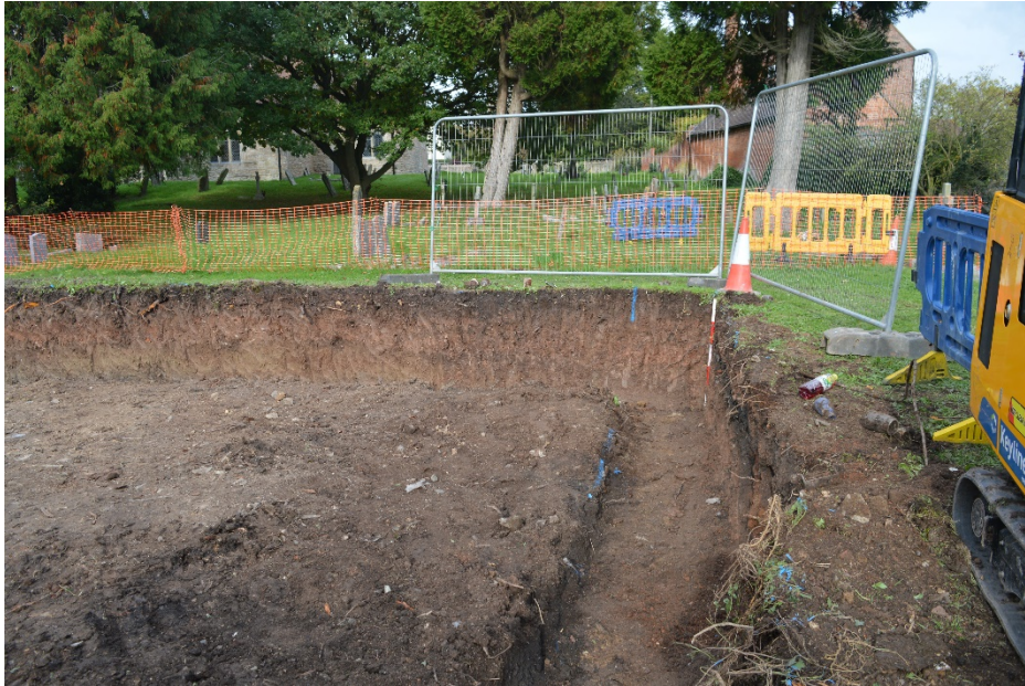
Plate 7 Site fully excavated from south
