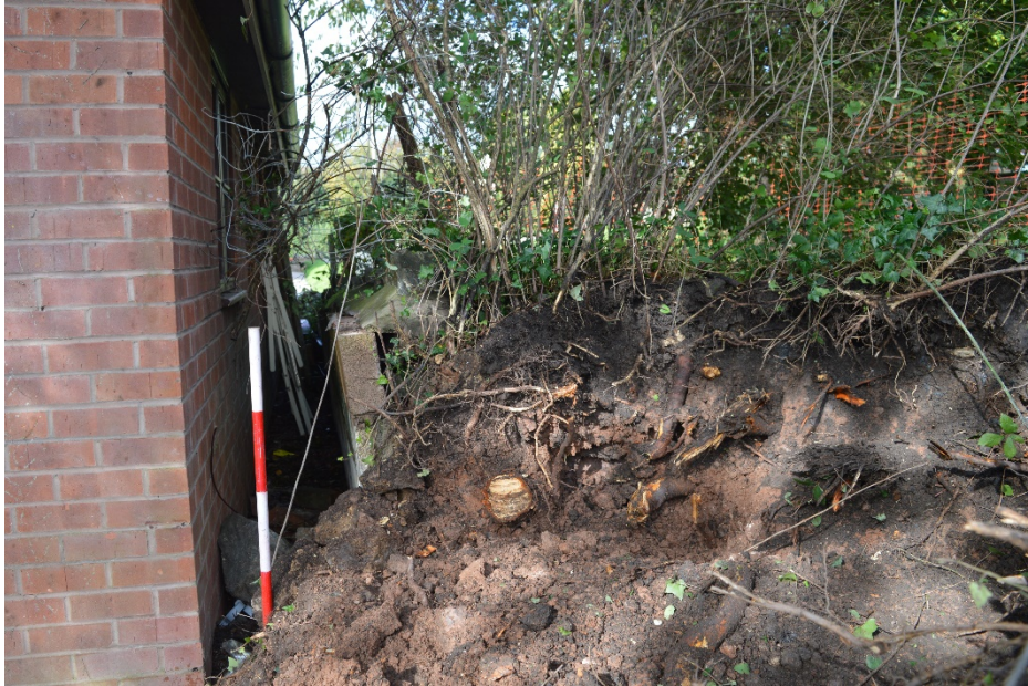
Plate 3 Western extent of demolition and excavation, by modern garden shed
