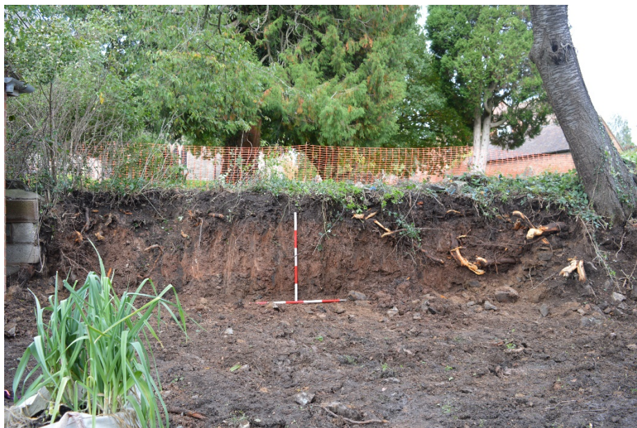
Plate 4 South-west facing section following removal of revetment wall
