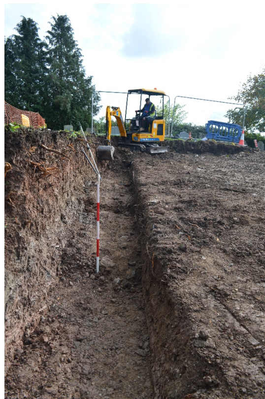
Plate 6 foundation trench for replacement wall, from north-west
