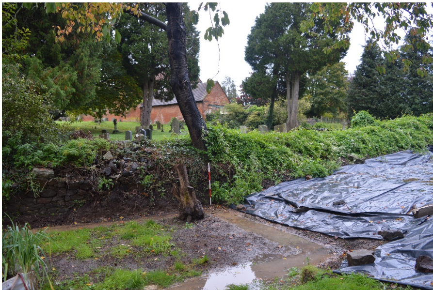
Plate 2 Wall before excavation, from south-west
