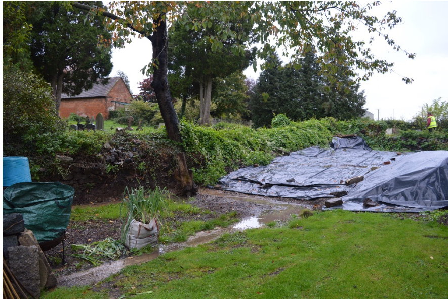
Plate 1 Site before excavation, from south-west
