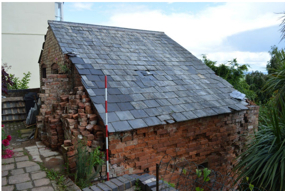
Plate 14: Oblique view north-east of south elevation
