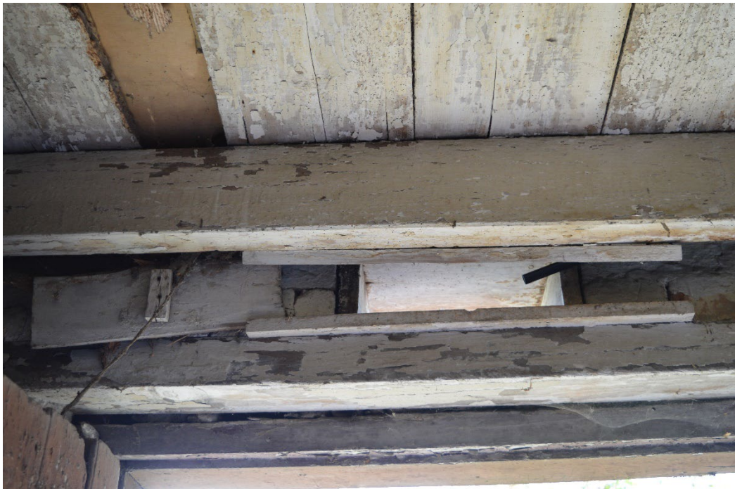
Plate 18: Possible ventilation hatch over door in stable
