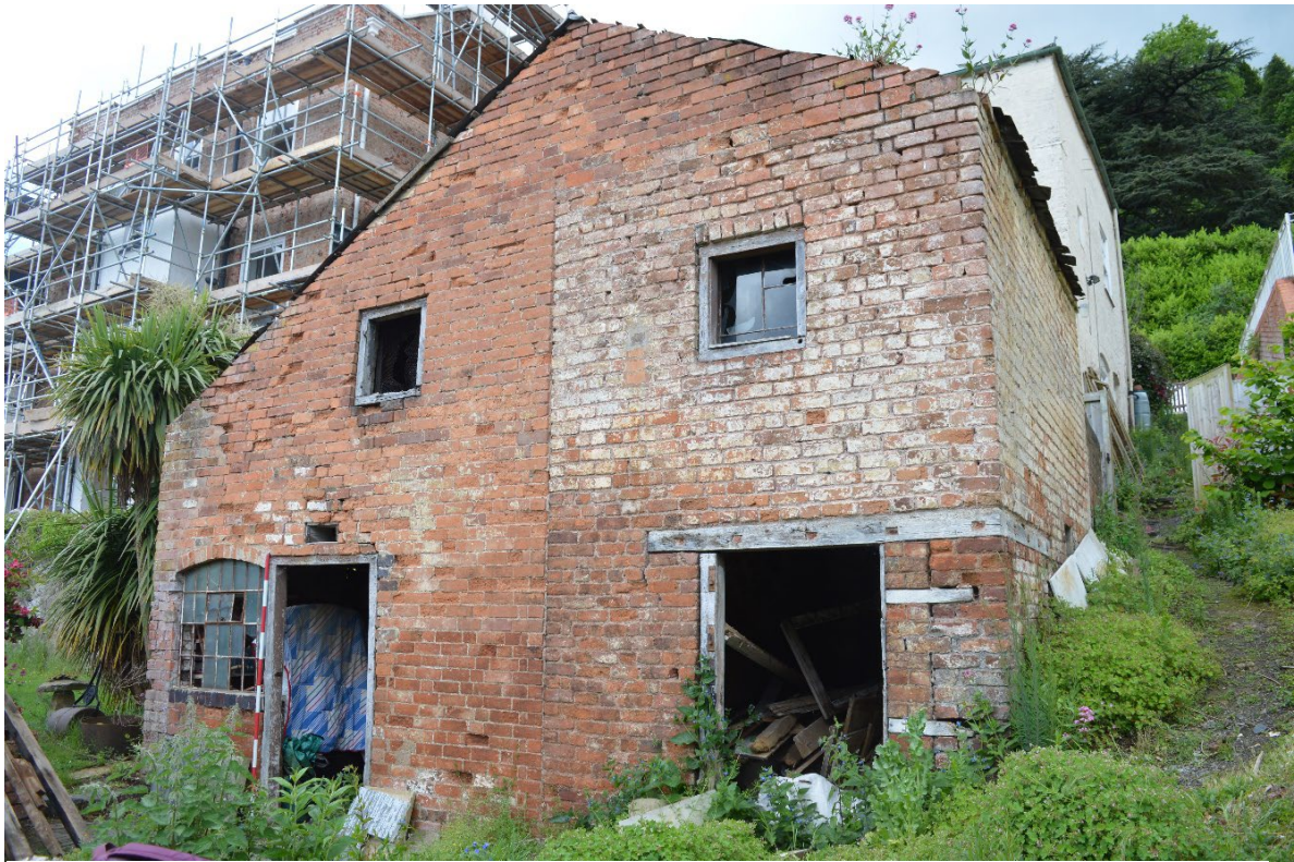
Plate 3: Oblique view south-west of recorded building
