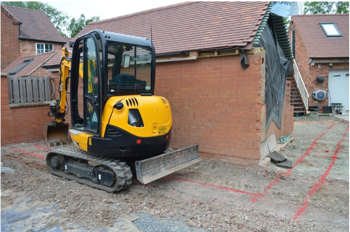
Plate 2. Trench 1 prior to excavation, view north
