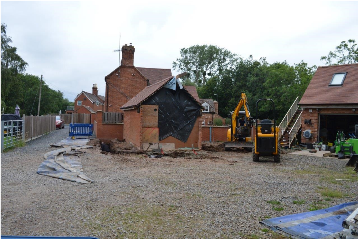
Plate 1. The site from the south-west
