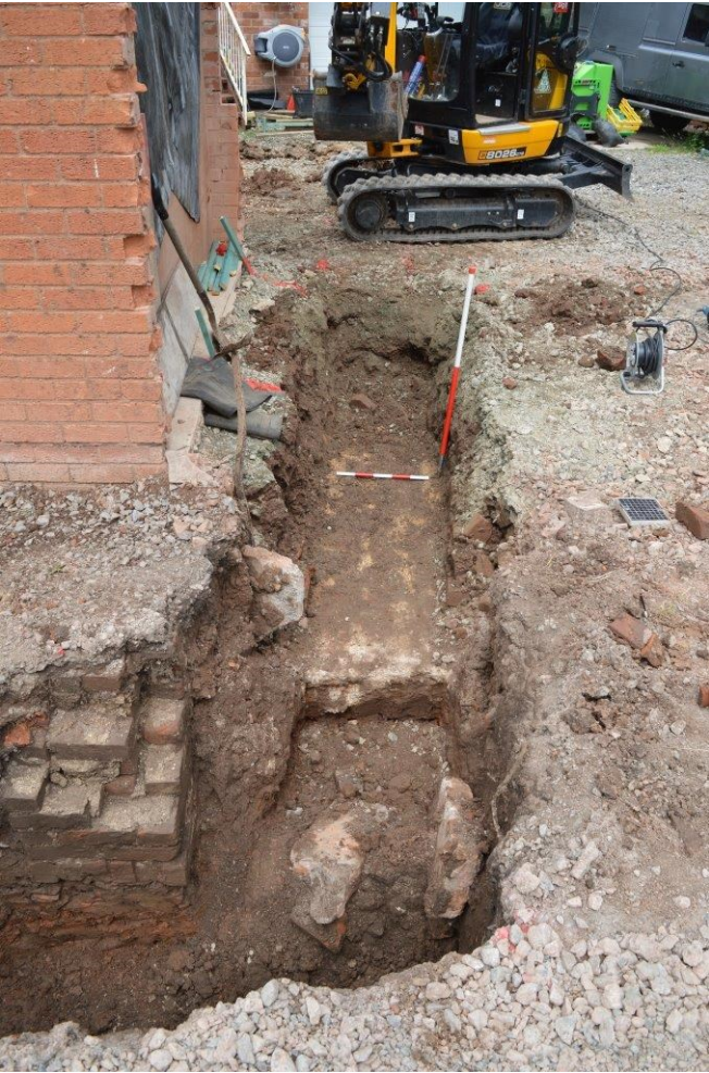
Plate 7. South-eastern section of Trench 1, view north-east, scales 1m and 0.5m
